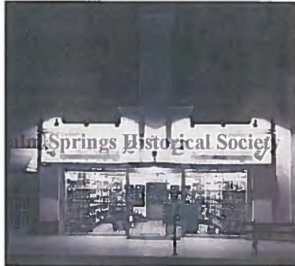
C. 1950's: CENTER PILASTERS REMOVED & DISPLAY WINDOWS ENLARGED DOWN TO THE FLOOR. NOTE THE "ANNEX" AT THE LEFT (344 NORTH PALM CANYON DRIVE)
