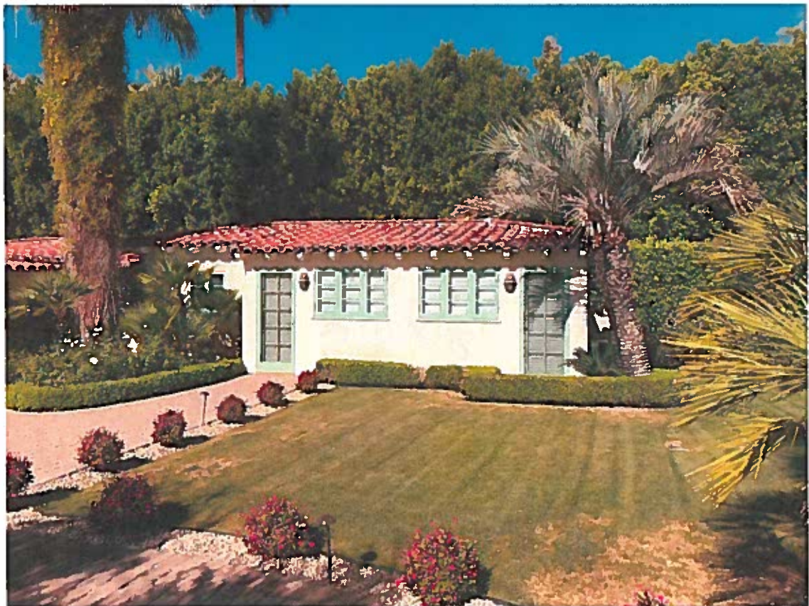
The Roosevelt guest cottage today, door and window configuration altered with additional square footage added to front.
