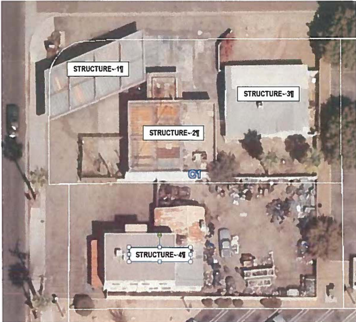
AERIAL PHOTO SHOWING THE TWO LOTS AND THE FOUR STRUCTURES.
