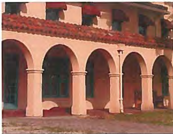
ABOVE LEFT, TYPICAL ARCHED COLONADE
