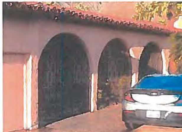
ABOVE RIGHT, ARCHED COLONADE AT 561 CAMINO NORTE
