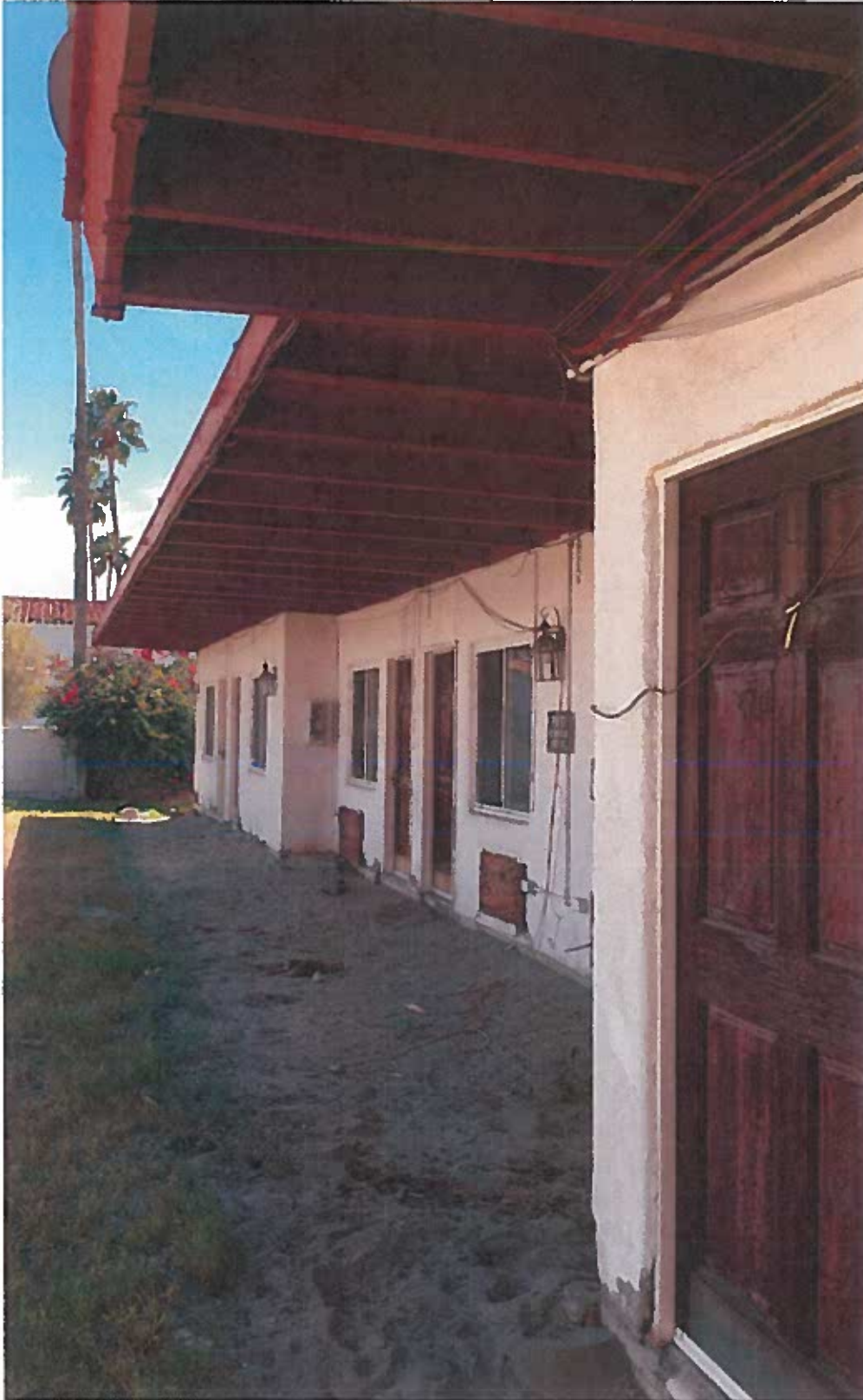
Photo 4: Crawford Apartments: Building "B" looking south along east façade.
