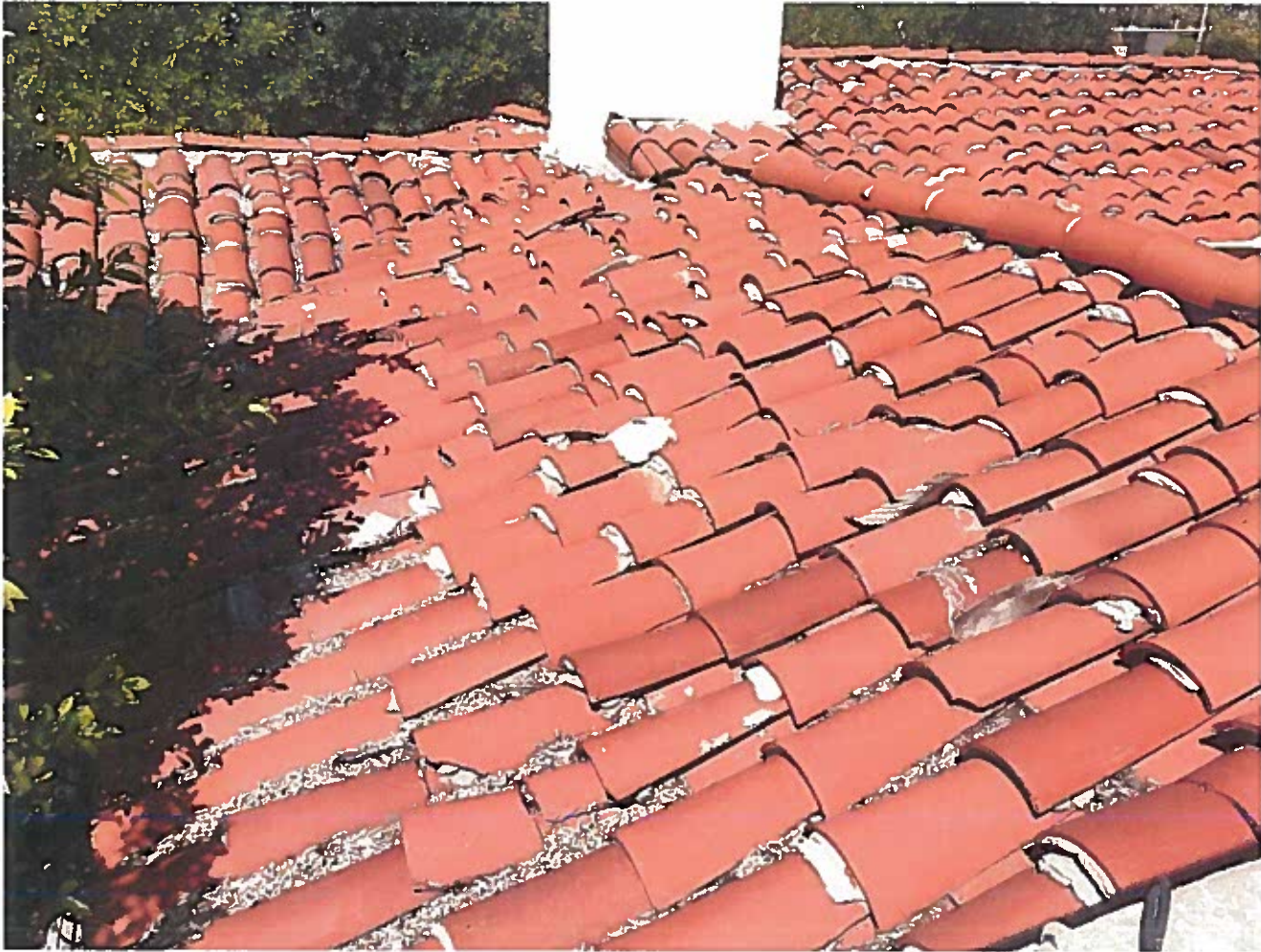
Photo 25 Harlow Haven Roof of Bldg C
