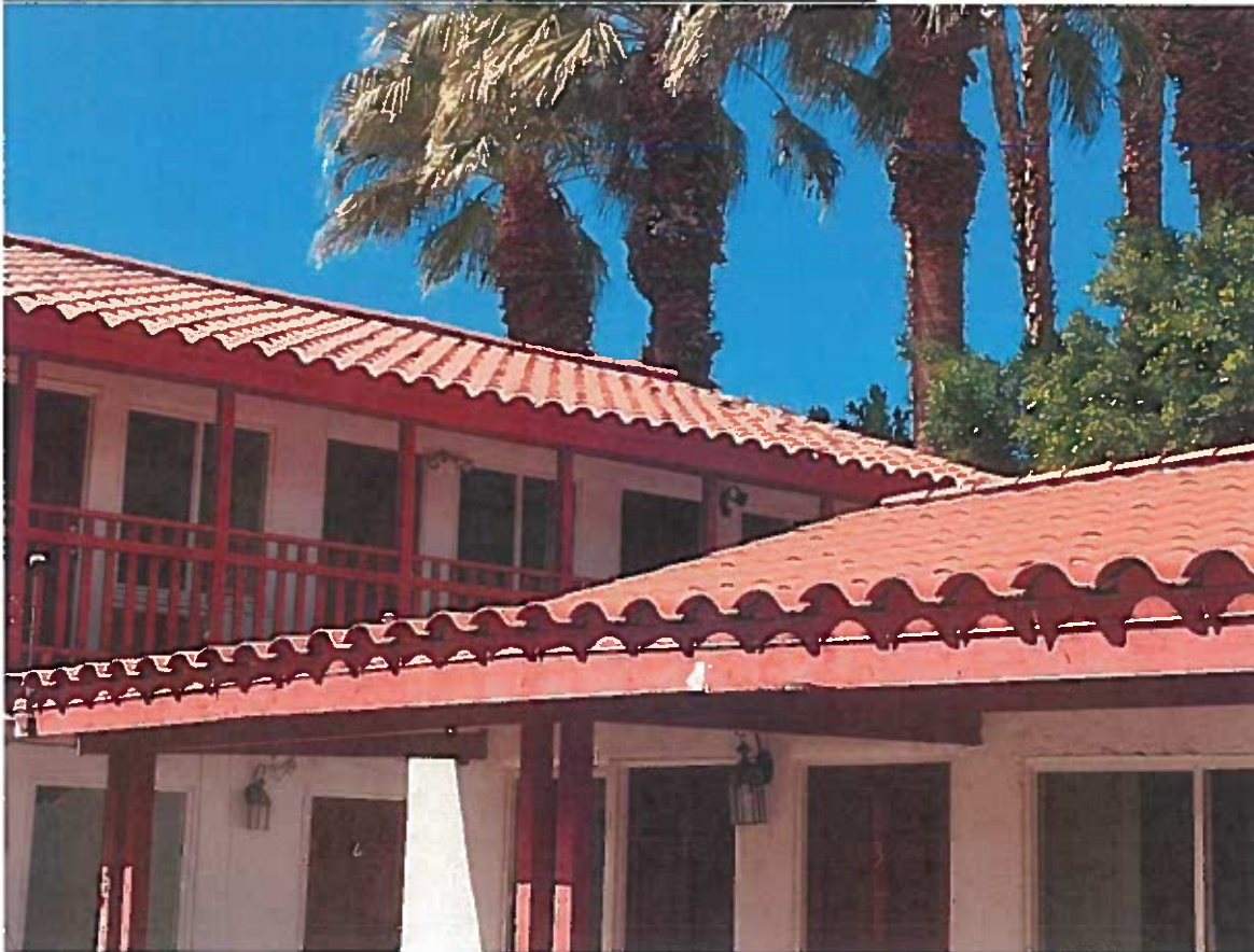
Photo 2: Crawford Apartments partial view of upper story
