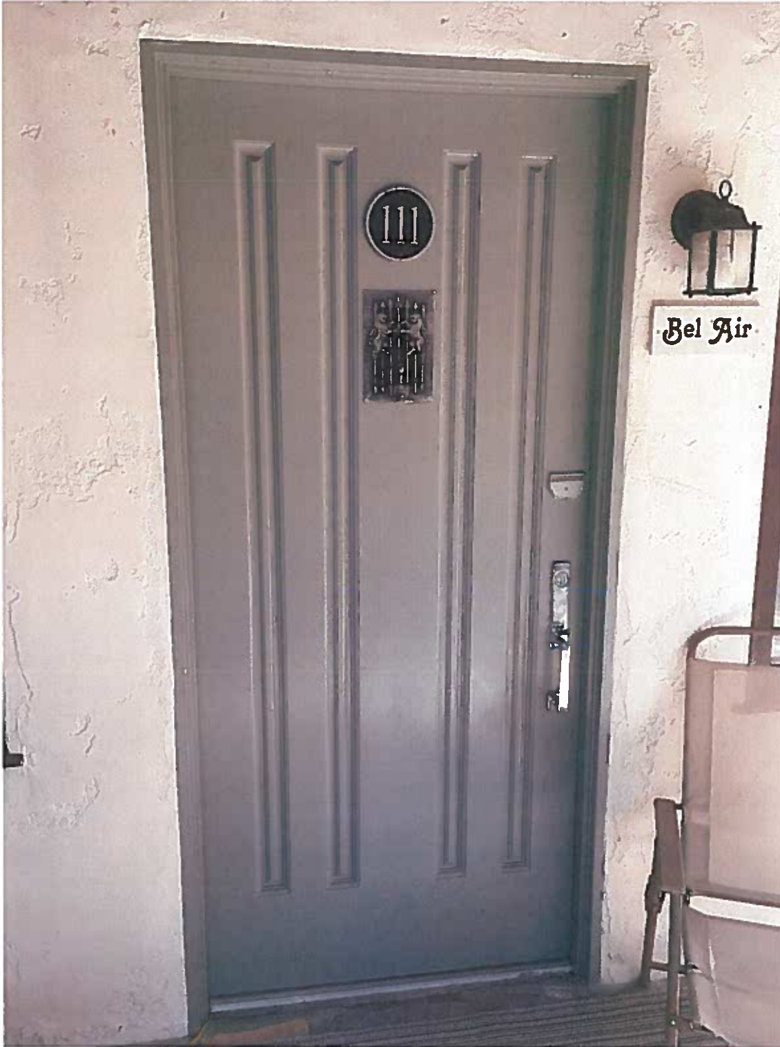
Photo 44 Harlow Haven Bldg D typical front door.
