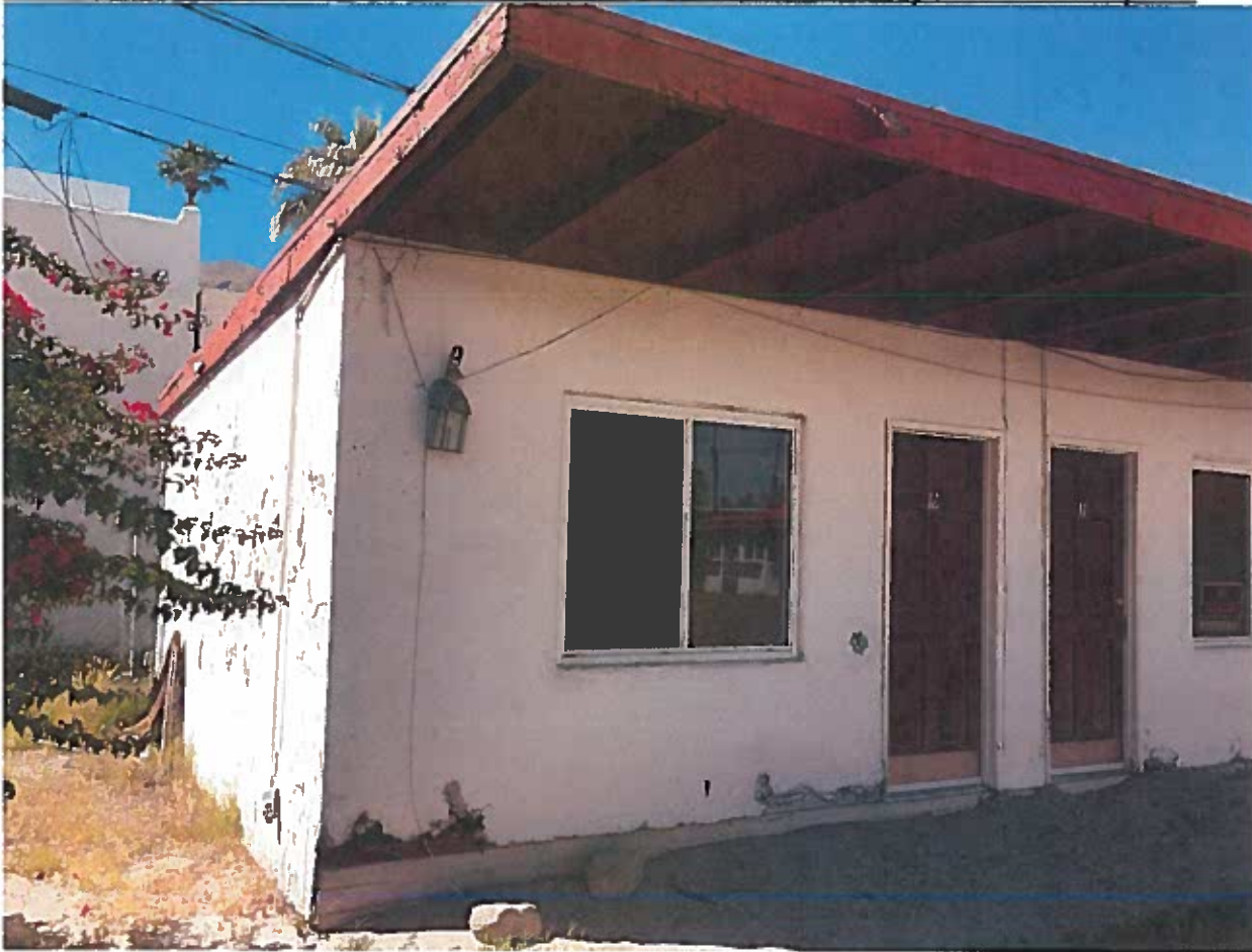
Photo 10: Crawford Apartments: Building "B" Corner of east façade / south façade.
