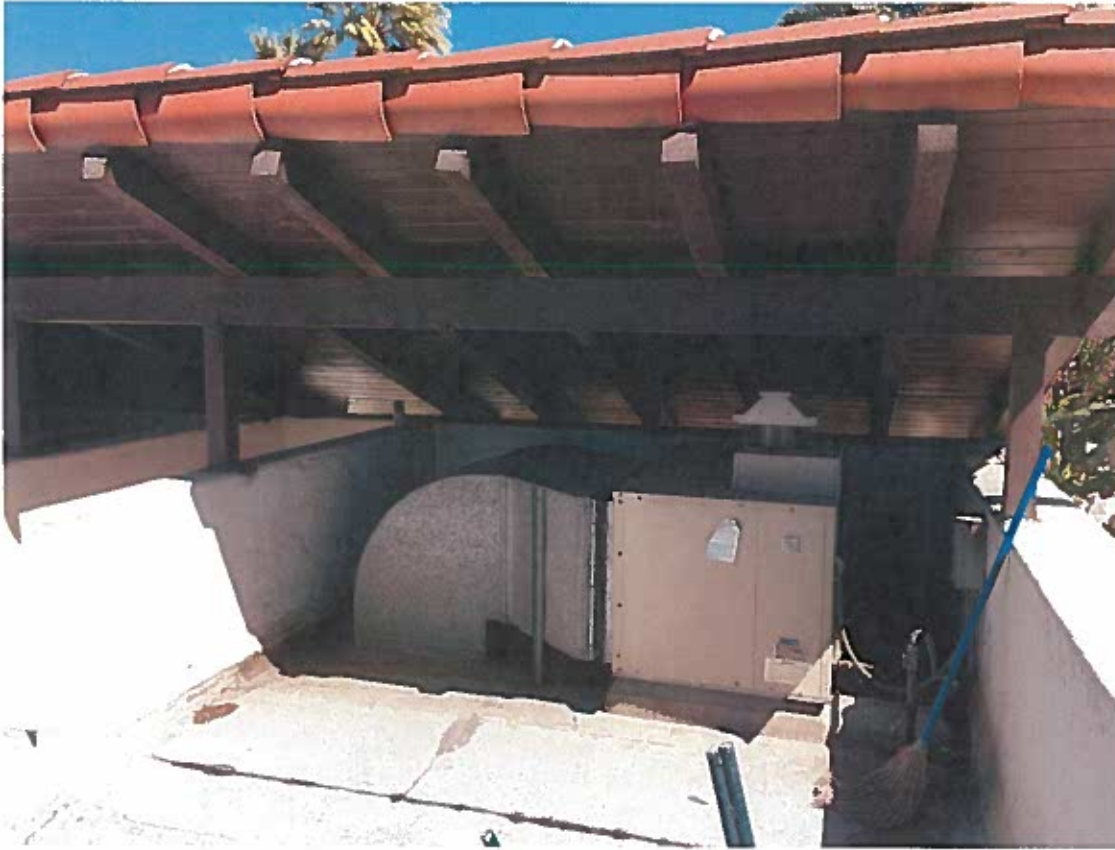
Photo 26 Harlow Haven Building C Roof
