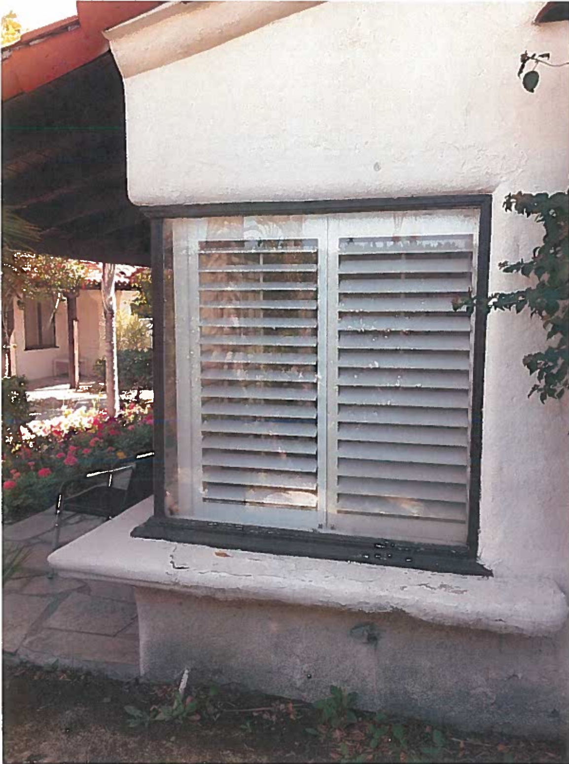
Photo 14 Harlow Haven Bldg C corner window
