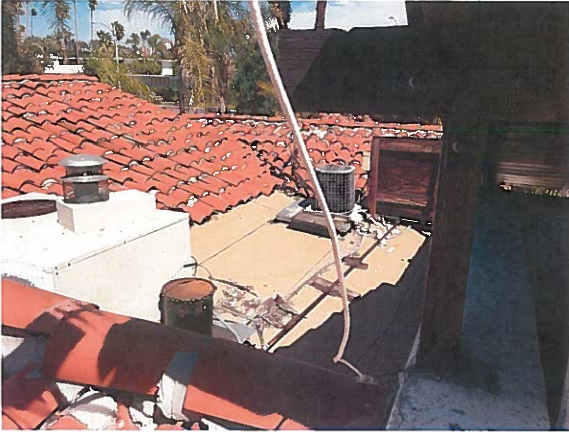
Photo 24 - Harlow Haven Roof of Bldg C
