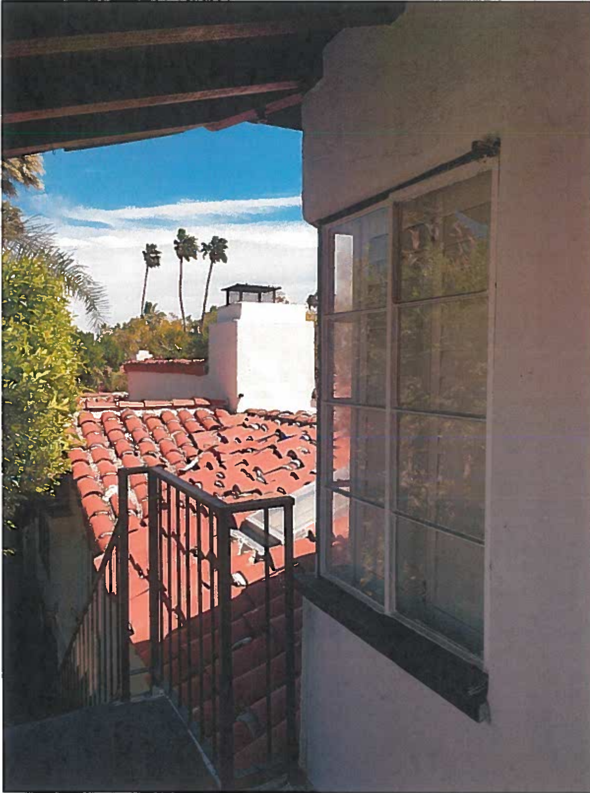
Photo 16 Harlow Haven Roof of Bldg C looking east
