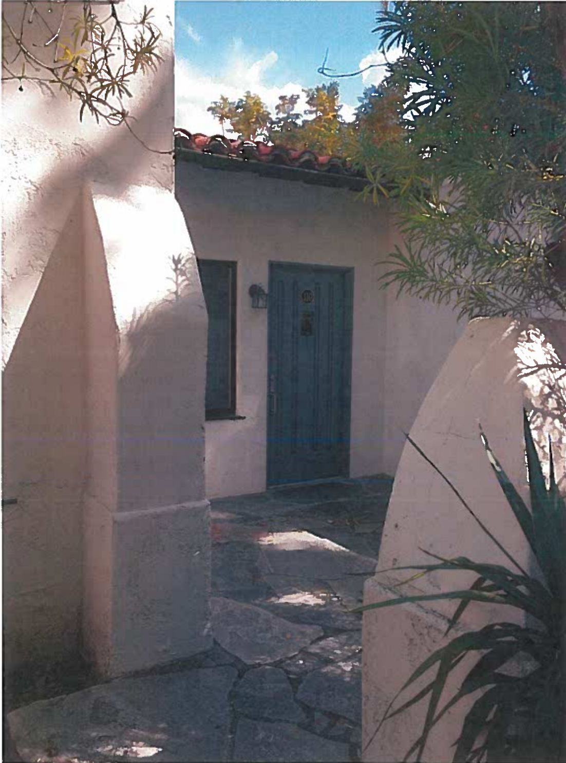
Photo 42 Harlow Haven Bldg D typical patio courtyard and patio walls.
