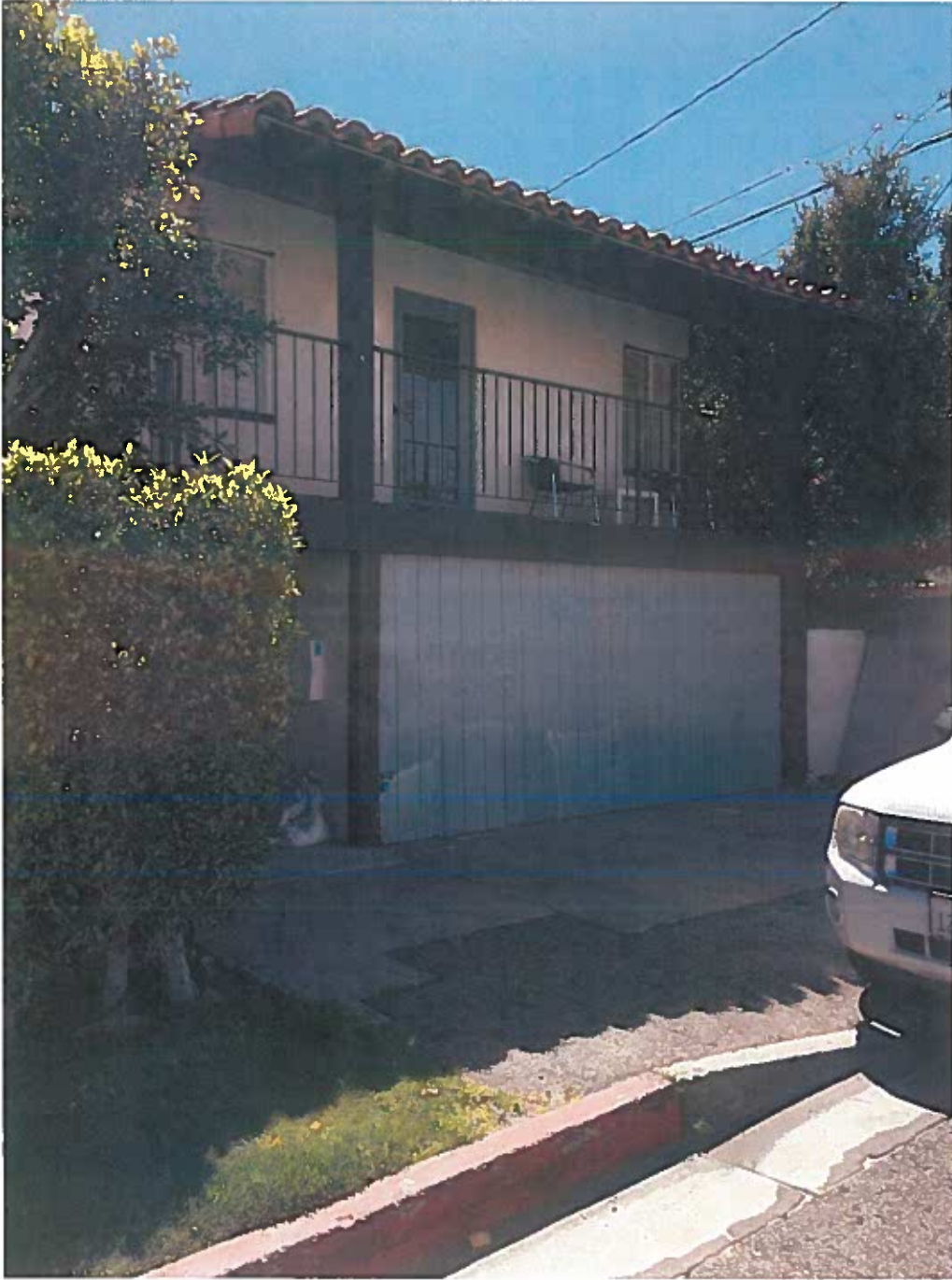
Photo 12 Harlow Haven Bldg "C" North elevation
