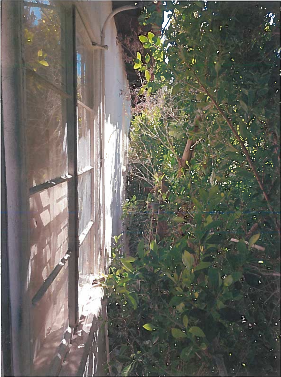
Photo 17 Harlow Haven Bldg C West elevation existing windows.
