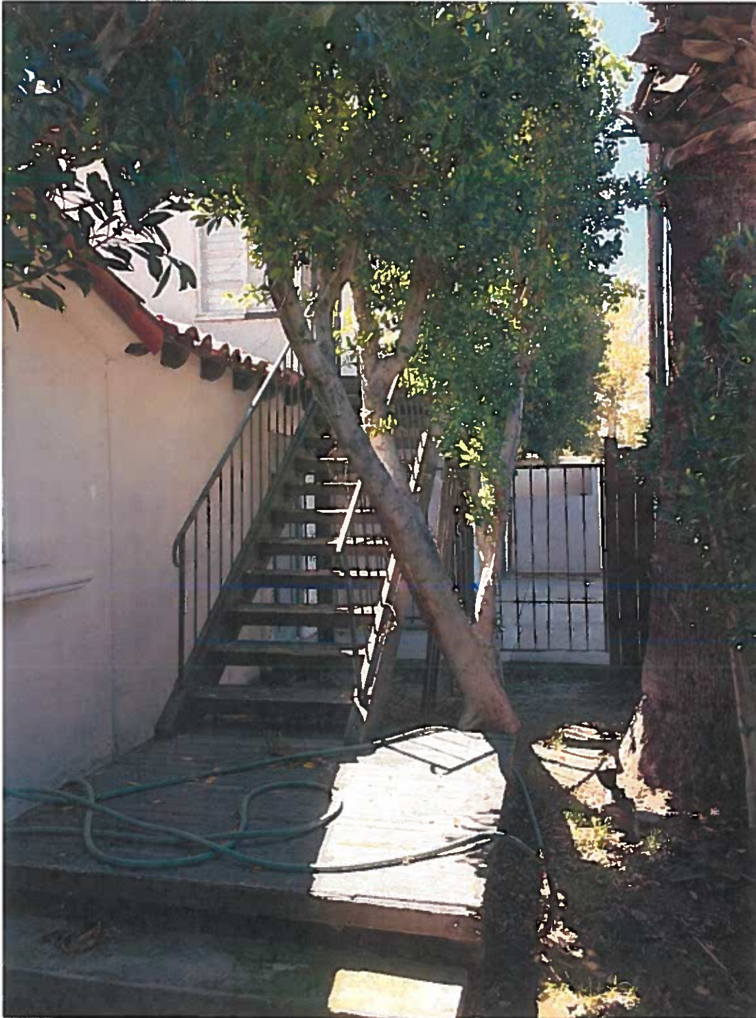
Photo 21 Harlow Haven North side Bldg C stair to second floor balcony
