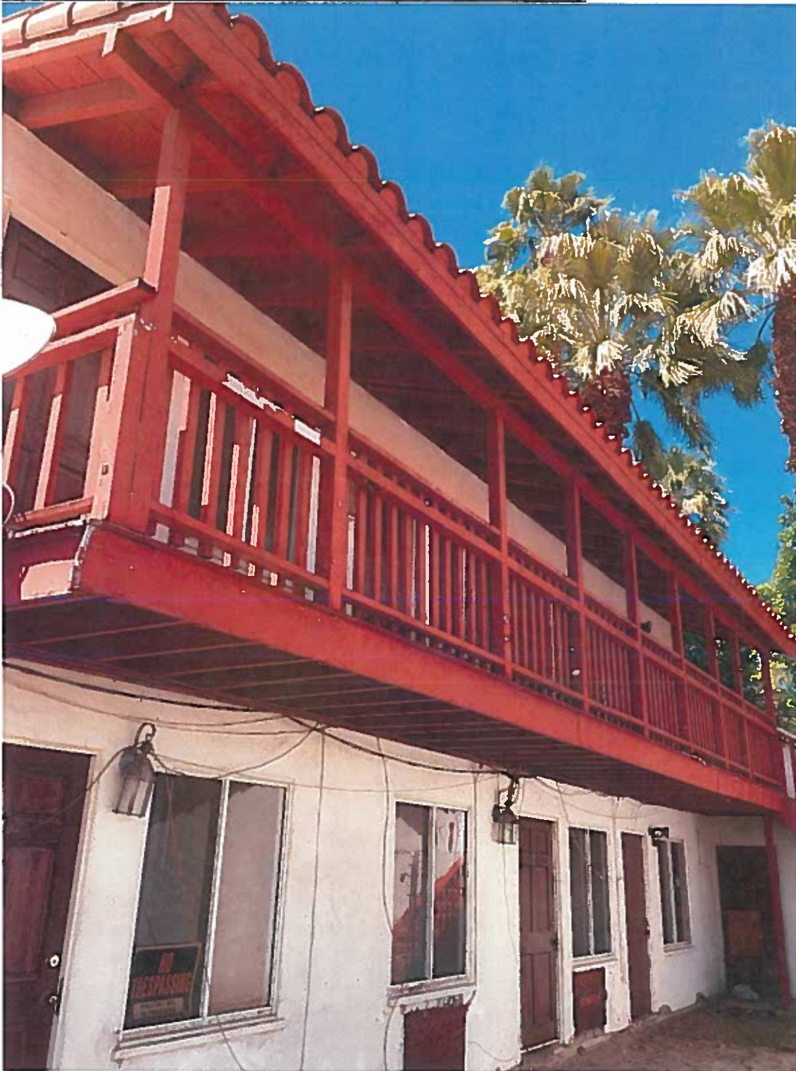
Photo 6: Crawford Apartments: Building "B" upper balcony
