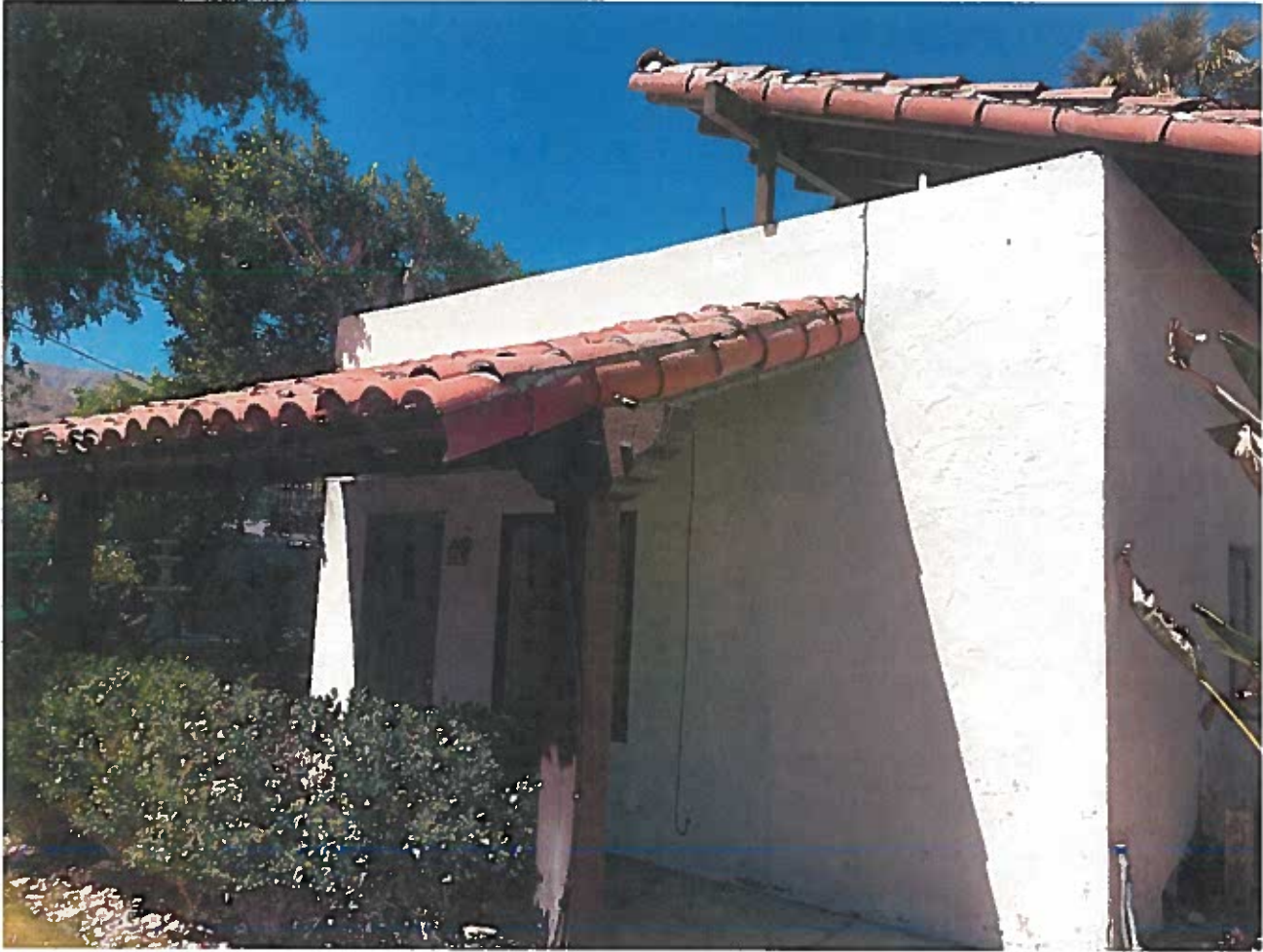
Photo 47 Harlow Haven Bldg C south elevation
