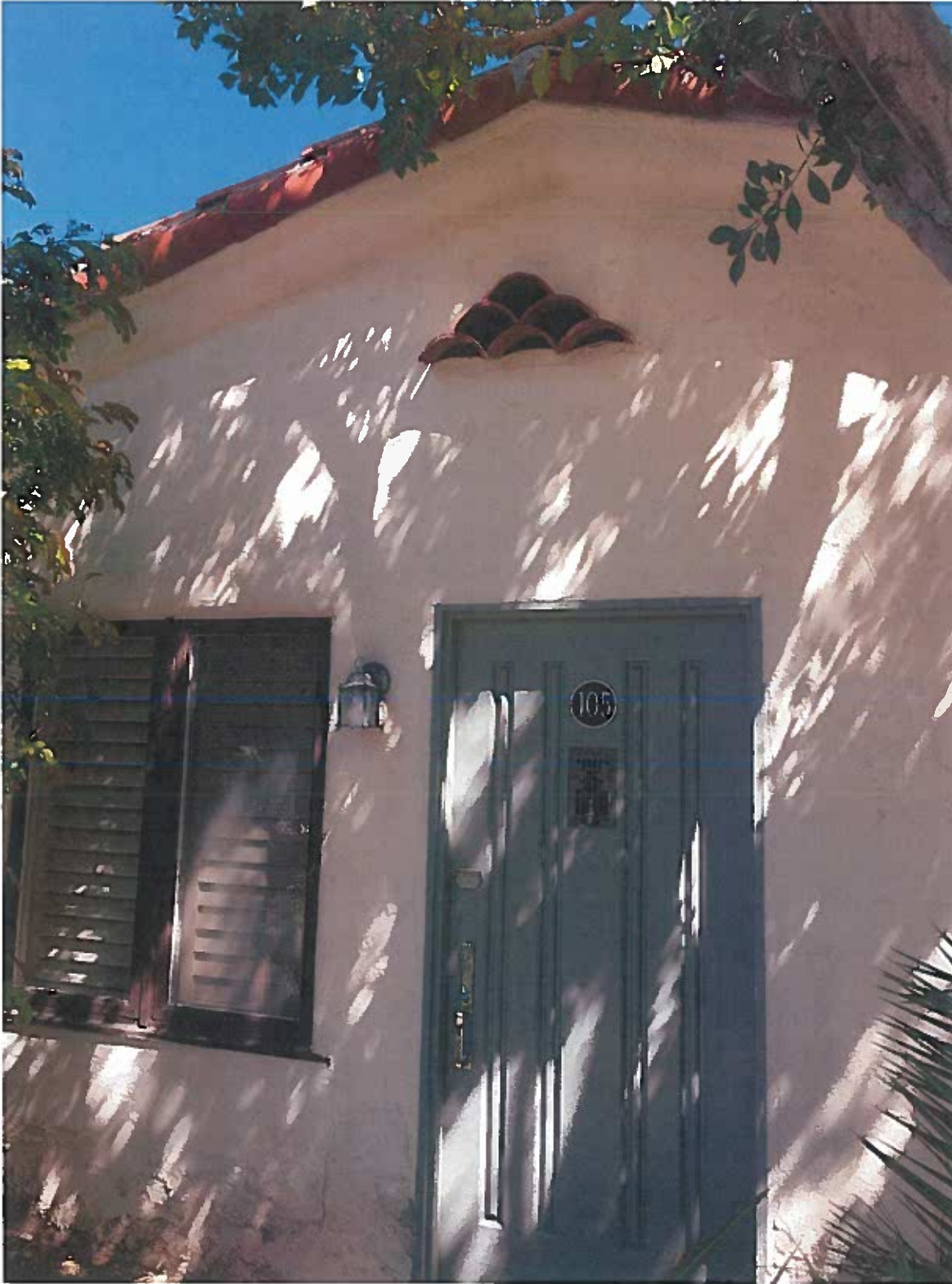
Photo 40 Harlow Haven Bldg D gable grill detail west elevation
