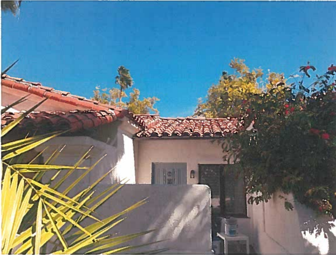
Photo 23 Harlow Haven Bldg D west elevation typical courtyard
