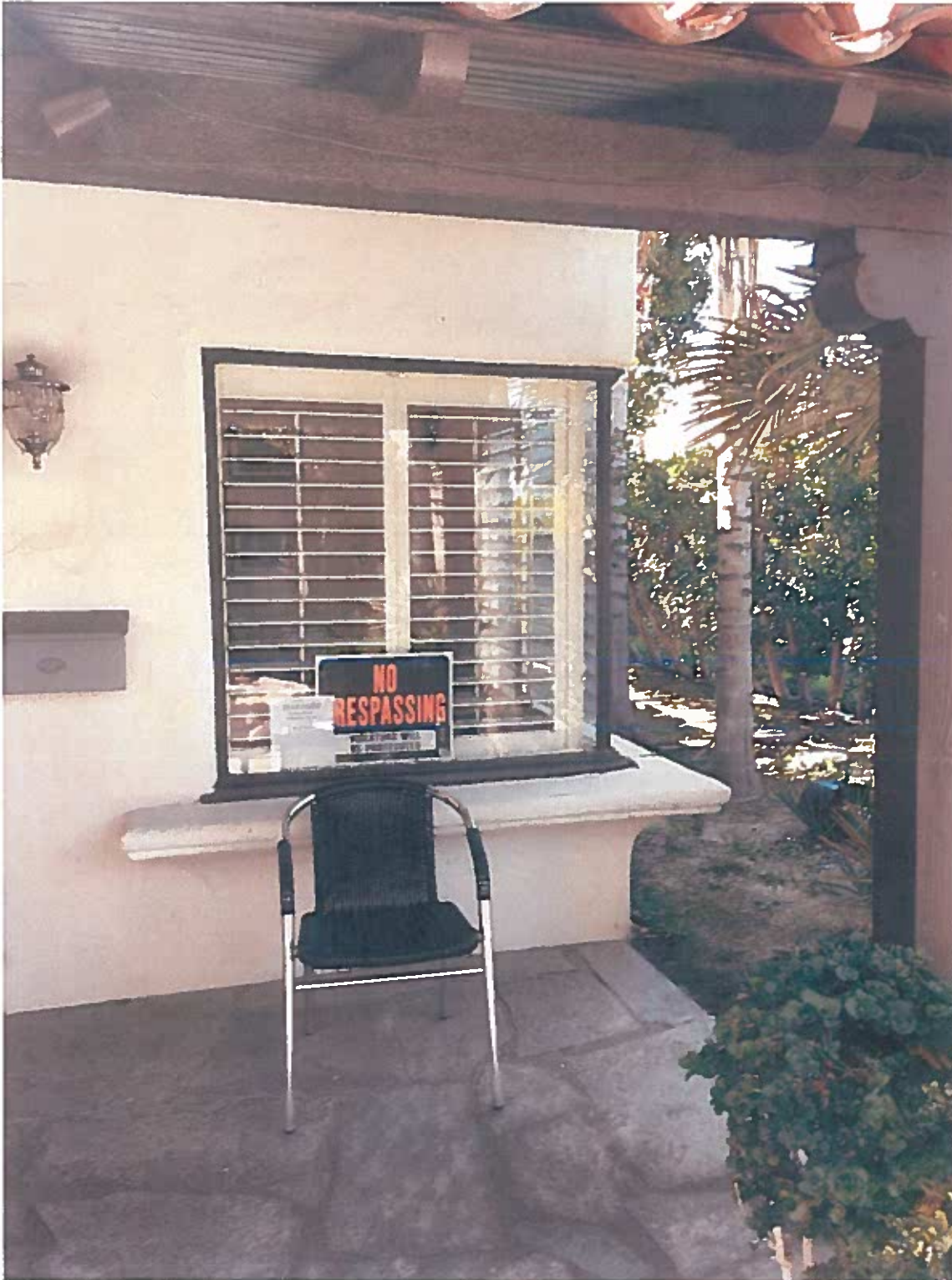
Photo 22 Harlow Haven Bldg C northeast corner window.
