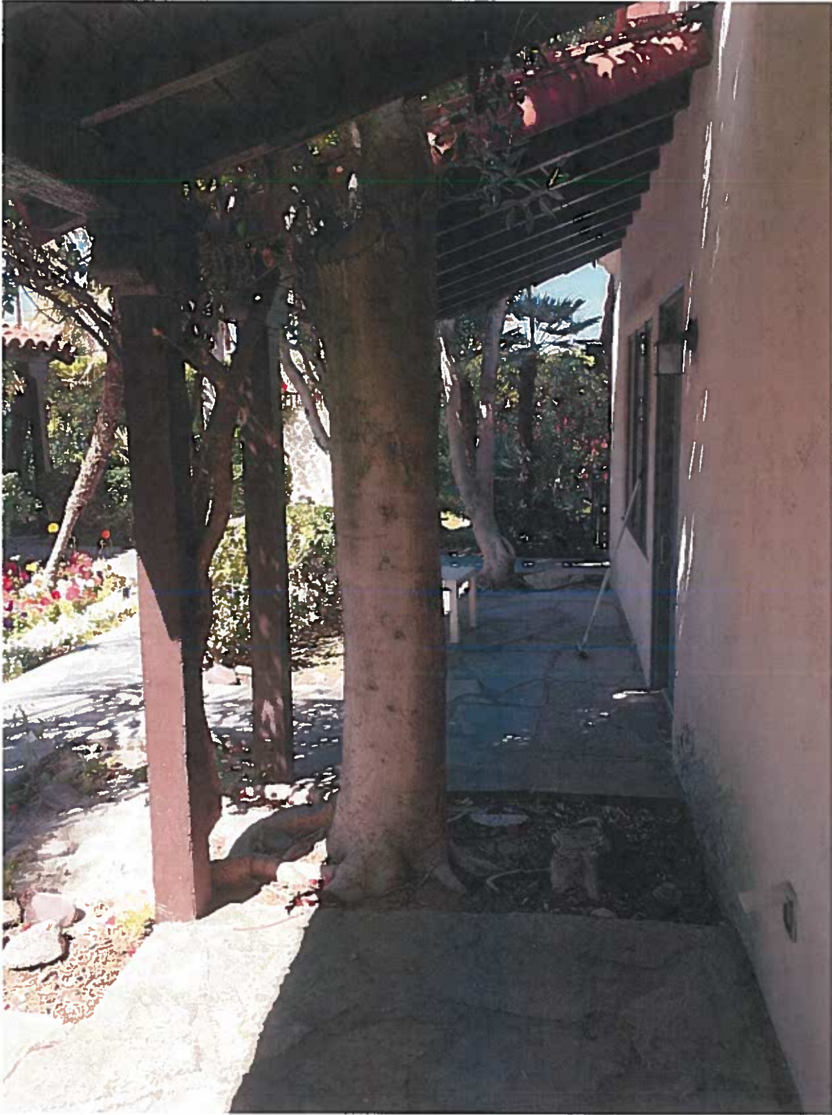
Photo 38 Harlow Haven Bldg D west elevation typical covered front porches
