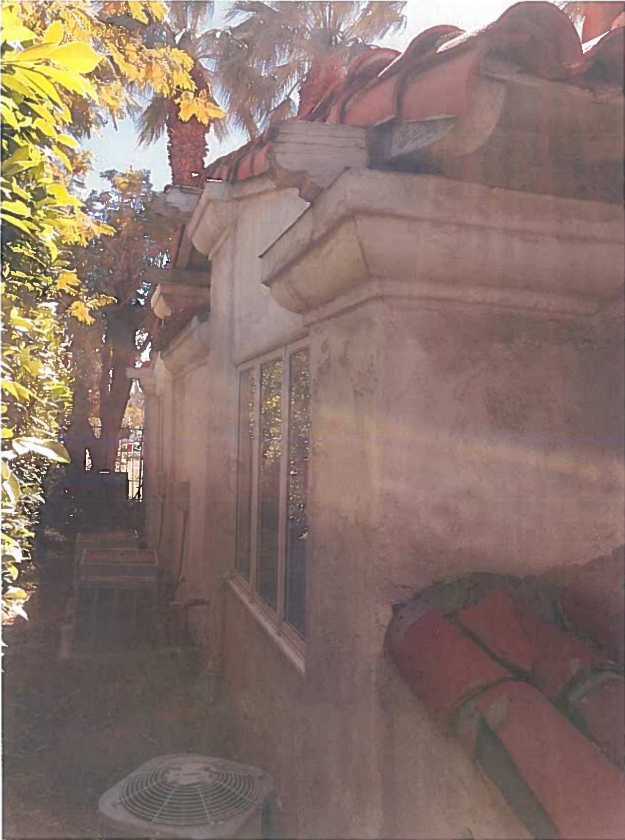
Photo 31 Harlow Haven Bldg D east elevation
