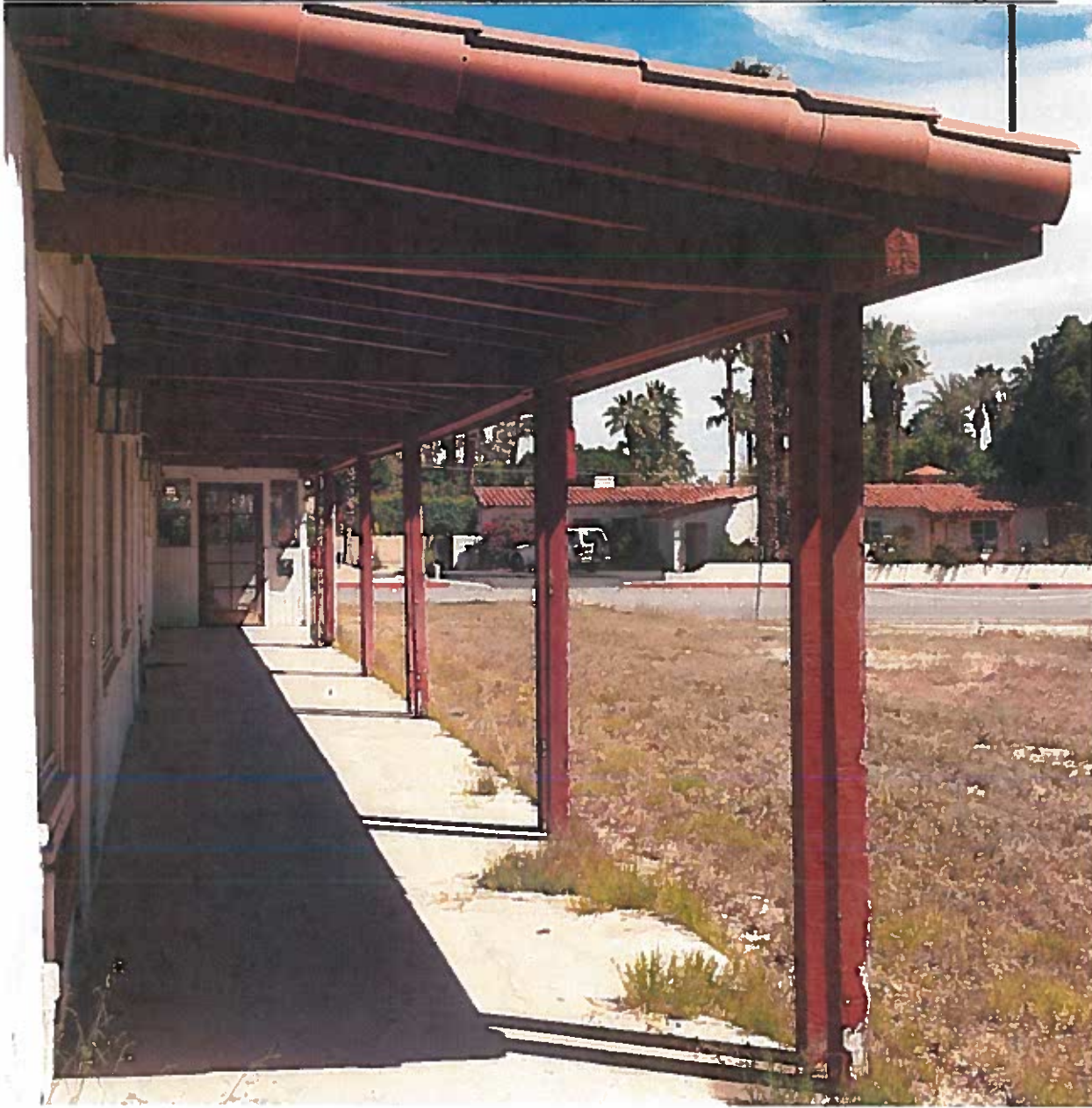
Photo 3: Crawford Apartments: Building "A" view of covered front porch looking east.
