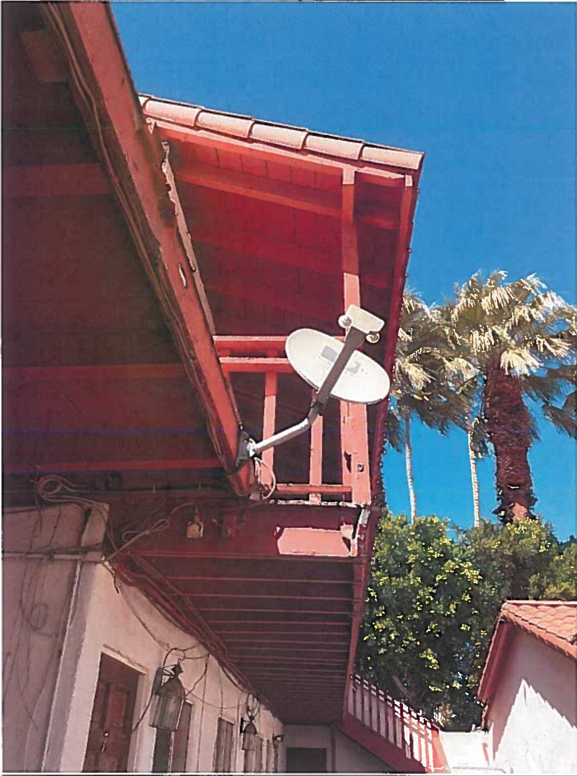
Photo 11: Crawford Apartments: Building "B" detail at upper balcony.
