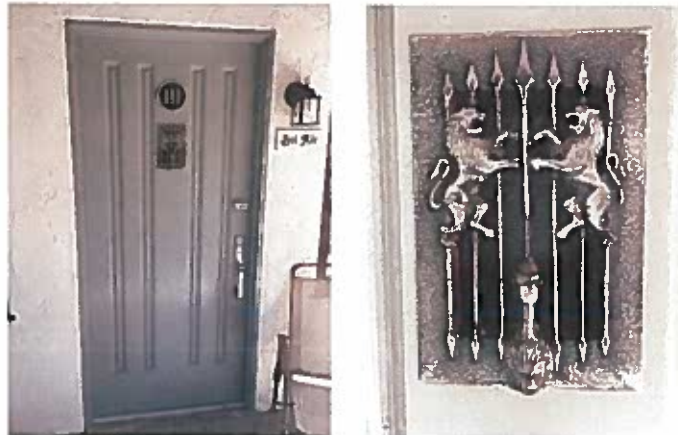
BELOW LEFT ARE THE EXISTING DOORS AT HARLOW HAVEN. THESE ARE PROPOSED TO BE REPLICATED FOR DOORS AT THE CRAWFORD APARTMENTS. BELOW RIGHT DETAIL OF THE PEEP HOLE GRILL
