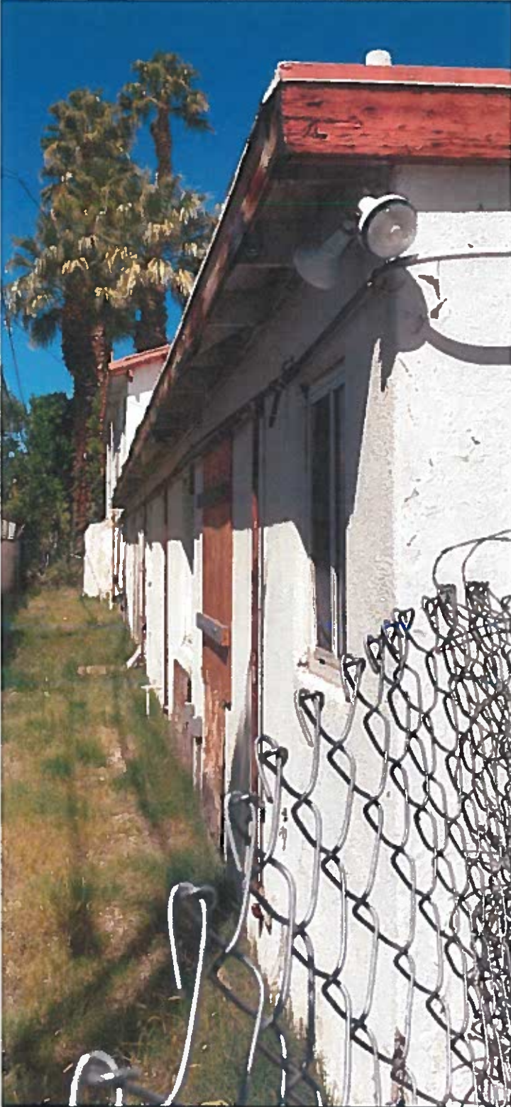
Photo 7: Crawford Apartments: Building "B" West façade.
