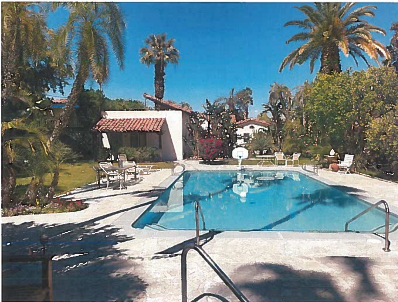
Photo 45 Harlow Haven pool courtyard Bldg C background left, building D background to the right
