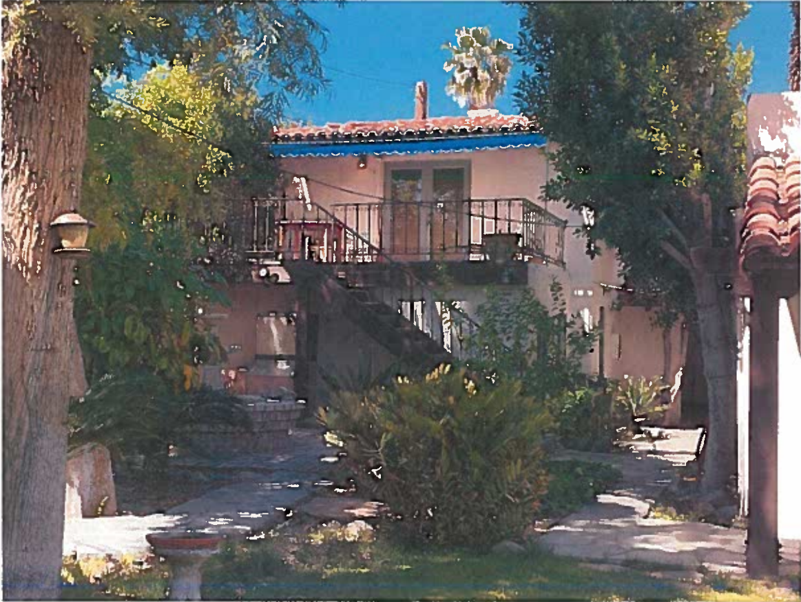
Photo 47 Harlow Haven Bldg C south elevation
