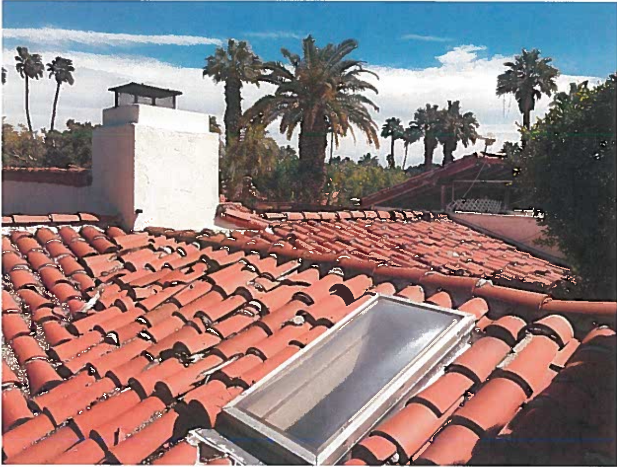
Photo 19 Harlow Haven roof of Bldg C
