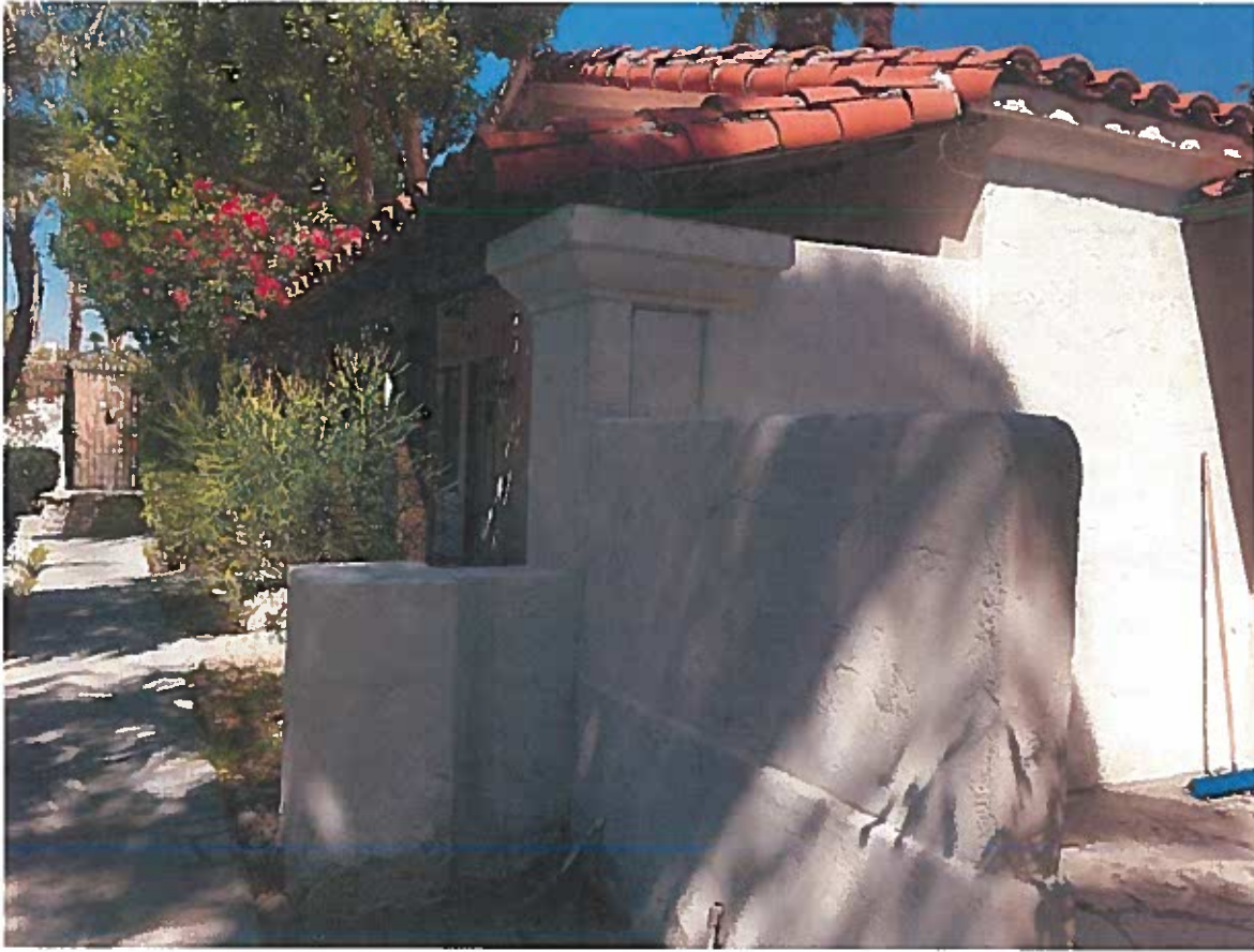
Photo 39 Harlow Haven Bldg D west elevation typical patio wall, at left walkway to north gate
