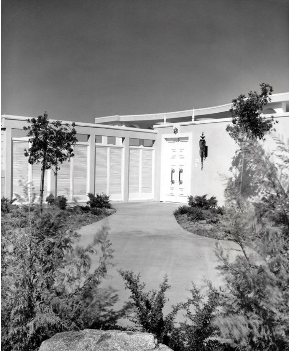
A 1965 view of the home’s entry. Note the louvered doors, which could be opened to facilitate airflow if desired. These have since been filled in. (Courtesy Estate of James H. McNaughton/Robert Miller)
