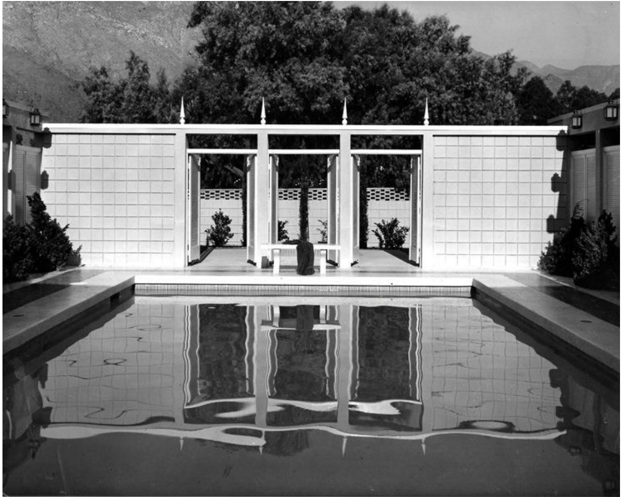
A 1965 view looking towards the front garden from across the pool/central courtyard. Note the four finials, since removed, and the walls, which were incised to appear as square blocks, another McNaughton favorite.
