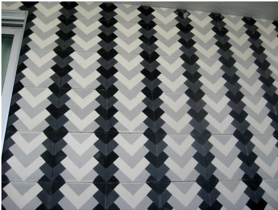
Detail of encaustic tiles in central courtyard added by the current owner. (Author Photo. February 2019)
