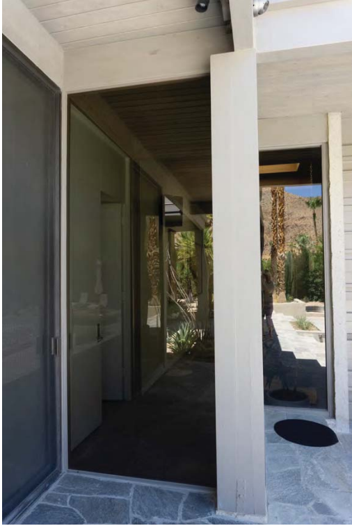
Image 22: West elevations: Window treatments hallways paving
