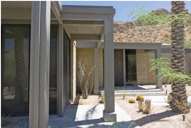
Image 7: Living room east wall and overhangs at left, entry and steps at right
