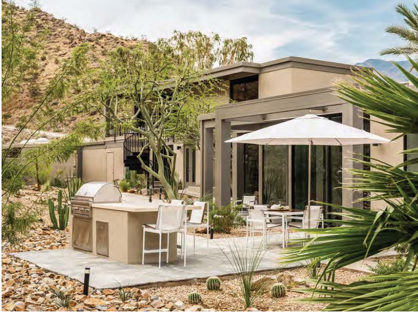
Image 19: East elevation, showing guest house and second story to left, rear of kitchen in main house to right. Photo: Lance Gerber
