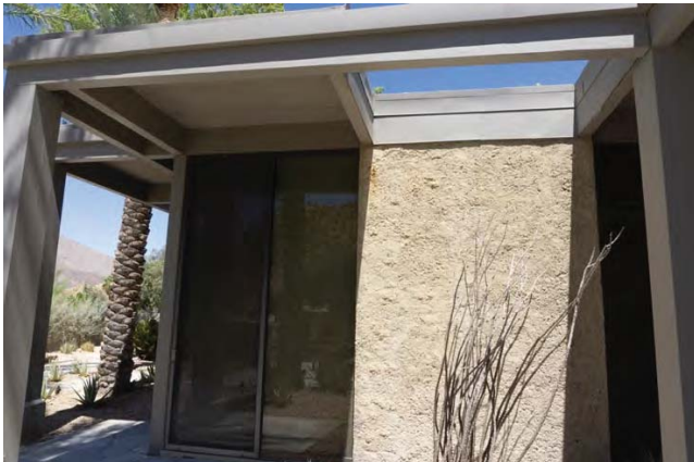
Image 8: Living room wall, east. Effect of sun through skylight on tilt-up panel
