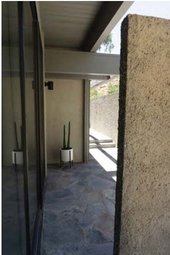
Image 13: Guesthouse, ground floor details, west elevation, looking south.
