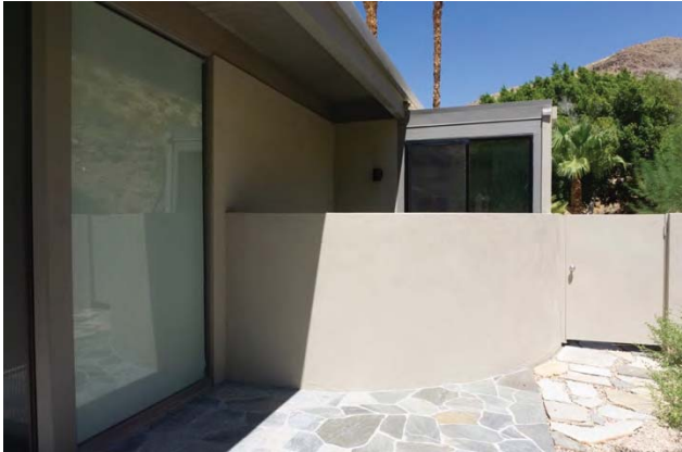
Image 21: East elevation. Curved patio wall outside master bathroom, east elevation.
