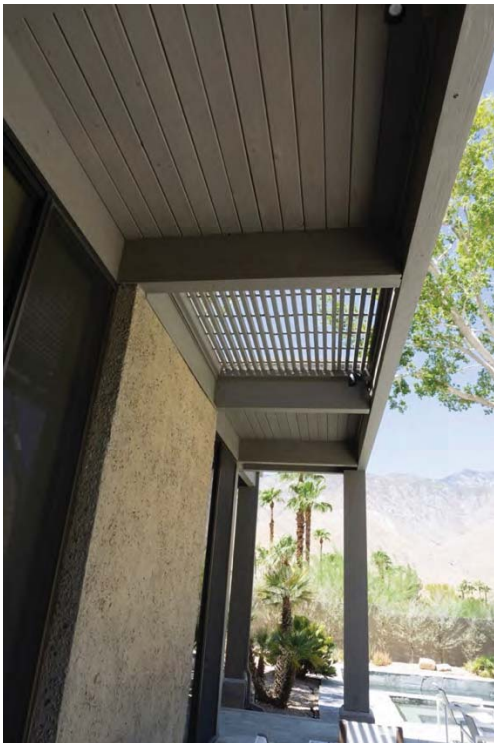
Image 24: West elevation. Overhang detail, living room wall, north.
