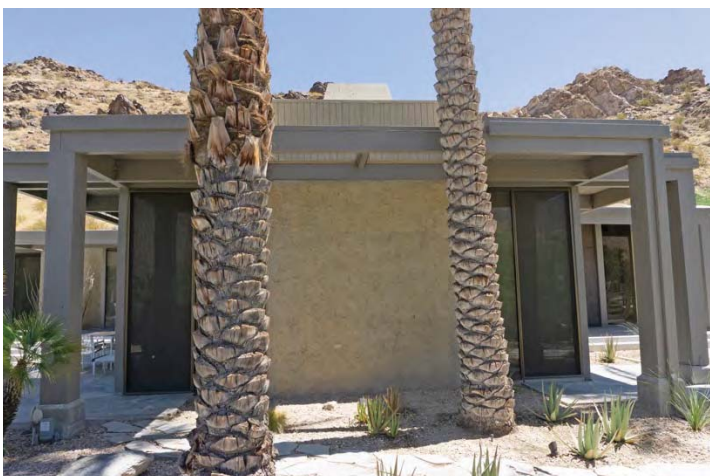
Image 5: Living room fireplace wall, west elevation
