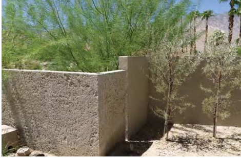
Image 15: Perimeter walls fronting property to street
