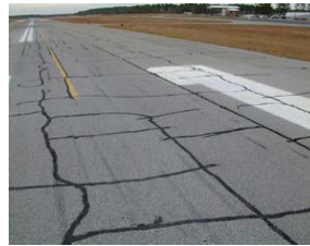
Block Cracking
