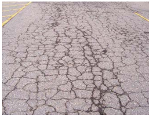
Alligator Cracking
