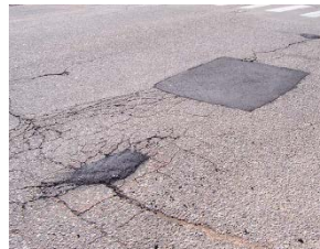
Patching and Utility Cuts
