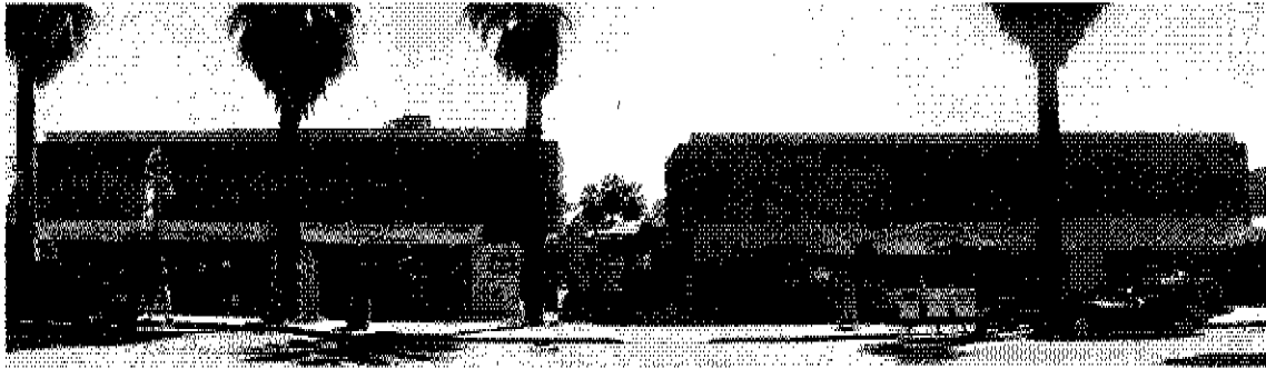
Figure 8 Current image of the twin buildings at 156-174 North Palm Canyon Drive. The passage to the Courtyard is partially blocked by an outdoor seating area. Contemporary in detail, these "twins" reflect a Beaux-Arts sensibility more typical of Paul R. Williams' work. Palm Springs has no other examples of this kind of pairing.
