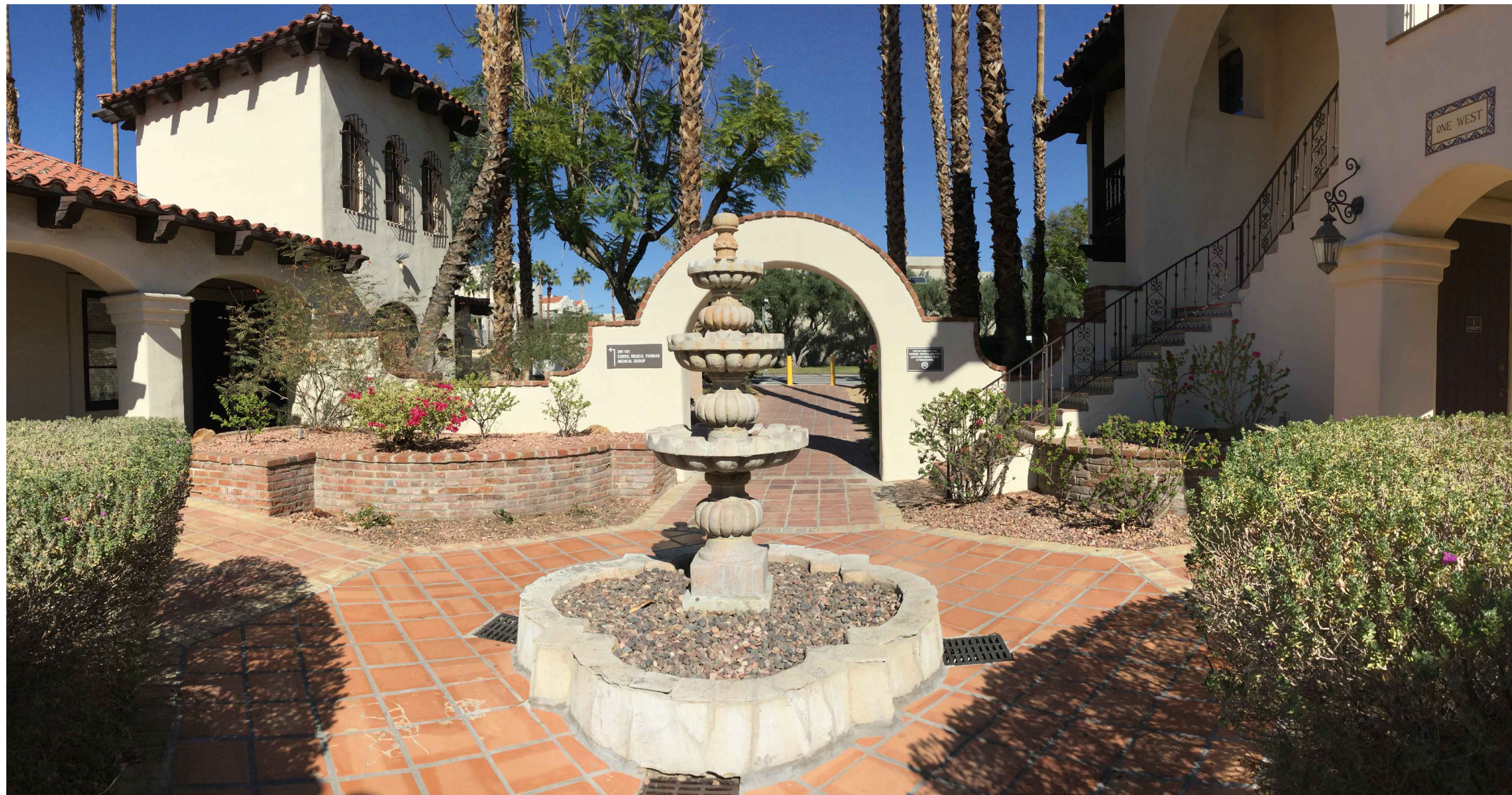
BEFORE INTERIOR COURTYARD WITH FOUNTAIN
