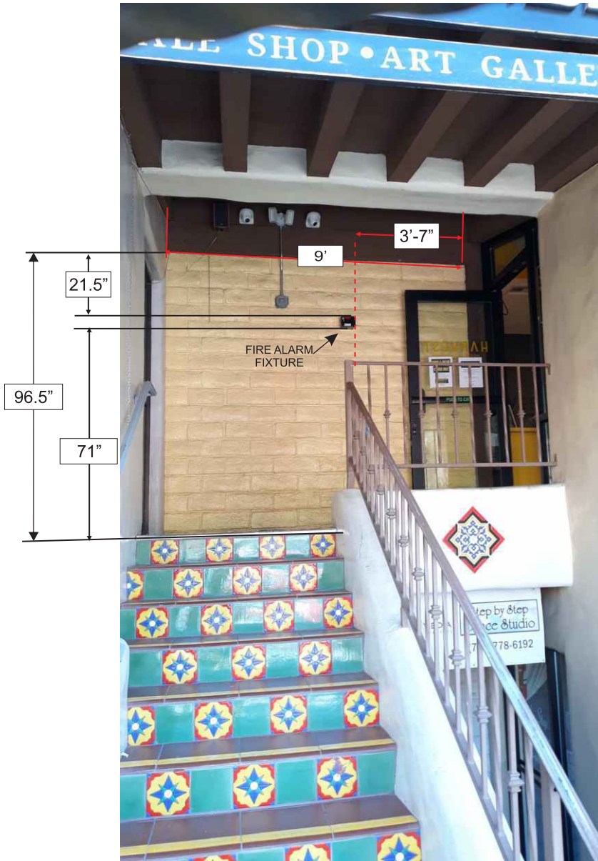
EXTERIOR ENTRANCE 2ND FLOOR
