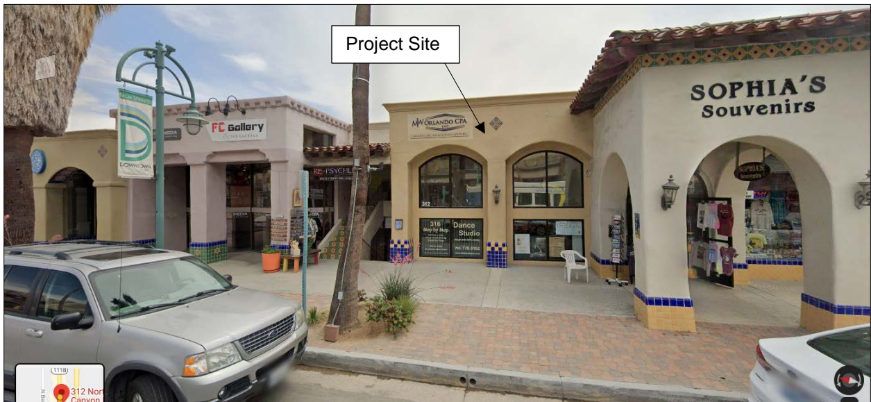
Image 1.2 Primary Elevation (North Palm Canyon Drive)
