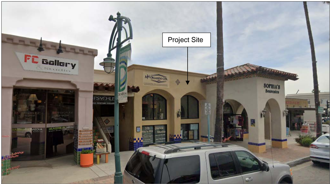
Image 1.3 Primary Elevation (North Palm Canyon Drive)
