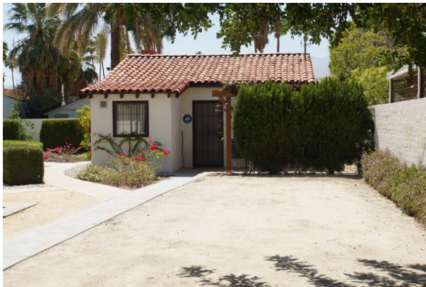
Building B, north façade. ( South view )
