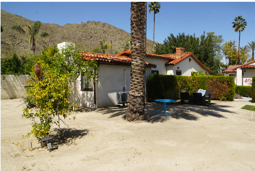
Building B, south and east façades. ( Northwest view )
