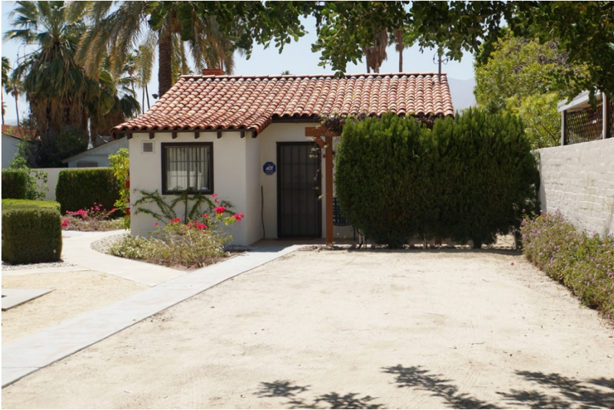
Building B, north façade. ( South view )
