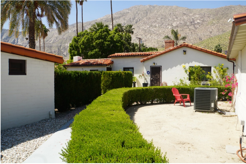
Building D (left) and Building B (center). ( West view )
