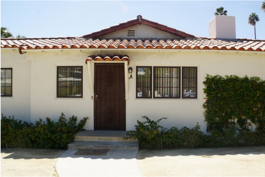
Building A, north façade, entrance detail. ( South view )
