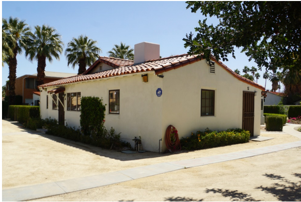
Building A, north and west façades. ( Southeast view )
