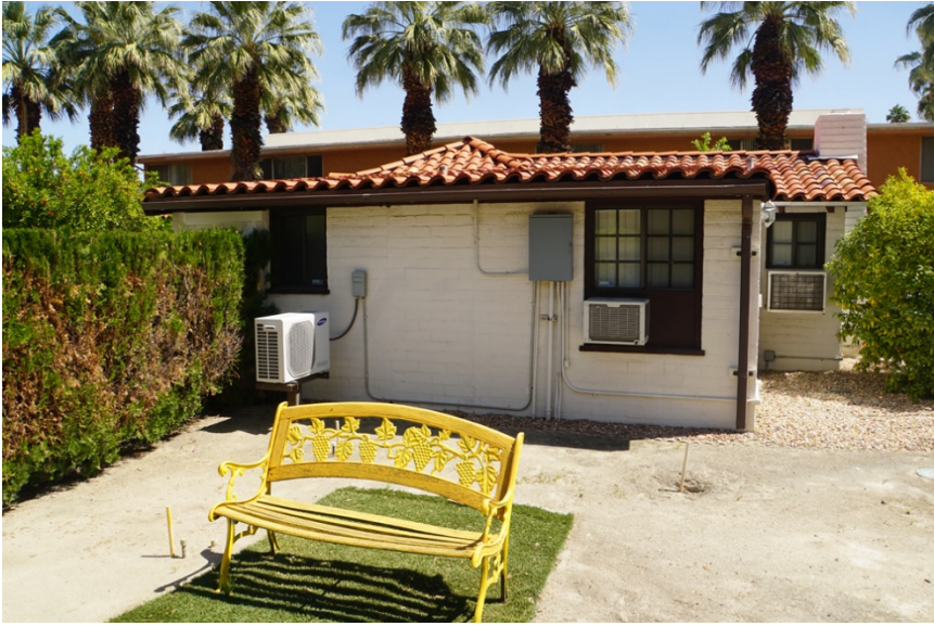
Building D, west façade. (East view)
