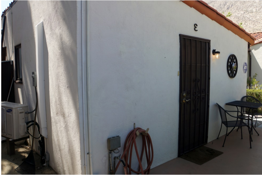
Building C, east and north façades. ( Southwest view )
