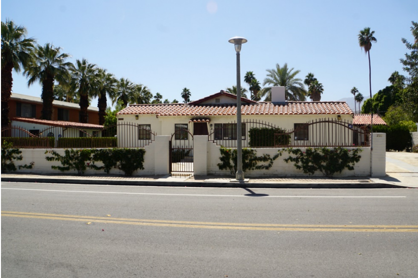
Subject Property, view from W. Arenas Road. ( South view )
