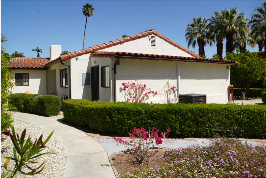
Building A, west and south façades. ( Northeast view )
