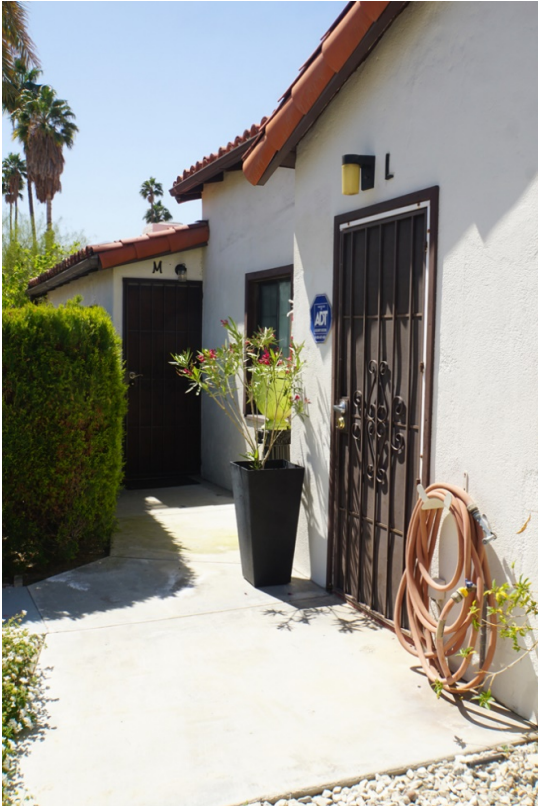
Building B, east façade, rear detail. ( Southwest view )
