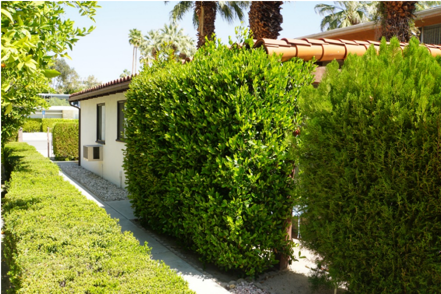
Building C, west and south façades. ( Northeast view )
