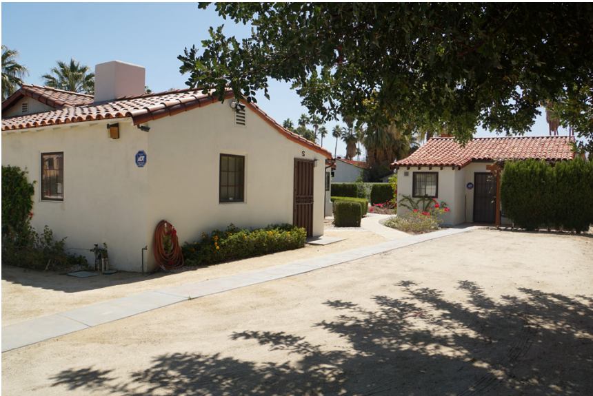
Building A (left) and Building B (right). (Southeast view)
