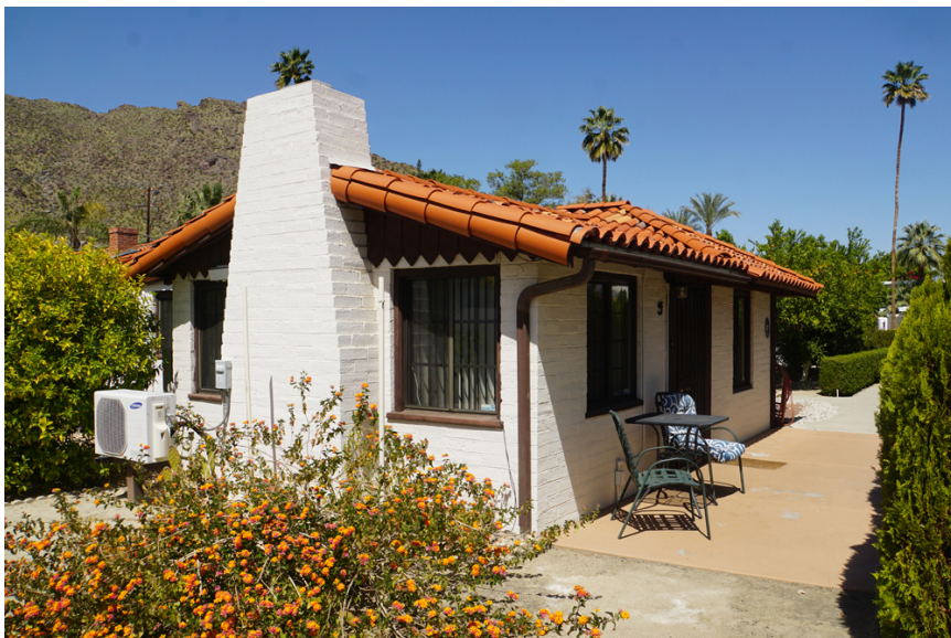
Building D, south and east façades. ( Northwest view )
