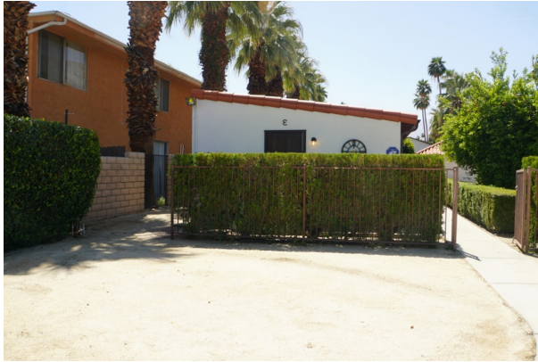
Building C, north façade. ( South view )
