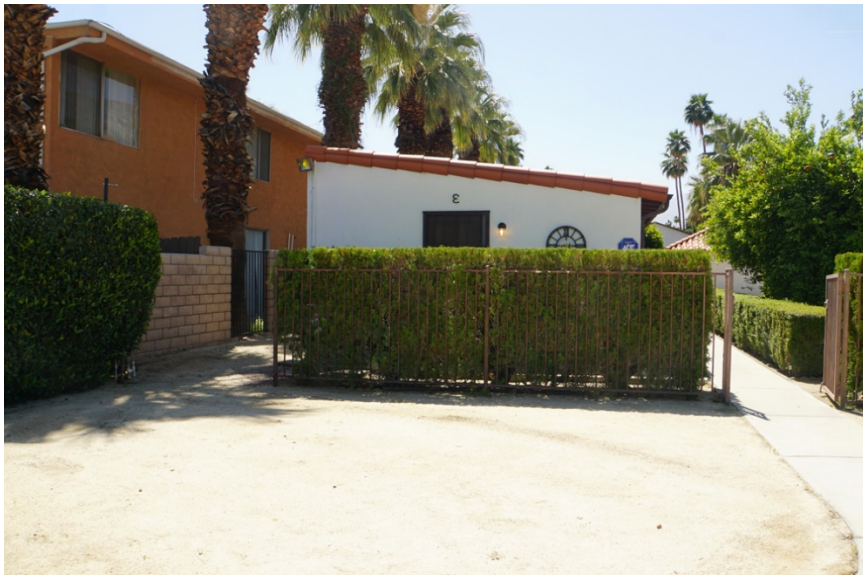
Building C, north façade. ( South view )
