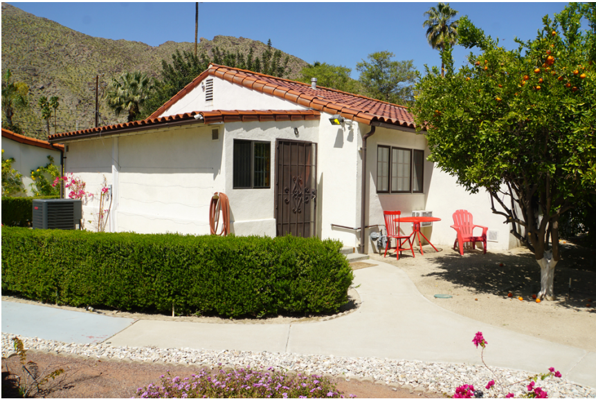
Building A, south and east façades. (Northwest view)
