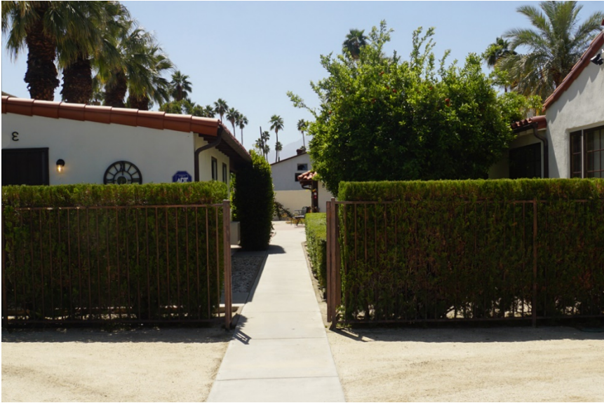
Central entrance, Building C (left) and Building A (right). ( South view )
