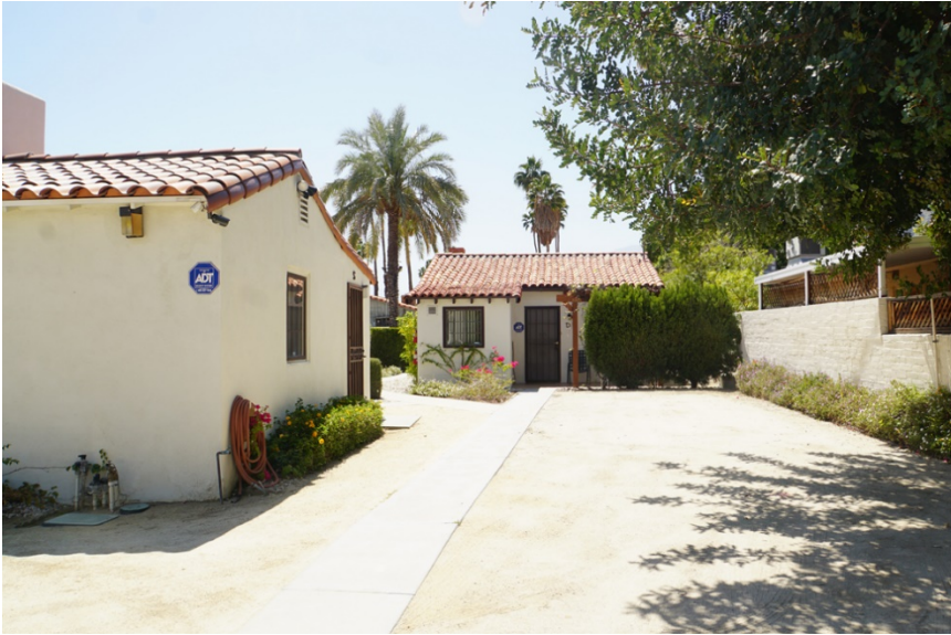
Building A (left) and Building B (center). (South view)
