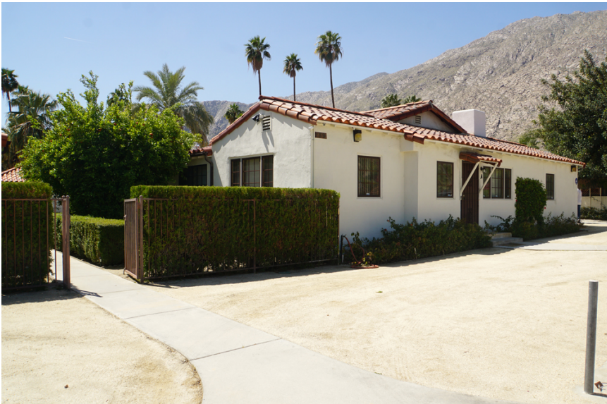
Building A, north and east façade. ( Southwest view )
