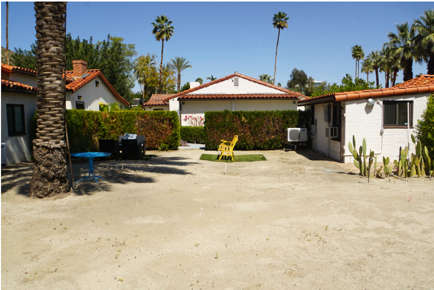
Courtyard, Building B (left), Building A (center), and Building D (right). ( North view )
