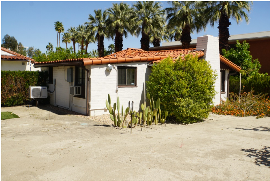
Building D, west and south façades. ( Northeast view )
