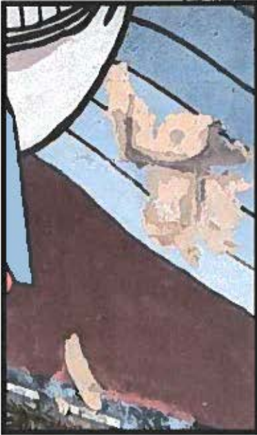
Detail photo of deterioration & severe fading of paint on mural
