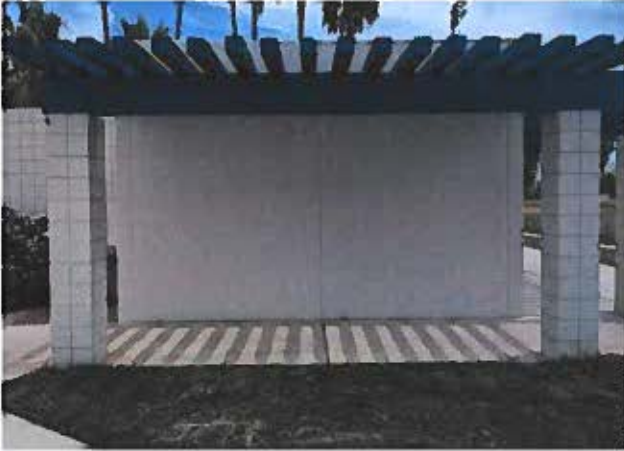
Demuth Park-Baseball Field Concession Building-(close up photo)
