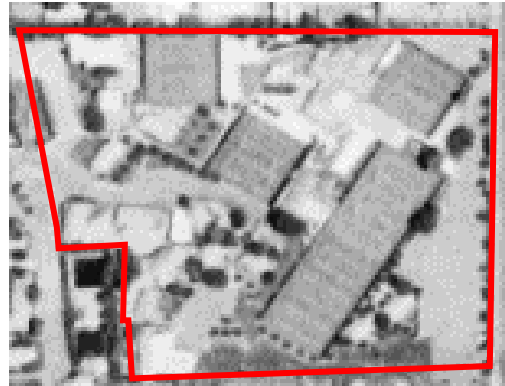
1980 aerial photograph. Source: UCSB Aerial Photography Collection.
