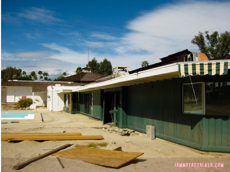
Clubhouse building, view facing northwest. Source: Lindsay Blake, iamnotastalker.com, 2008.
