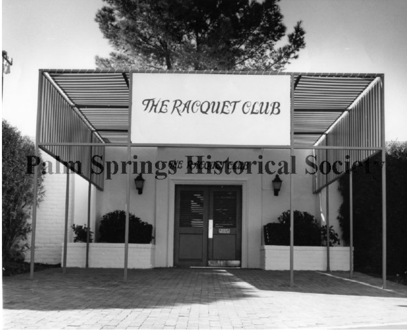
Racquet Club front entrance and entry canopy, c. 1965. Source: Palm Springs Historical Society.
