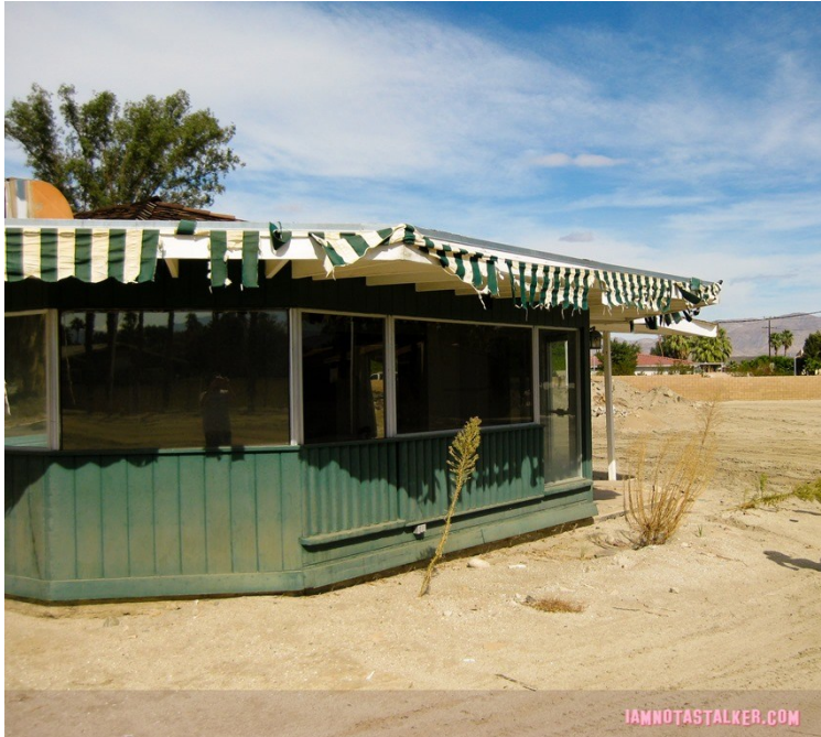
Clubhouse building, view facing northwest. Source: Lindsay Blake, iamnotastalker.com, 2008.
