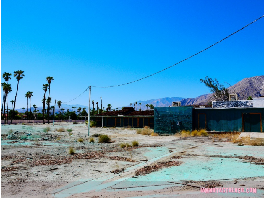
Clubhouse building, view facing southwest. Source: Lindsay Blake, iamnotastalker.com, 2008.
