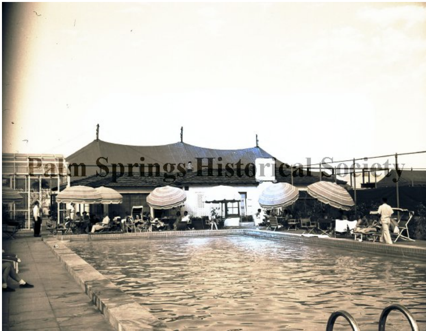
Main Pool and Clubhouse with tent behind, view facing northeast, date unknown. Source: Palm Springs Historical Society.
