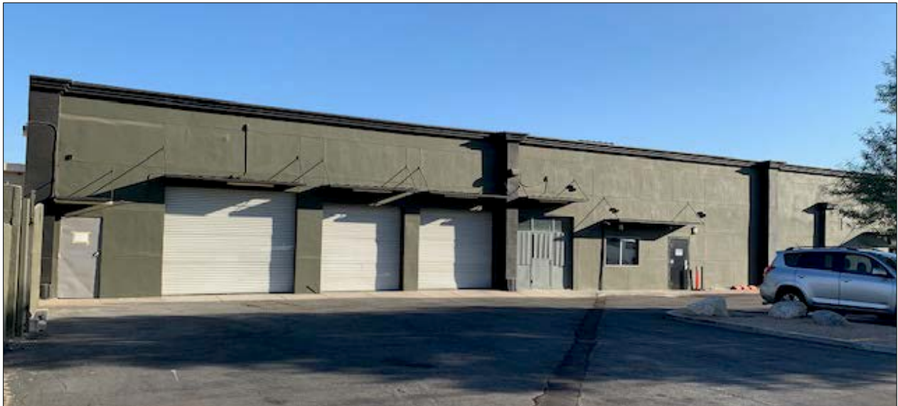
Image 1.9 Exterior Building Wall Colors
