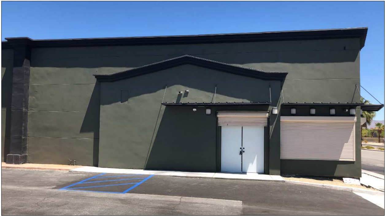
Image 1.8 Exterior Building Wall Colors
