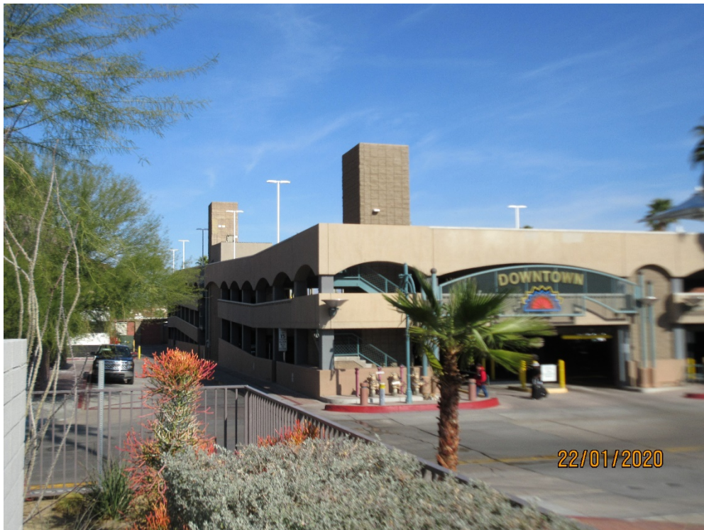
Elevator shaft from Belardo Road showing existing Verizon facility
