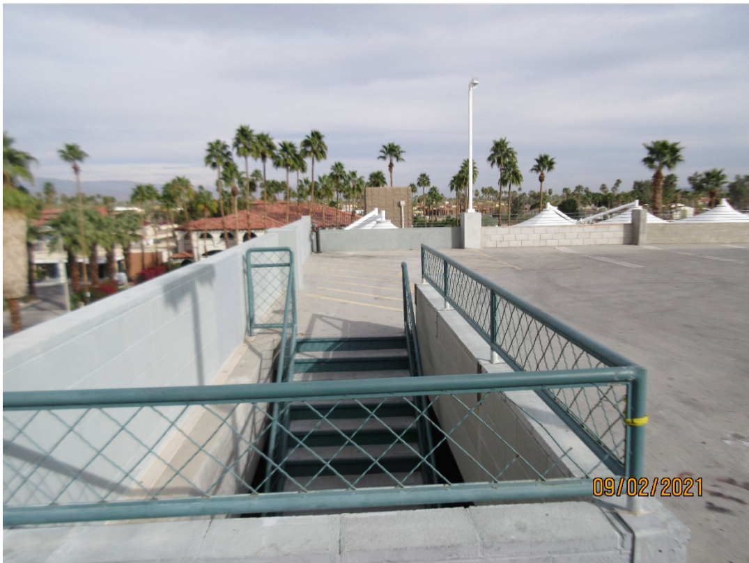
Location of new equipment shelter to left of light pole
