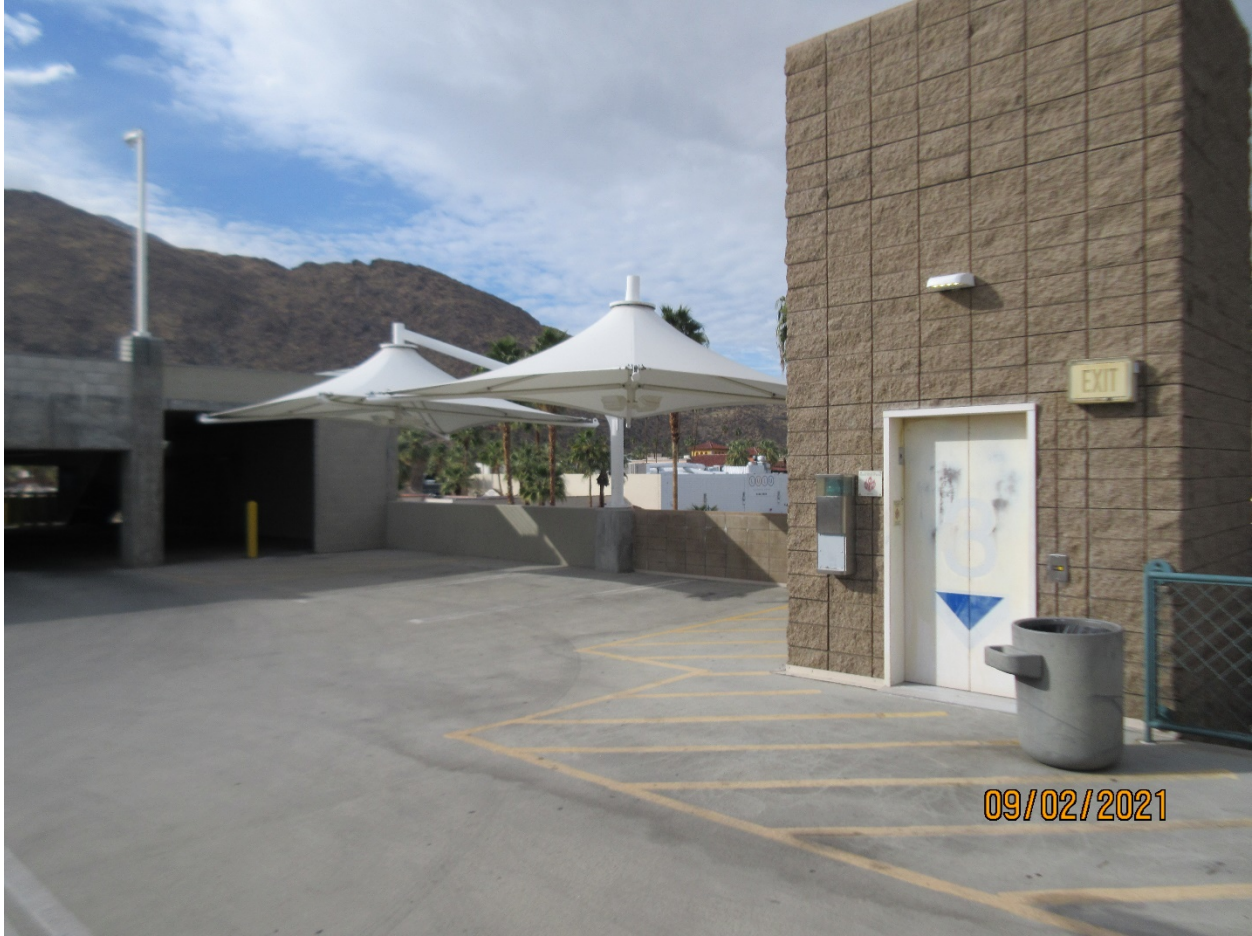
Location of new equipment shelter to the right of light pole in background
