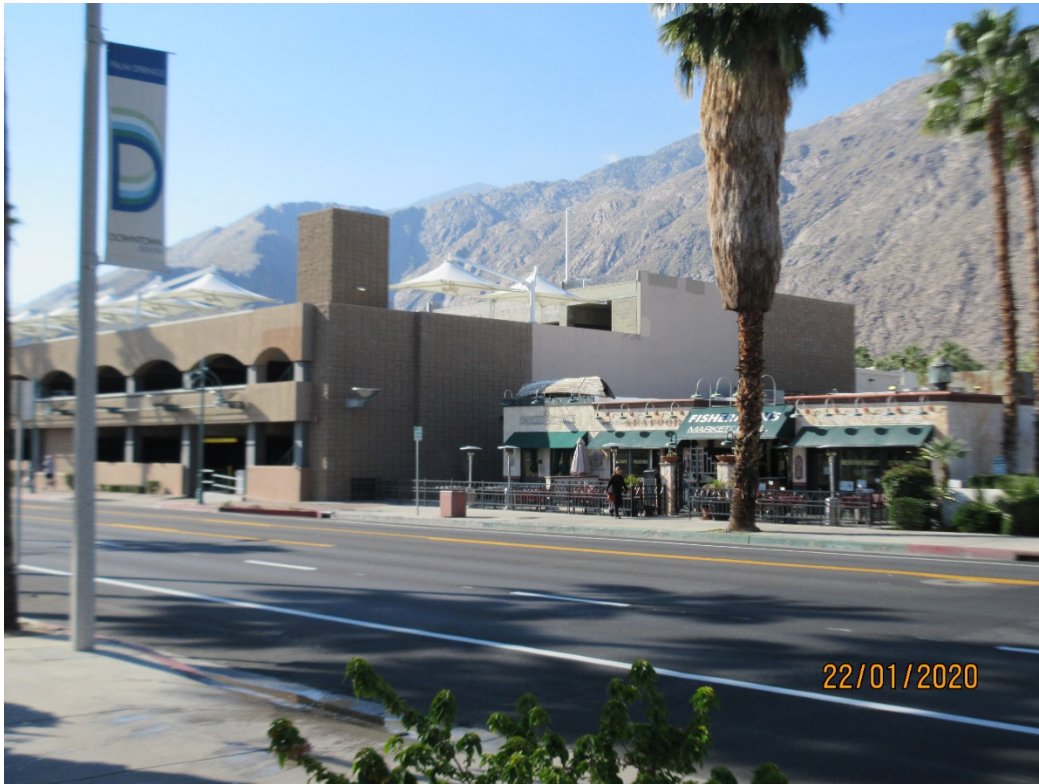
View of northeast elevator from street
