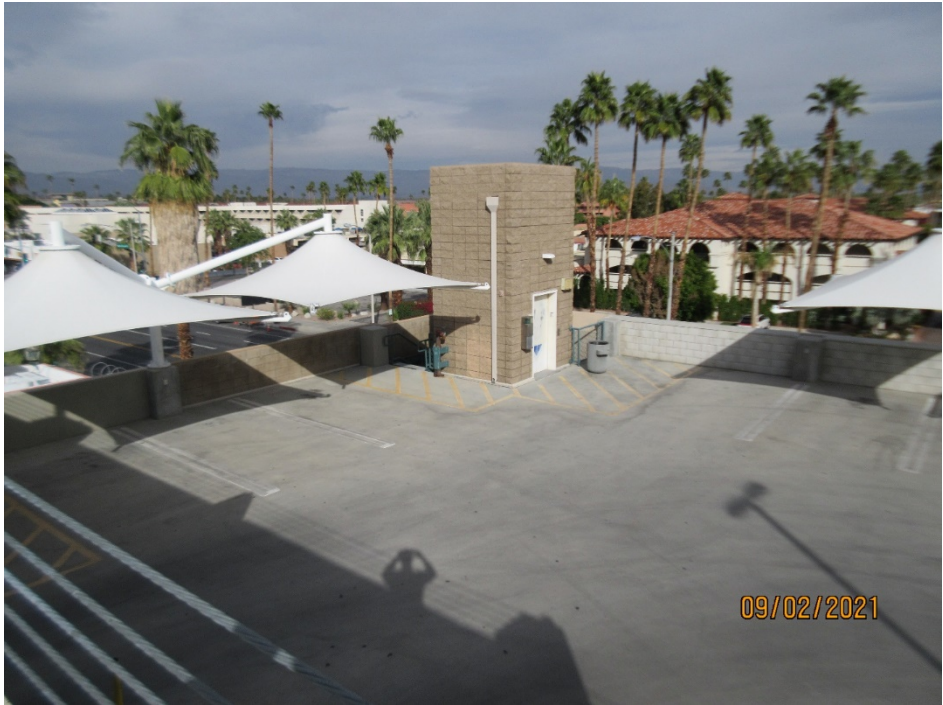
View of northeast elevator
