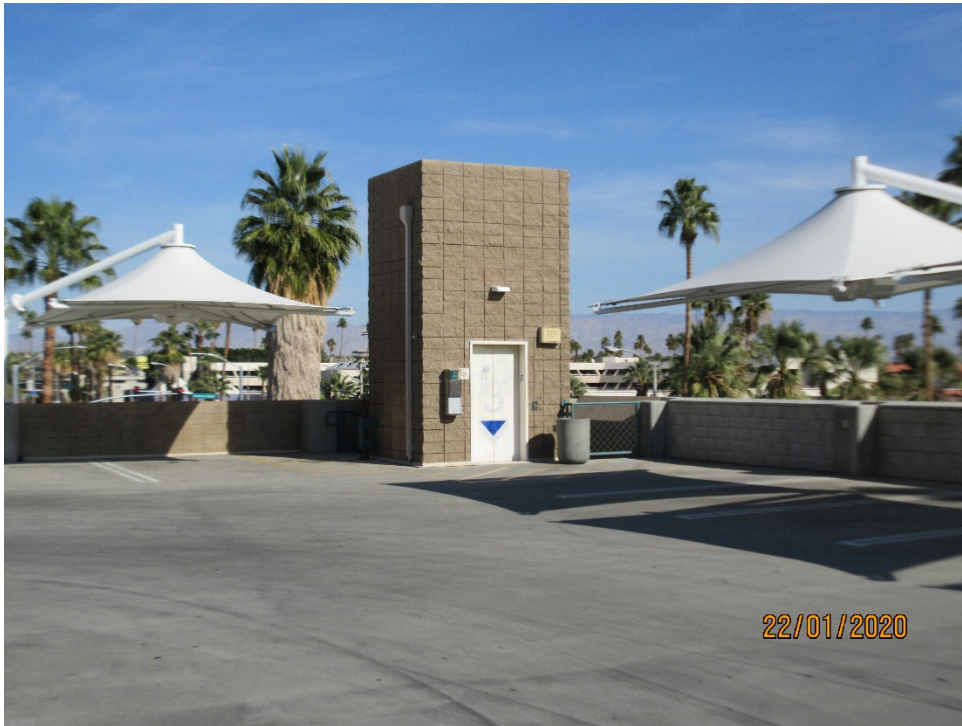
Northeast elevator shaft fronting South Indian Canyon Drive
