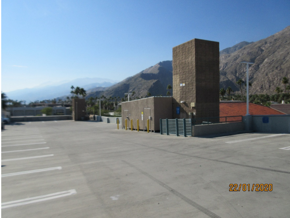
Existing Verizon facility look south toward southwest elevator shaft
