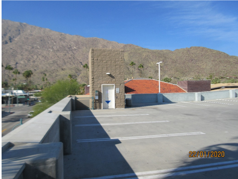
Southwest elevator shaft facing Belardo Road
