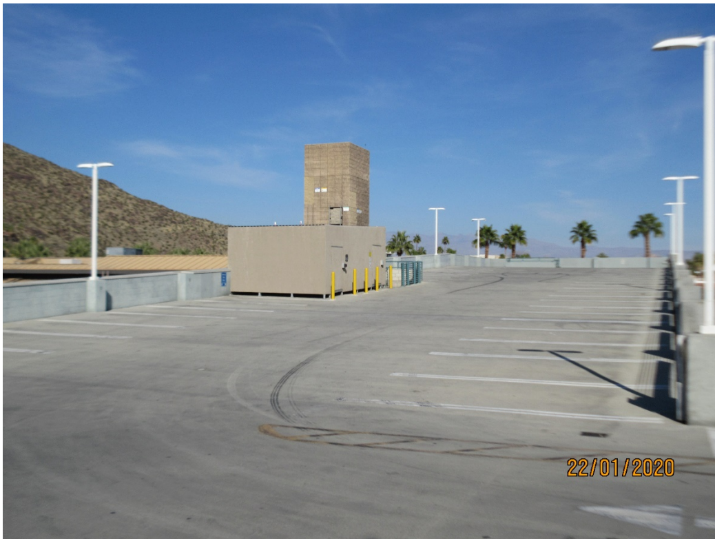
Existing Verizon facility and equipment enclosure
