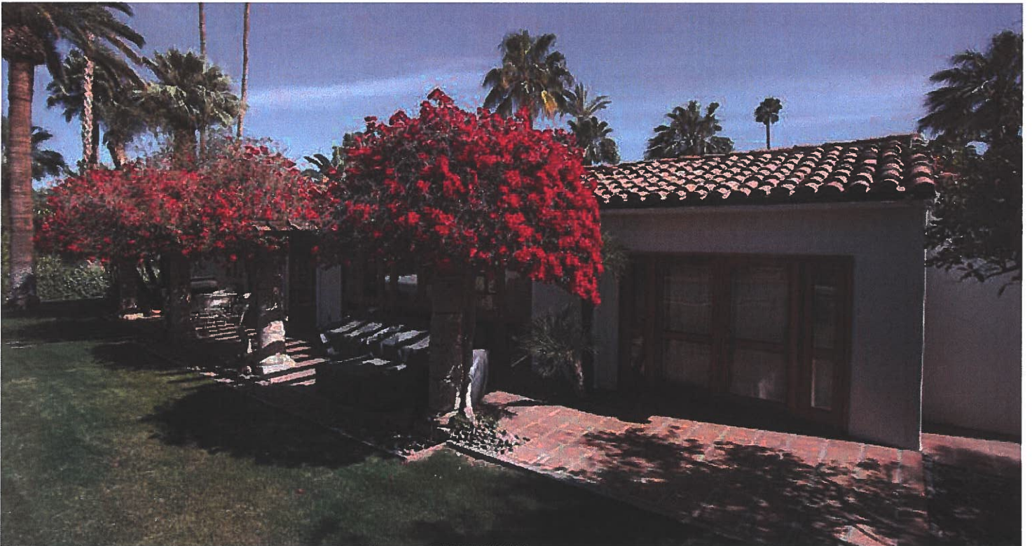
22 view southeast from backyard toward bedroom 3 (right) and living room
