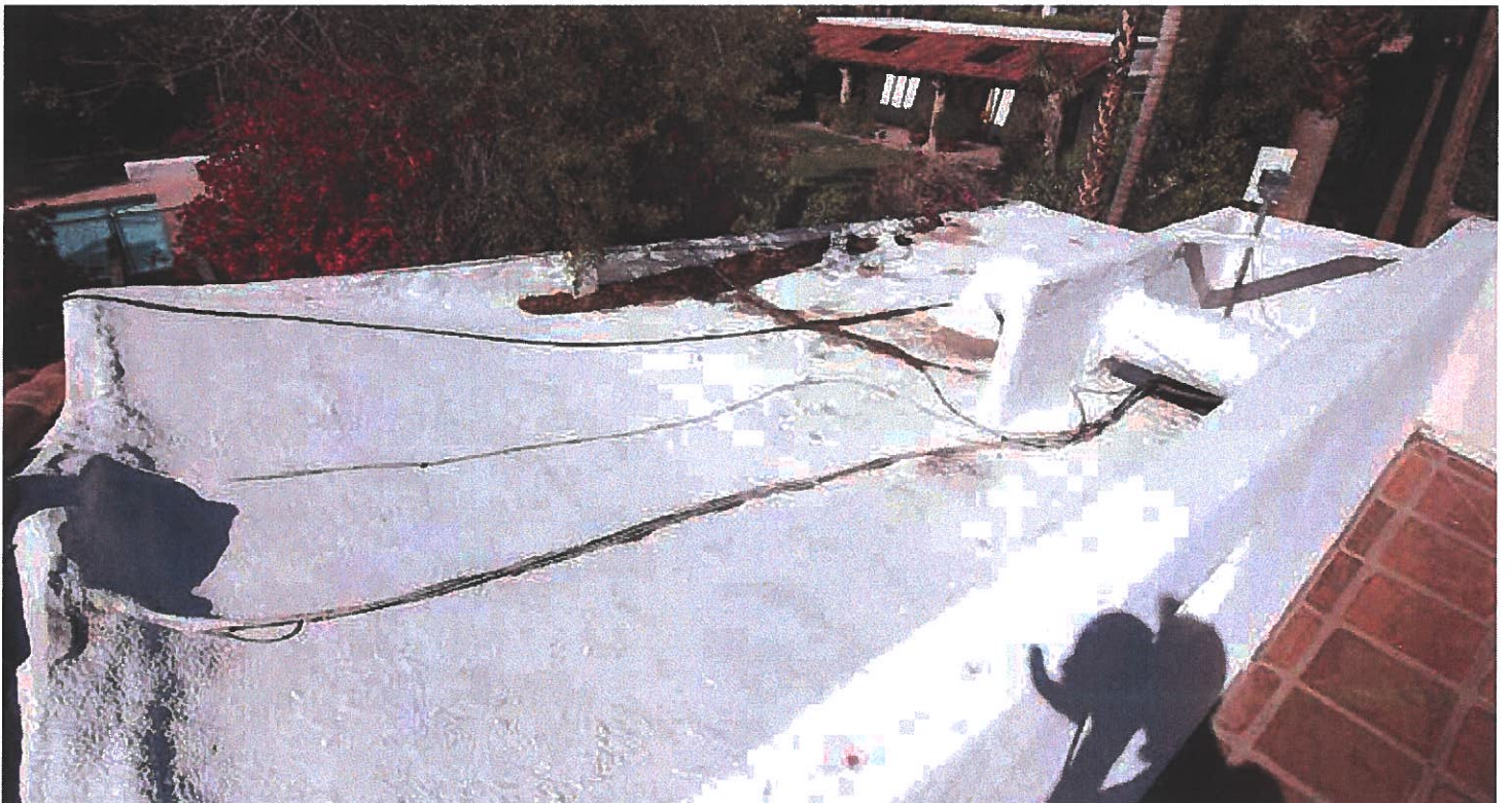
36 view north from roofdeck over kitchen roof
