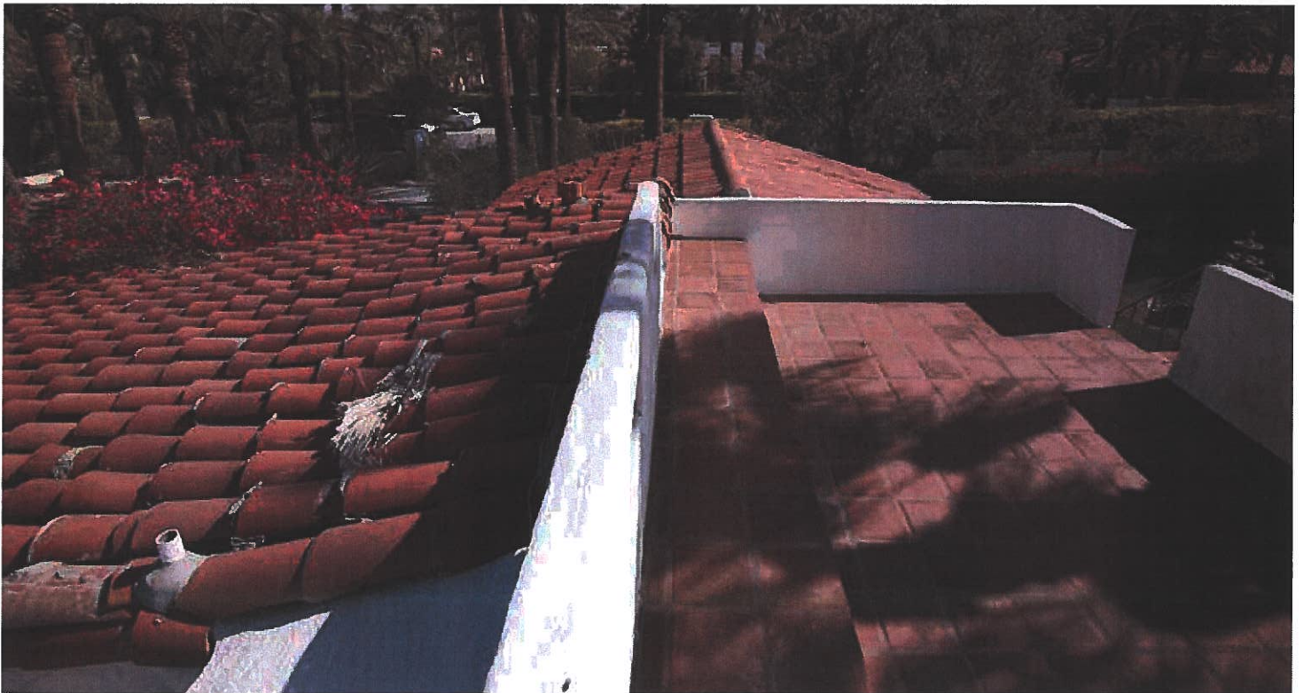
34 view south from roofdeck over bedroom 5 (left) and garage (in distance)
