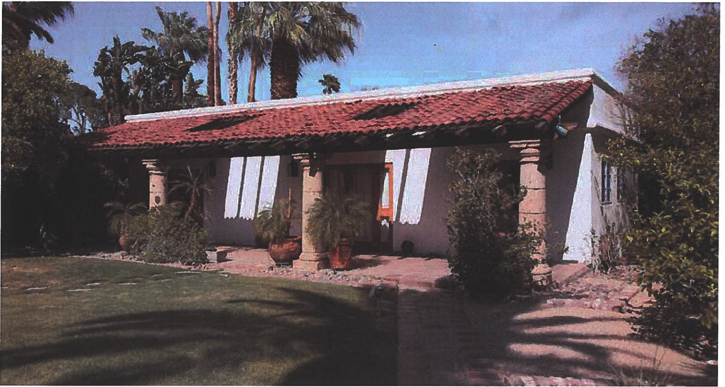
25 view northeast from backyard toward casita west elevation; note different covered patio style, and taller parapet wall with rounded stucco detail that was not common in the era of the original house
