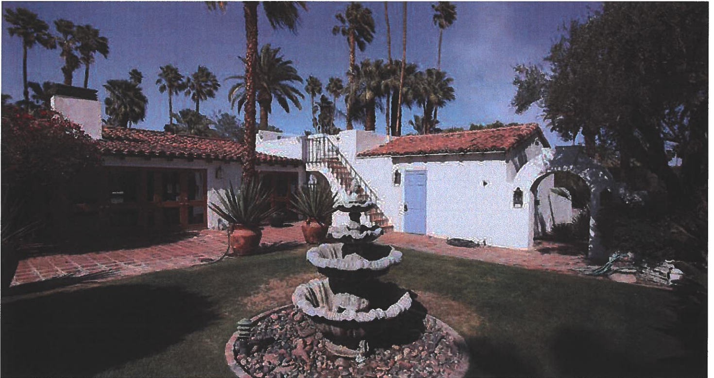
16 view northeast in central courtyard toward garage (right) and stairs to roofdeck; note the different roofline of garage and the poor integration of the roofdeck
