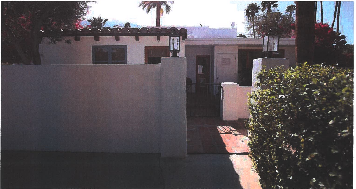
12 view west from driveway toward bedroom 5 (left) and kitchen (right); note the flat roof over kitchen
