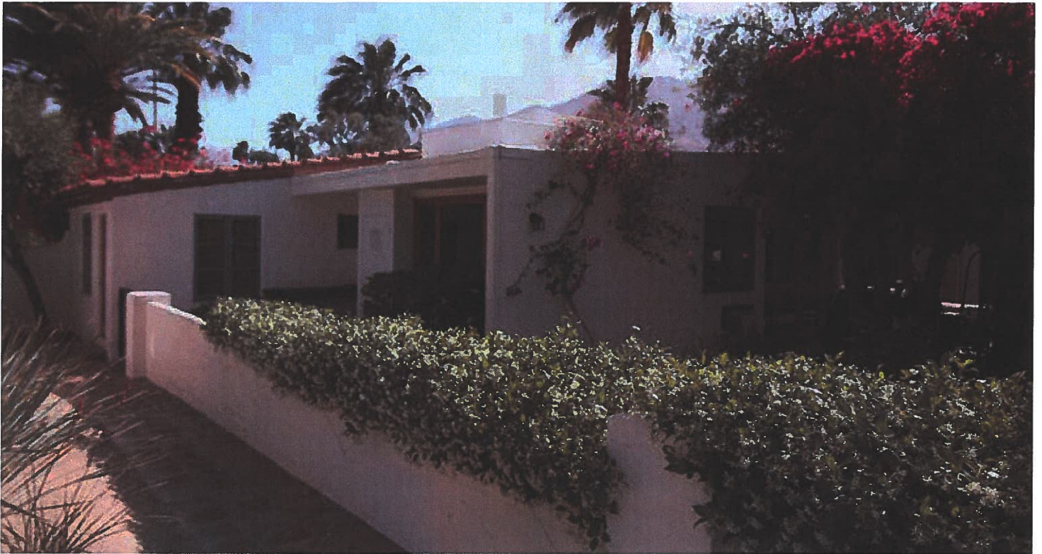
15 view southwest from back yard toward kitchen; note the flat roof and mechanical equipment on kitchen roof
