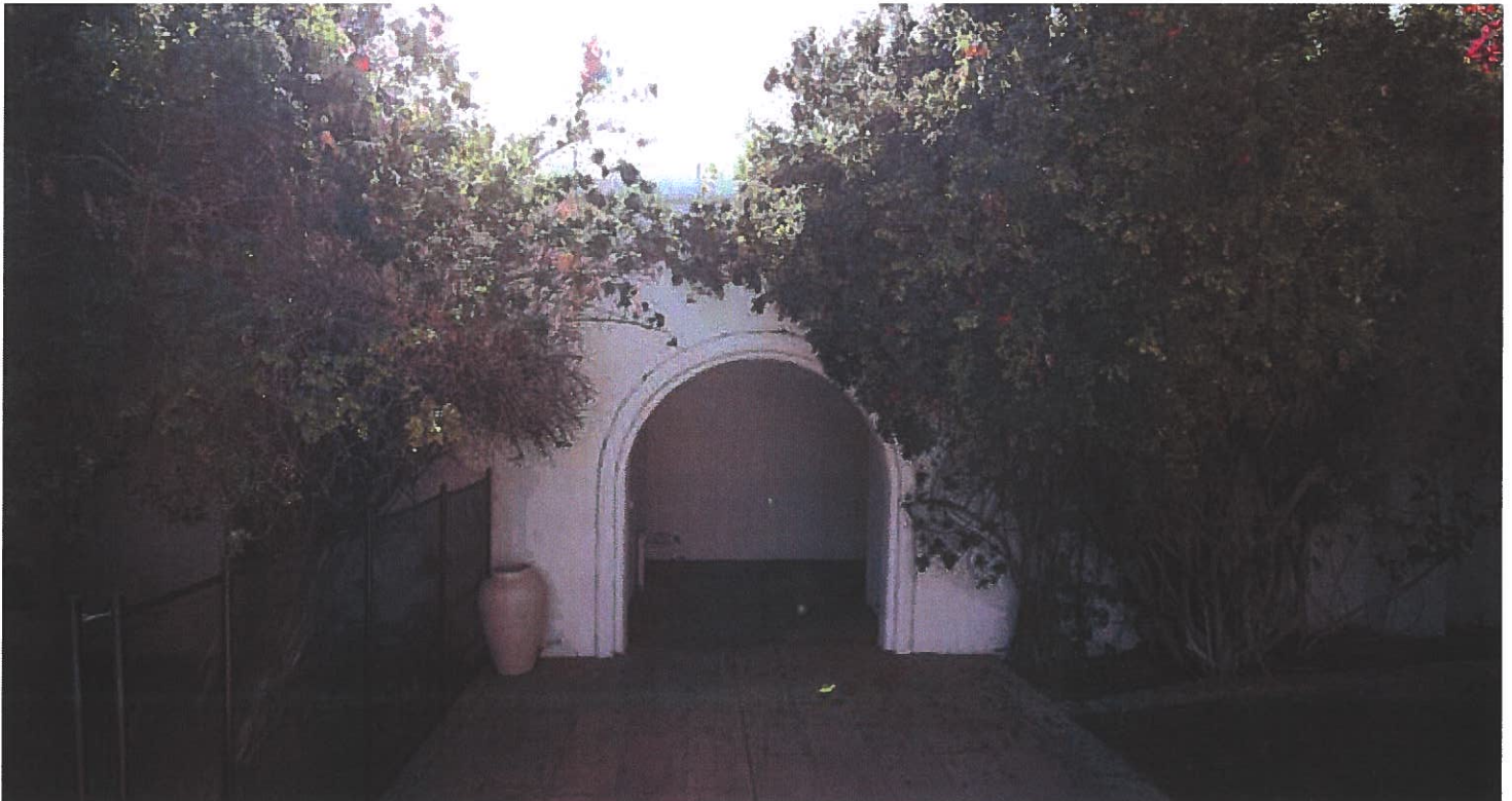
28 view west from pool of entrance to pool house
