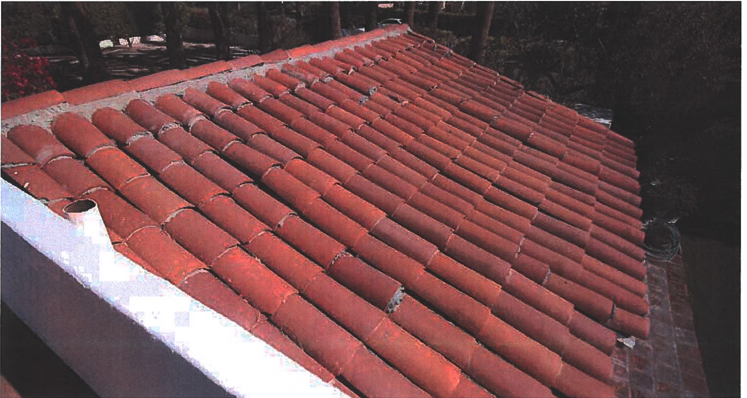
32 view south from roofdeck over garage roof
