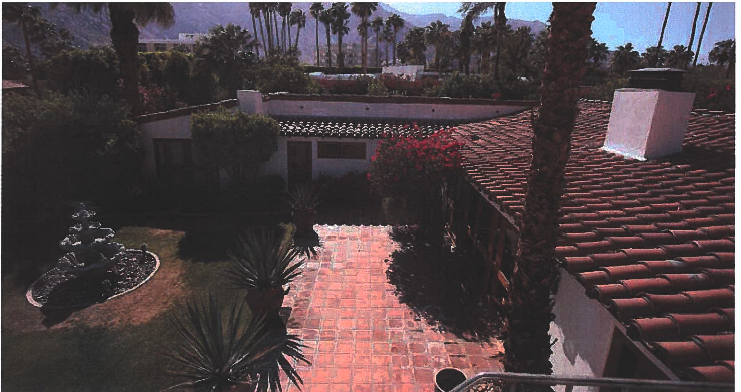
30 view west from roofdeck; not various rooflines that suggest a number of additions and renovations at various time periods
