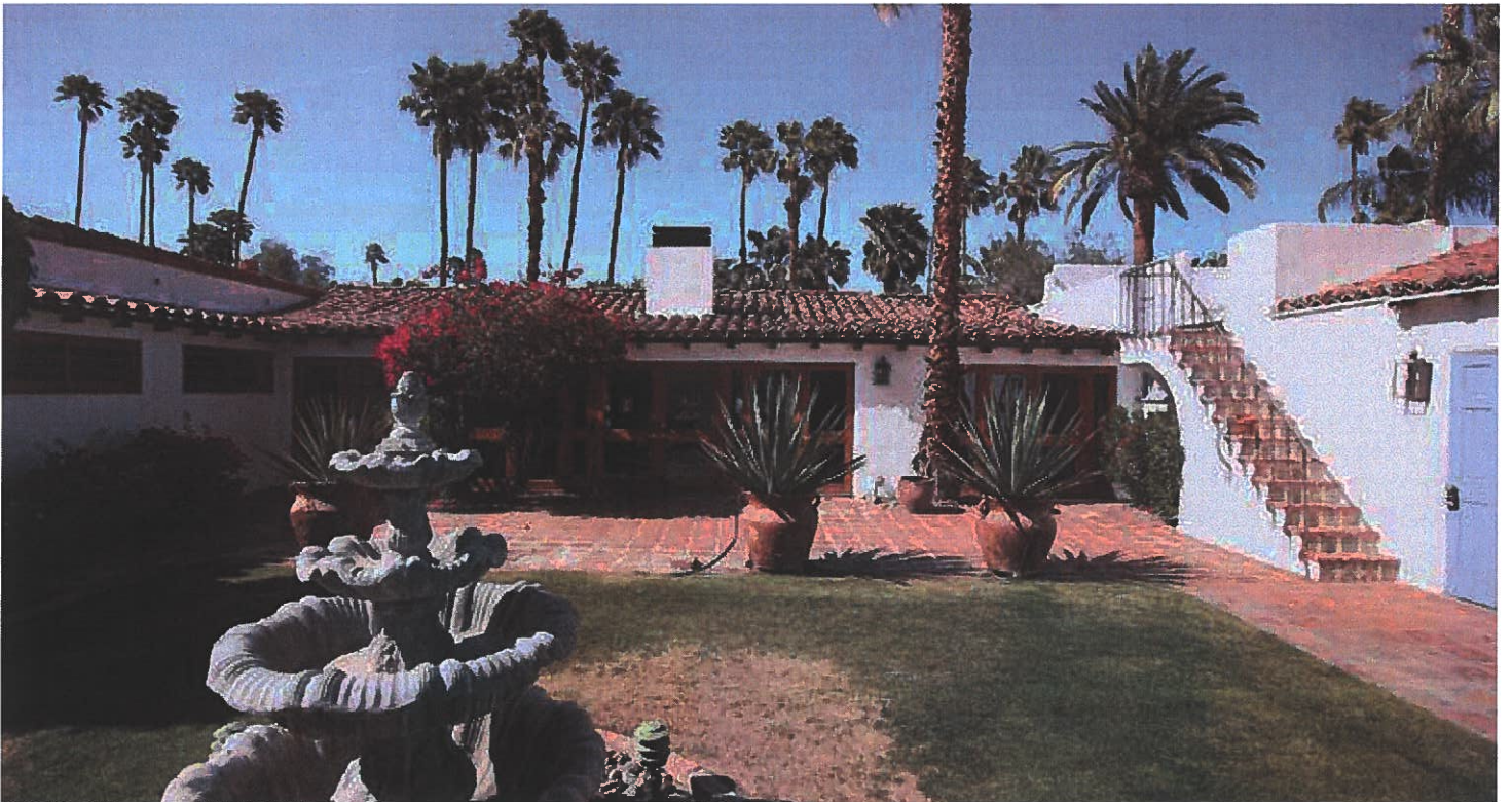
18 view north in the central courtyard with garage on right; this will be the view from the proposed new entrance gate into the courtyard
