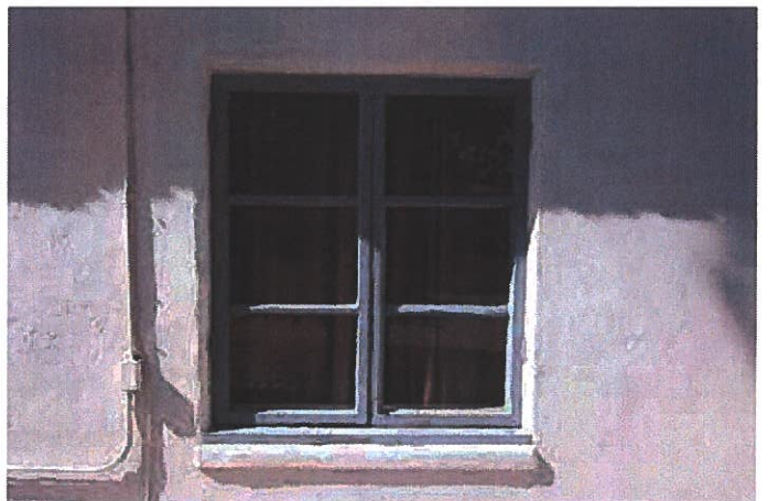
Existing french casement window style to be replicated by Loewen in aluminum-clad wood
