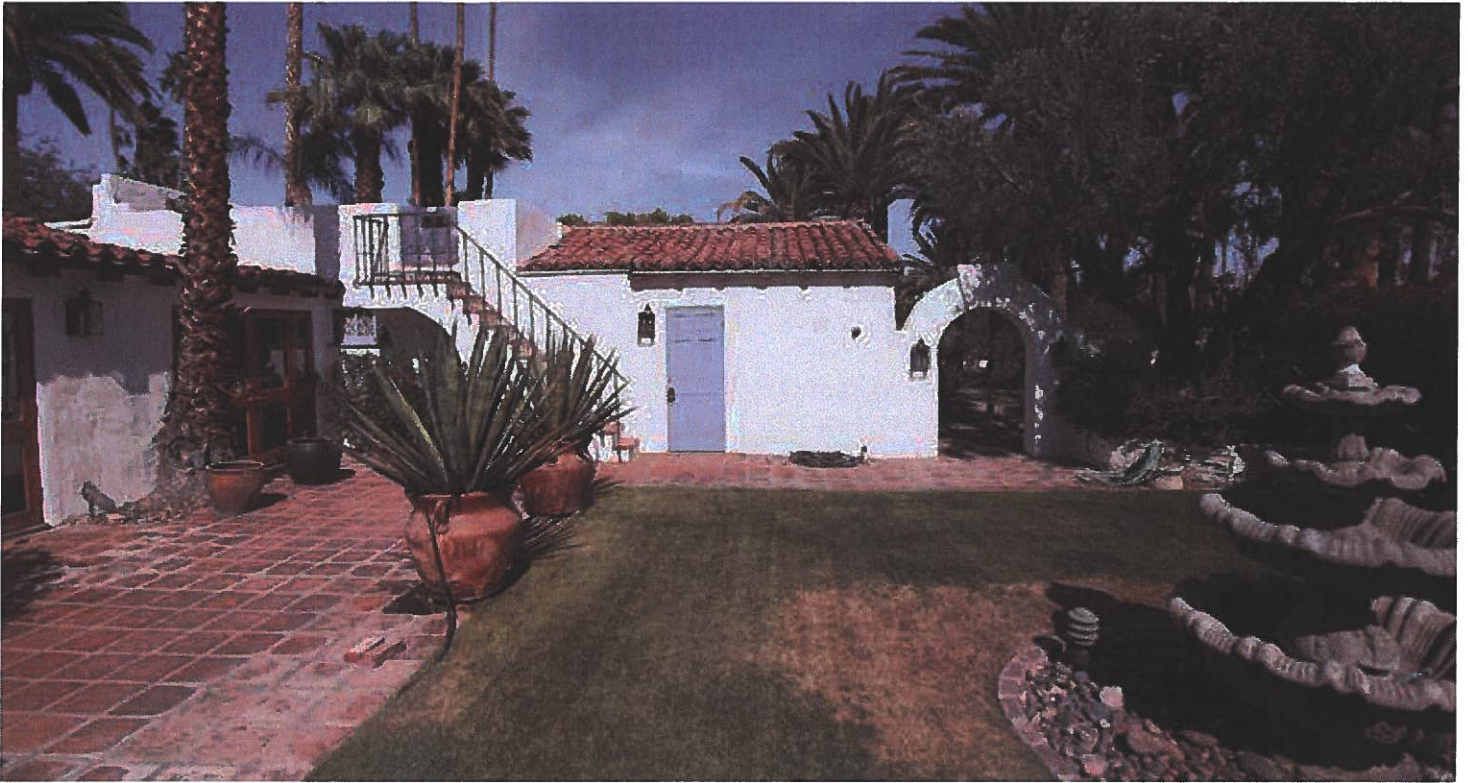
17 view east from courtyard toward garage; proposed owners' suite will replace the garage but replicate the gable roofline; owner's suite will have doors onto the courtyard
