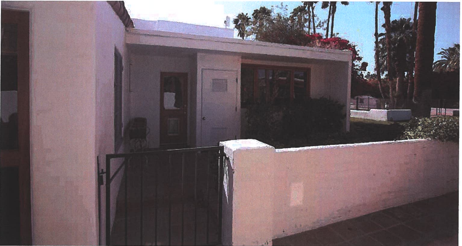
13 view west toward kitchen; note the flat roof and wing wall on right – details not more common in mid-century rather than Spanish revival
