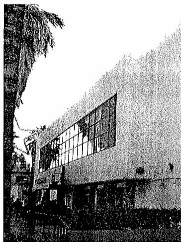
Oasis Commercial – North Facade
