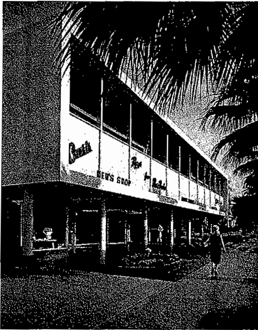
Palm Canyon elevation. (photo: Shulman)
