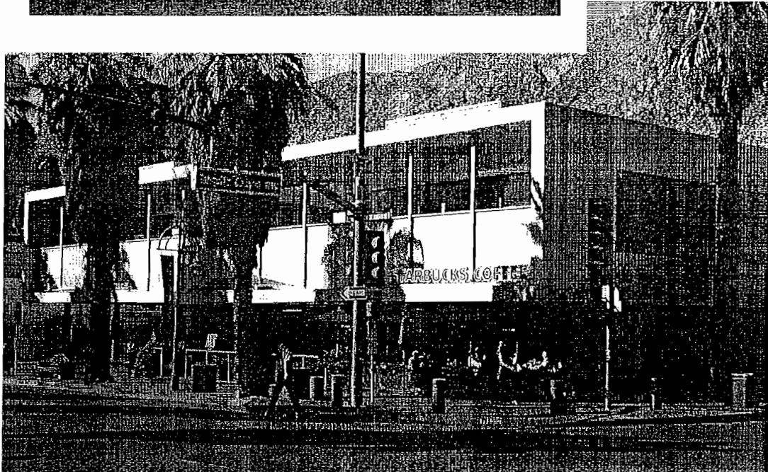
Figure 4 In this image, the Oasis Commercial Building is compared to Le Corbusier's 1929 Villa Savoye. Both buildings feature a "floating" white volume, supported on slender pilotis.
