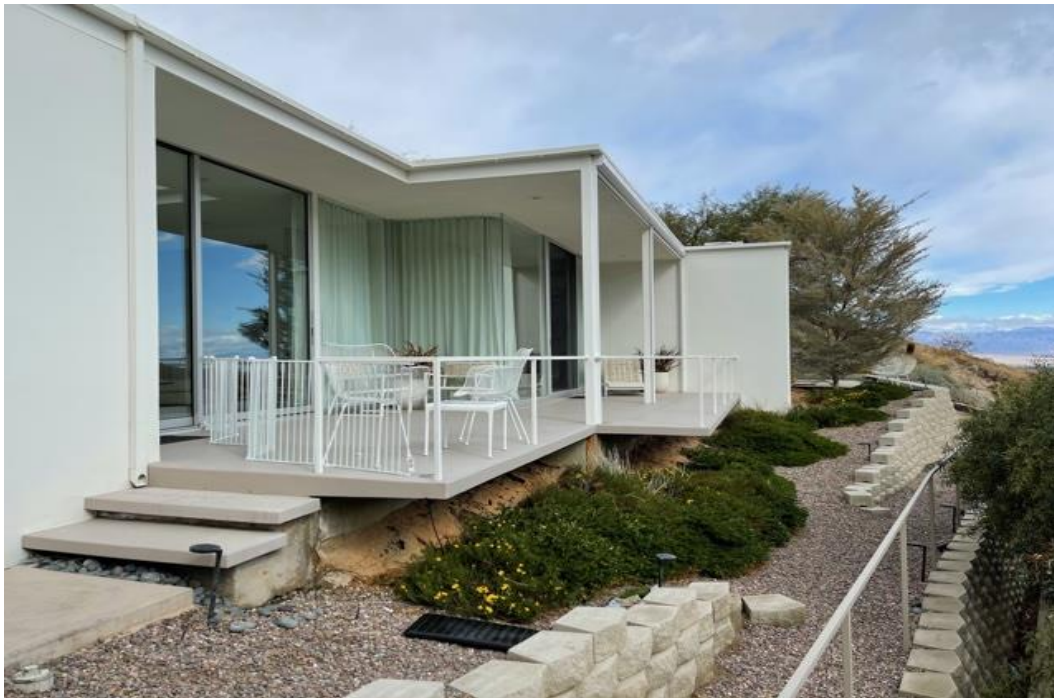
Image 15: Goldberg House. Southeast façade with exterior deck. [facing northeast] Photo Credit: Michael Johnston [January 2021]
