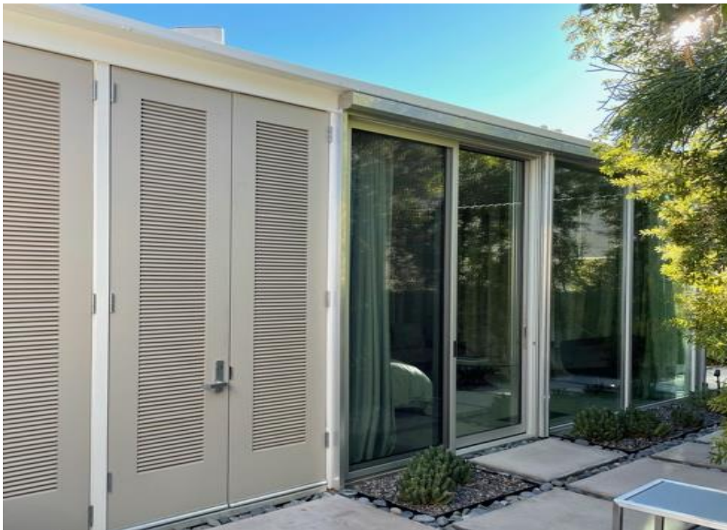
Image 19: Goldberg House. Southwest façade. Detail of replacement louvered doors [facing east]. Photo Credit: Michael Johnston [January 2021]
