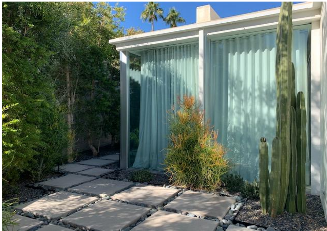
Image 17: Goldberg House. Southeast façade including addition to bedroom c. 1975 [facing northwest] Photo Credit: Michael Johnston [January 2021]
