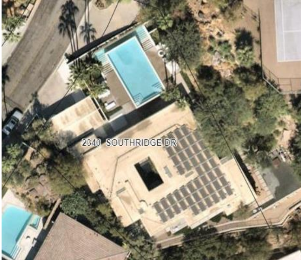
BELOW AN AERIAL VIEW OF THE RESIDENCE.
