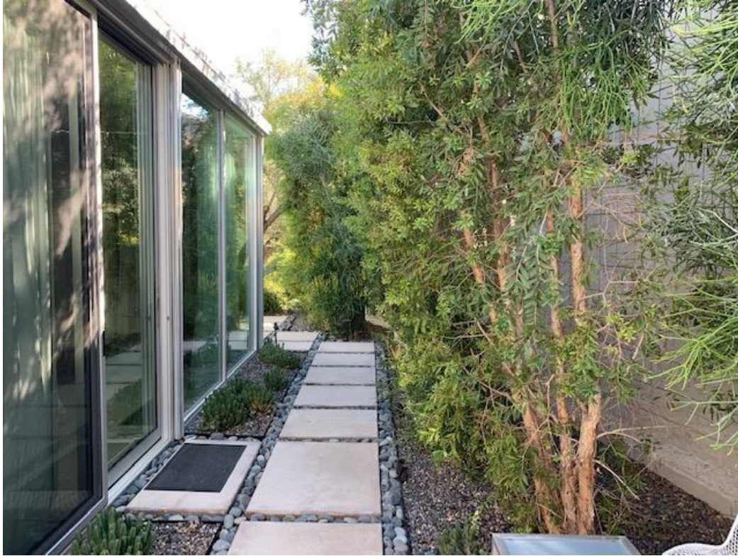
Image 18: Goldberg House. Southwest façade. Detail of bedroom addition [facing south]. Photo Credit: Michael Johnston [January 2021]
