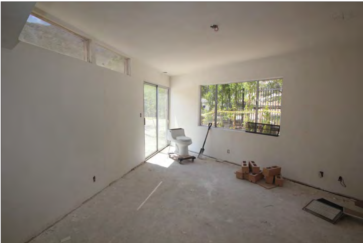
Image 59: Subject property, interior, room addition, view northwest (Chattel, 2021)
