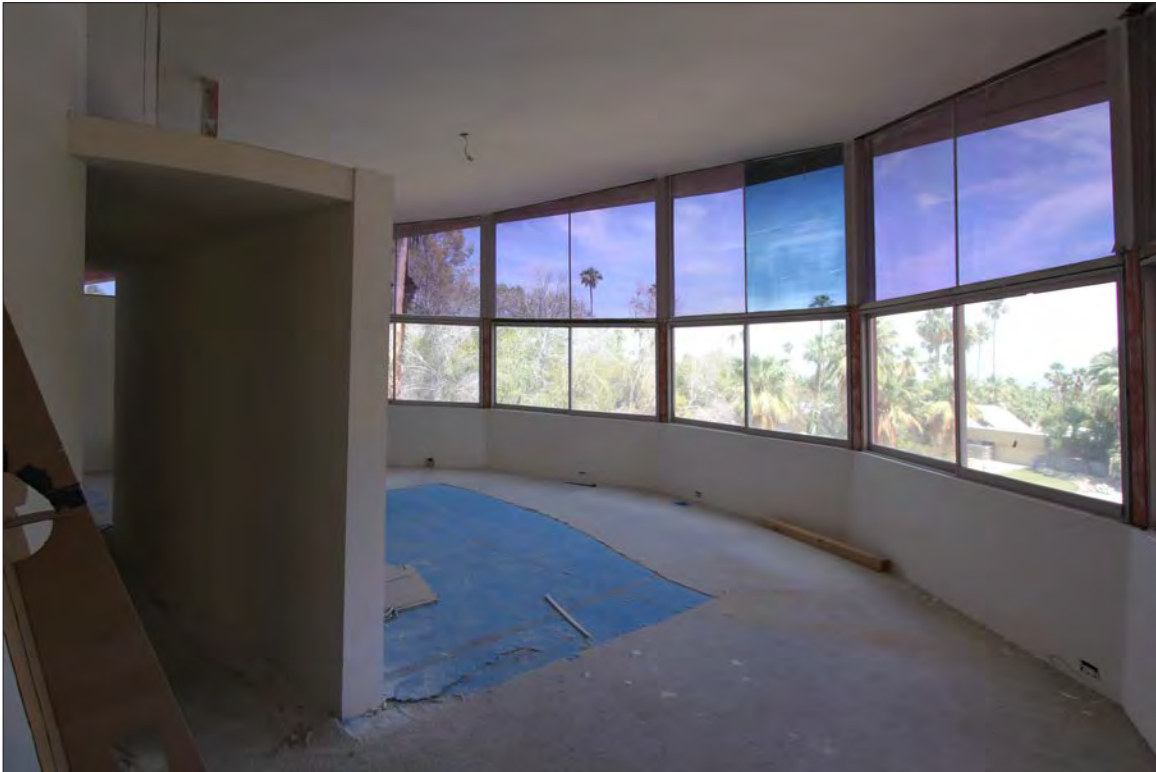
Image 70: Subject property, interior, master bedroom, view east, note added tint
