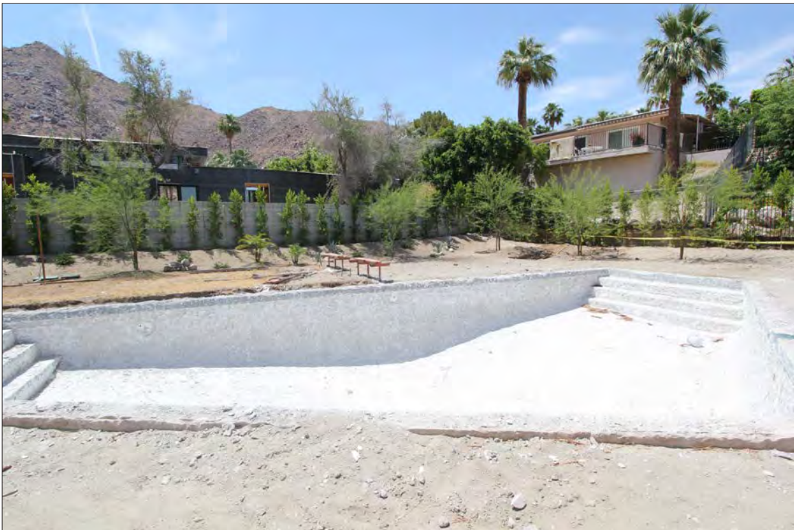
Image 30: Subject property, exterior, rear yard, detail of gunite swimming pool, view northwest (Chattel, 2021)
