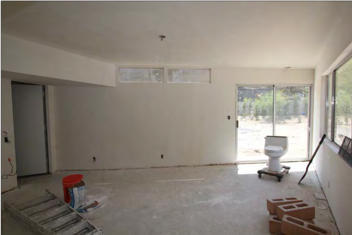
Image 58: Subject property, interior, room addition, view west (Chattel, 2021)
