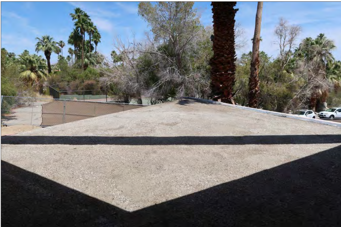
Image 45: Subject property, exterior, roof of carport, view east (Chattel, 2021)
