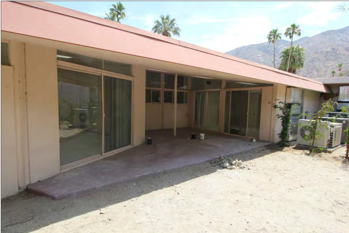
Image 19: Subject property, exterior, north elevation, inset patio, view south (Chattel, 2021)
