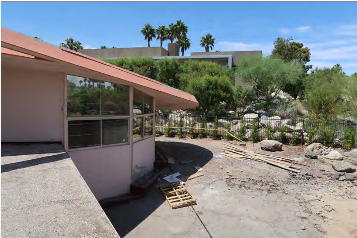
Image 43: Subject property, exterior, east elevation, view of side yard from roof of carport, view north (Chattel, 2021)
