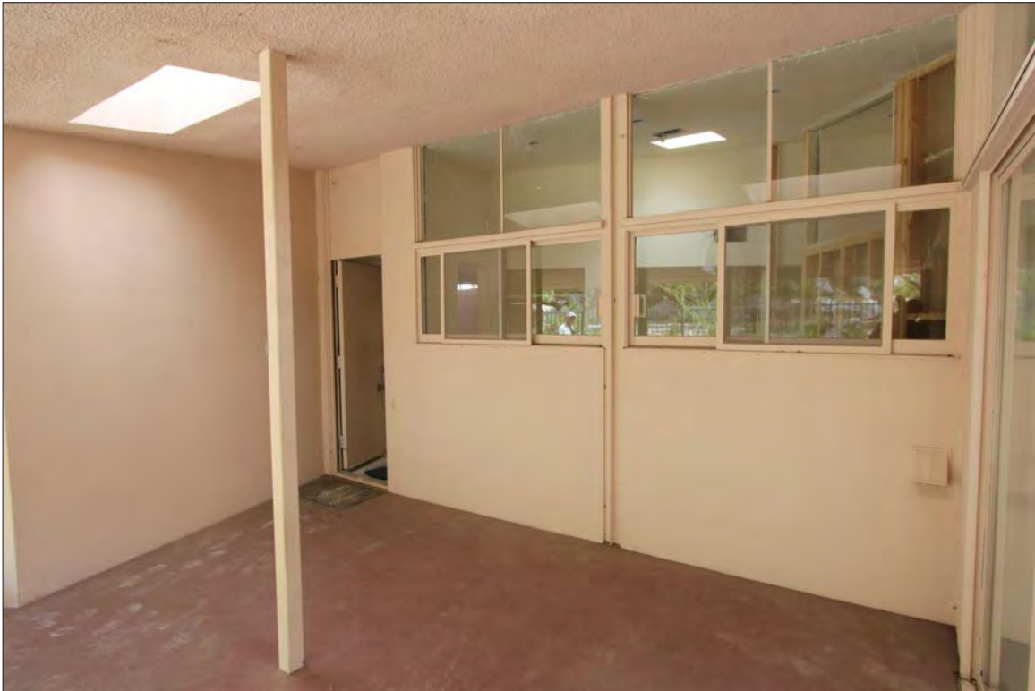
Image 23: Subject property, exterior, north elevation, inset patio, view south (Chattel, 2021)
