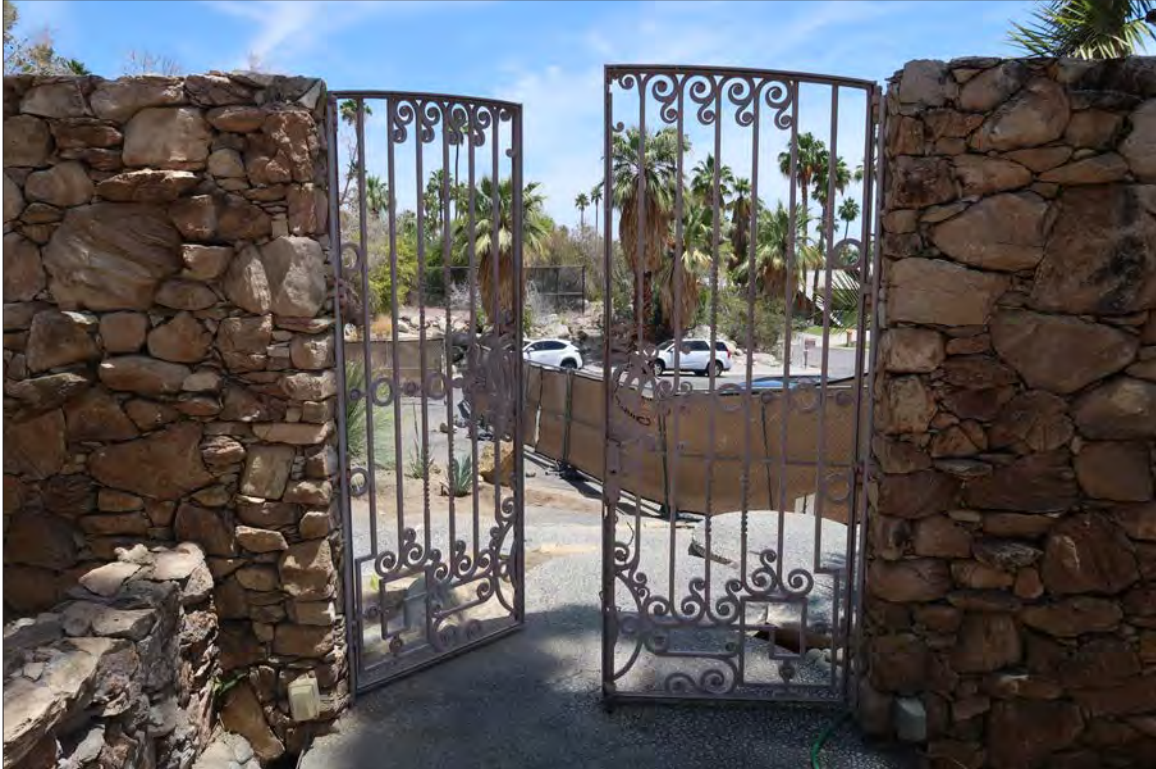
Image 8: Subject property, exterior, entrance courtyard gate, view southeast (Chattel, 2021)
