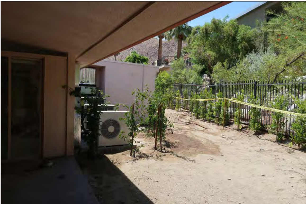
Image 22: Subject property, exterior, north elevation, inset patio and mechanical equipment, view west (Chattel, 2021)
