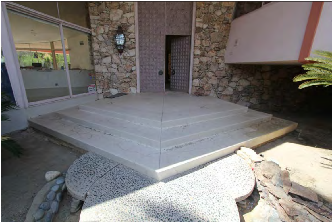
Image 11: Subject property, exterior, south elevation, pentagon-shaped, terrazzo-clad projecting stoop, view north (Chattel, 2021)
