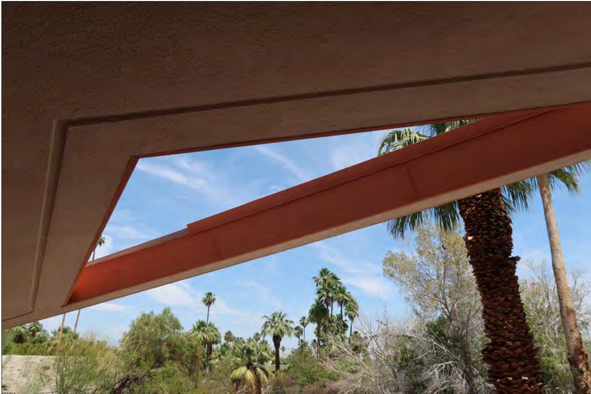
Image 46: Subject property, exterior, detail of triangular cutout at roof (Chattel, 2021)
