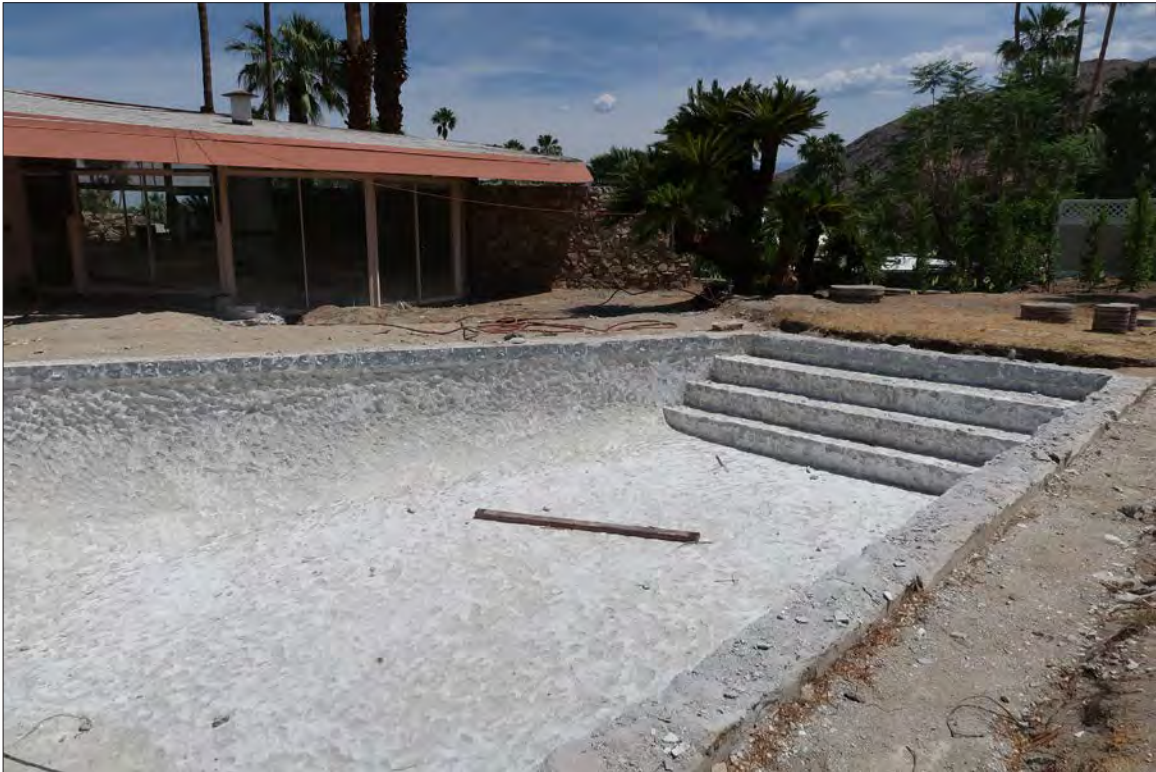
Image 31: Subject property, exterior, rear yard, detail of gunite swimming pool, view east (Chattel, 2021)
