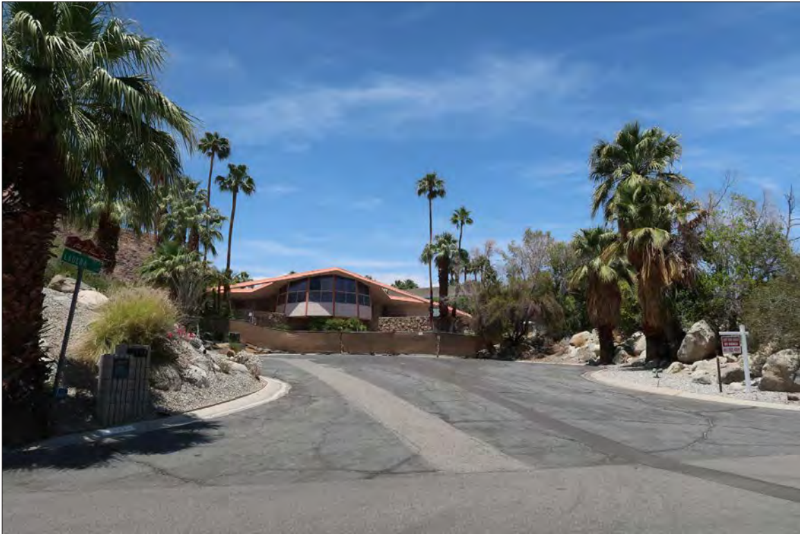
Image 1: Subject property, site context, residence and Ladera Circle from Abrigo Road and S. Via Las Palmas, view north (Chattel, 2021)
