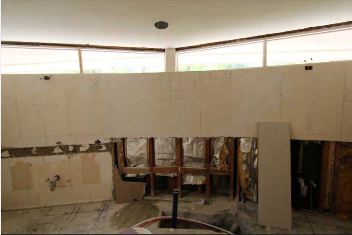
Image 63: Subject property, interior, bathroom, view north (Chattel, 2021)
