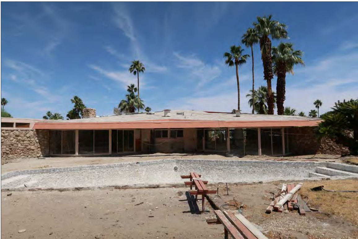
Image 26: Subject property, exterior, west elevation, rear yard, view southeast (Chattel, 2021)
