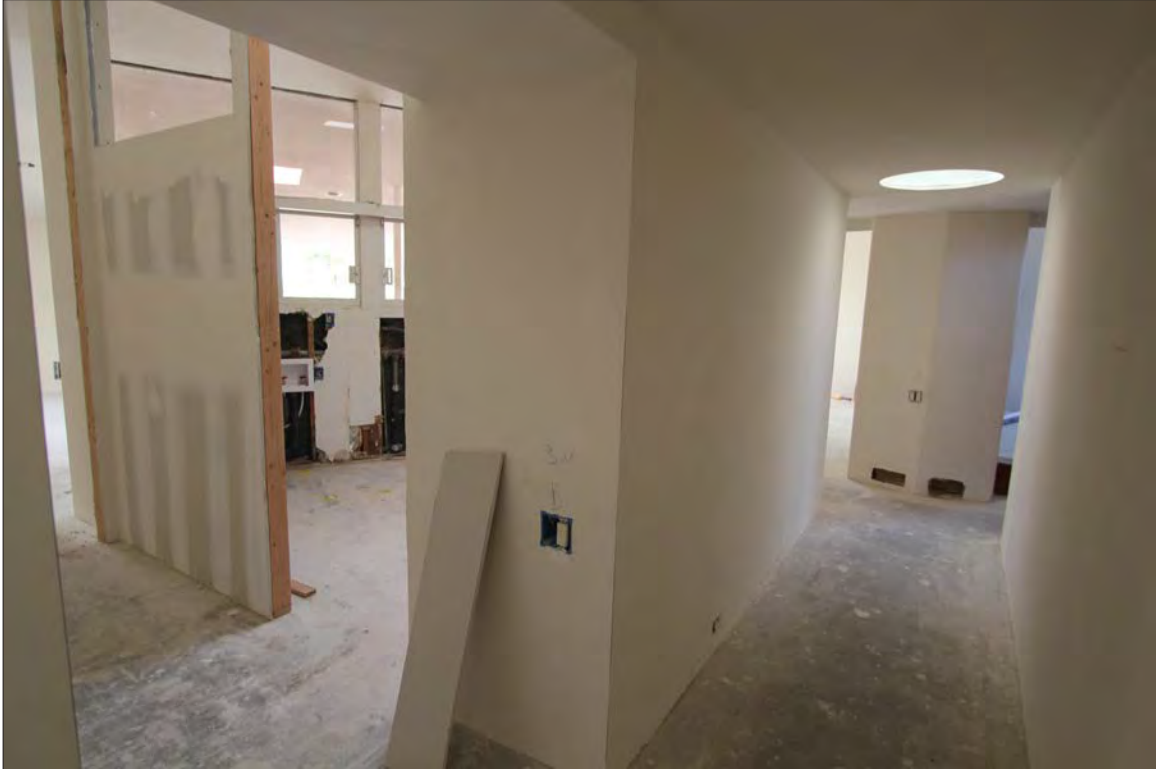
Image 60: Subject property, interior, hallway, view north (Chattel, 2021)
