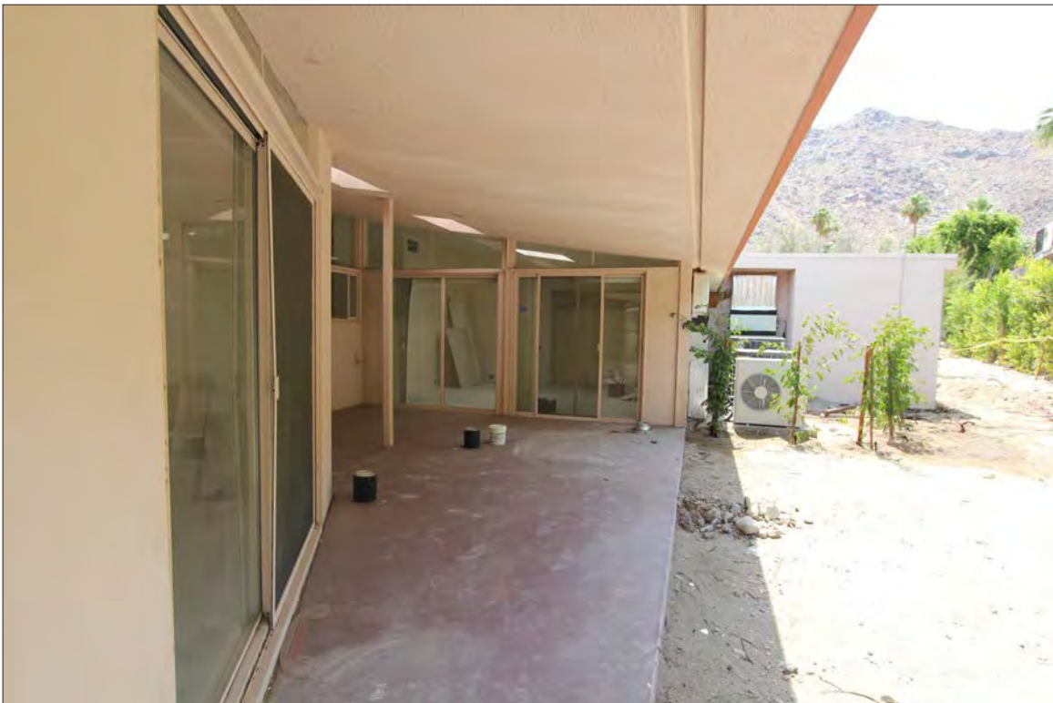
Image 20: Subject property, exterior, north elevation, inset patio, view west (Chattel, 2021)
