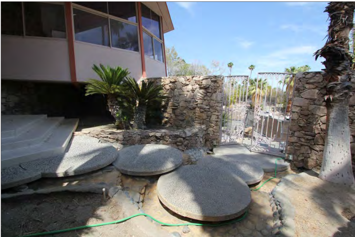
Image 9: Subject property, exterior, circular seeded aggregate steppingstones inside entrance courtyard, view east (Chattel, 2021)
