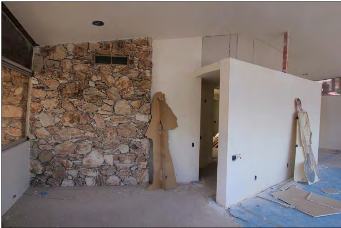
Image 69: Subject property, interior clad wall and privacy wall (Chattel, 2021)
