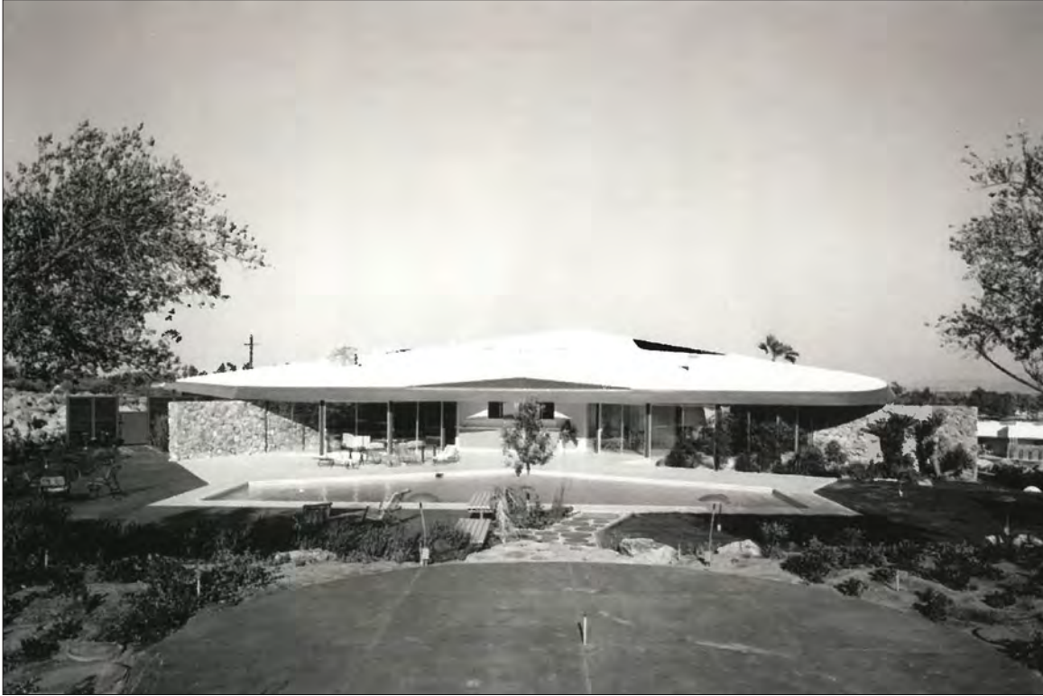
Image 14: Exterior, west elevation with swimming pool visible, view east (Gail B. Thompson, Willows Historic Palms Springs Inn, c. 1960s)
