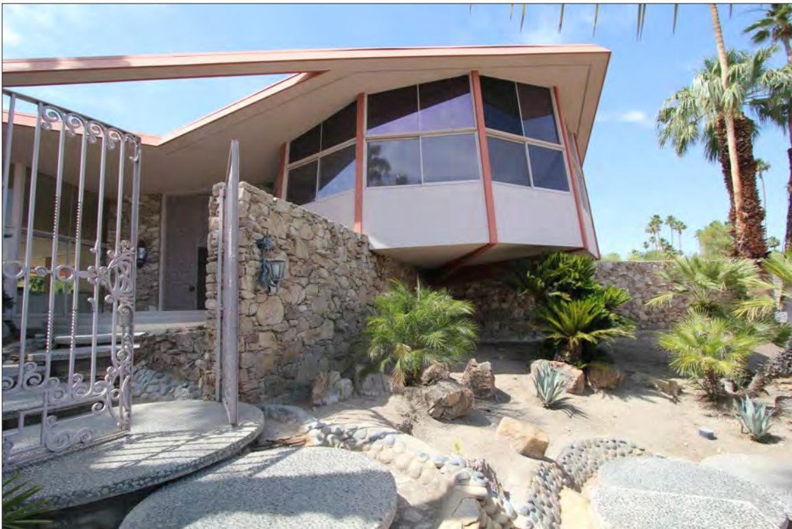
Image 4: Subject property, exterior, facade, note circular seeded aggregate steppingstones, view north (Chattel, 2021)
