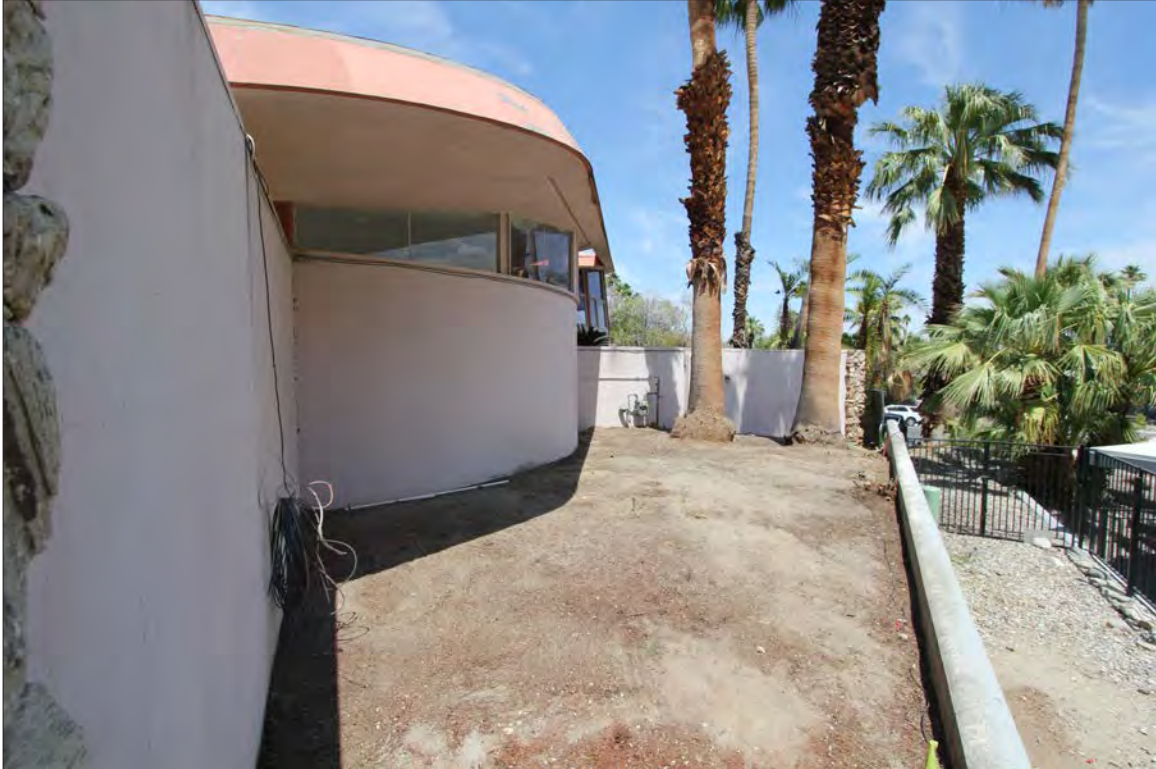
Image 40: Subject property, exterior, south elevation, view east (Chattel, 2021)
