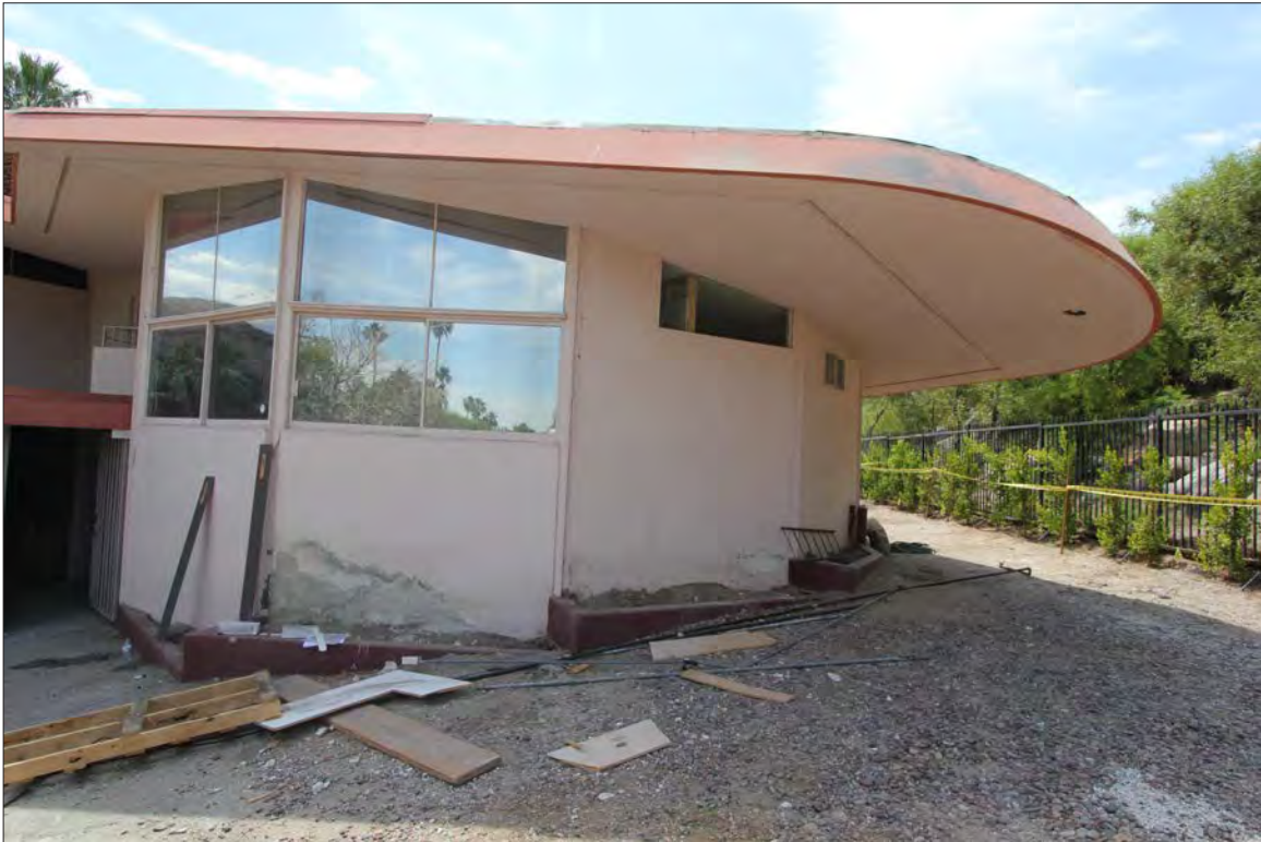
Image 17: Subject property, exterior, east elevation, view northwest (Chattel, 2021)
