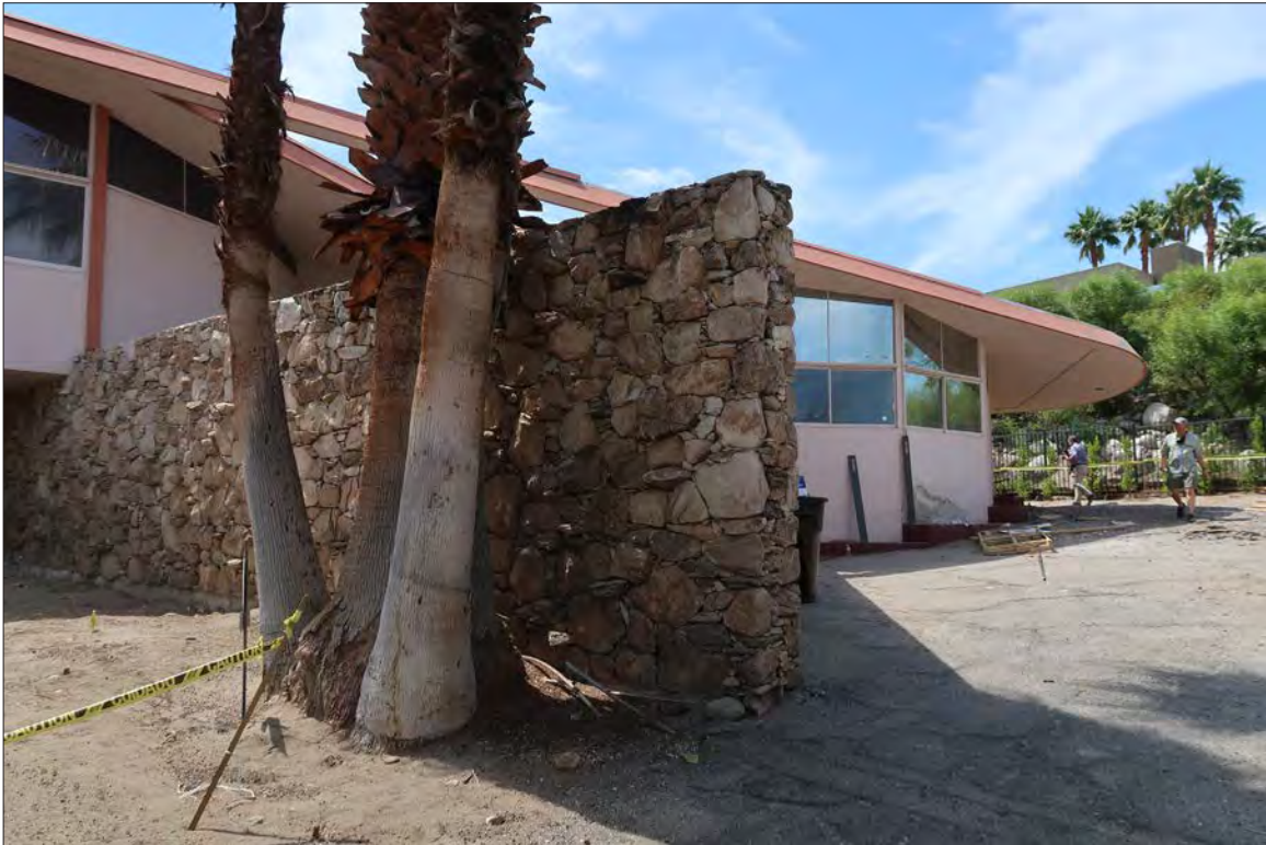
Image 15: Subject property, exterior elevation, view west (Chattel, 2021)
