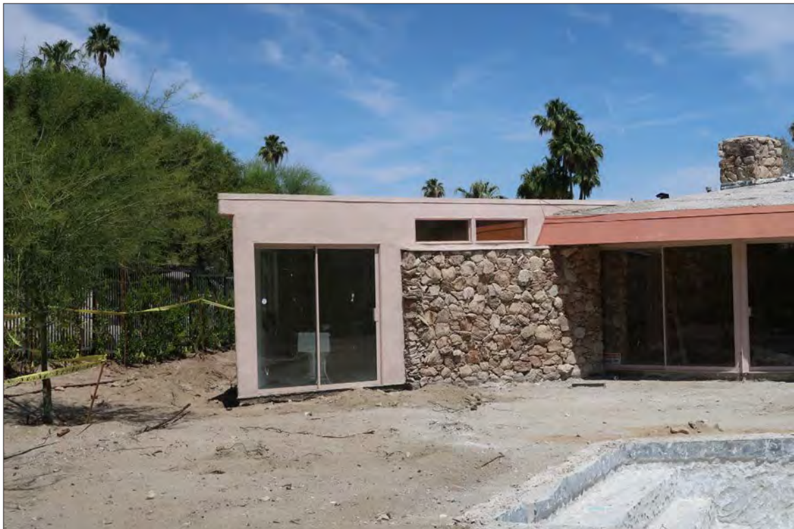
Image 33: Subject property, exterior, west elevation, room addition to north of
