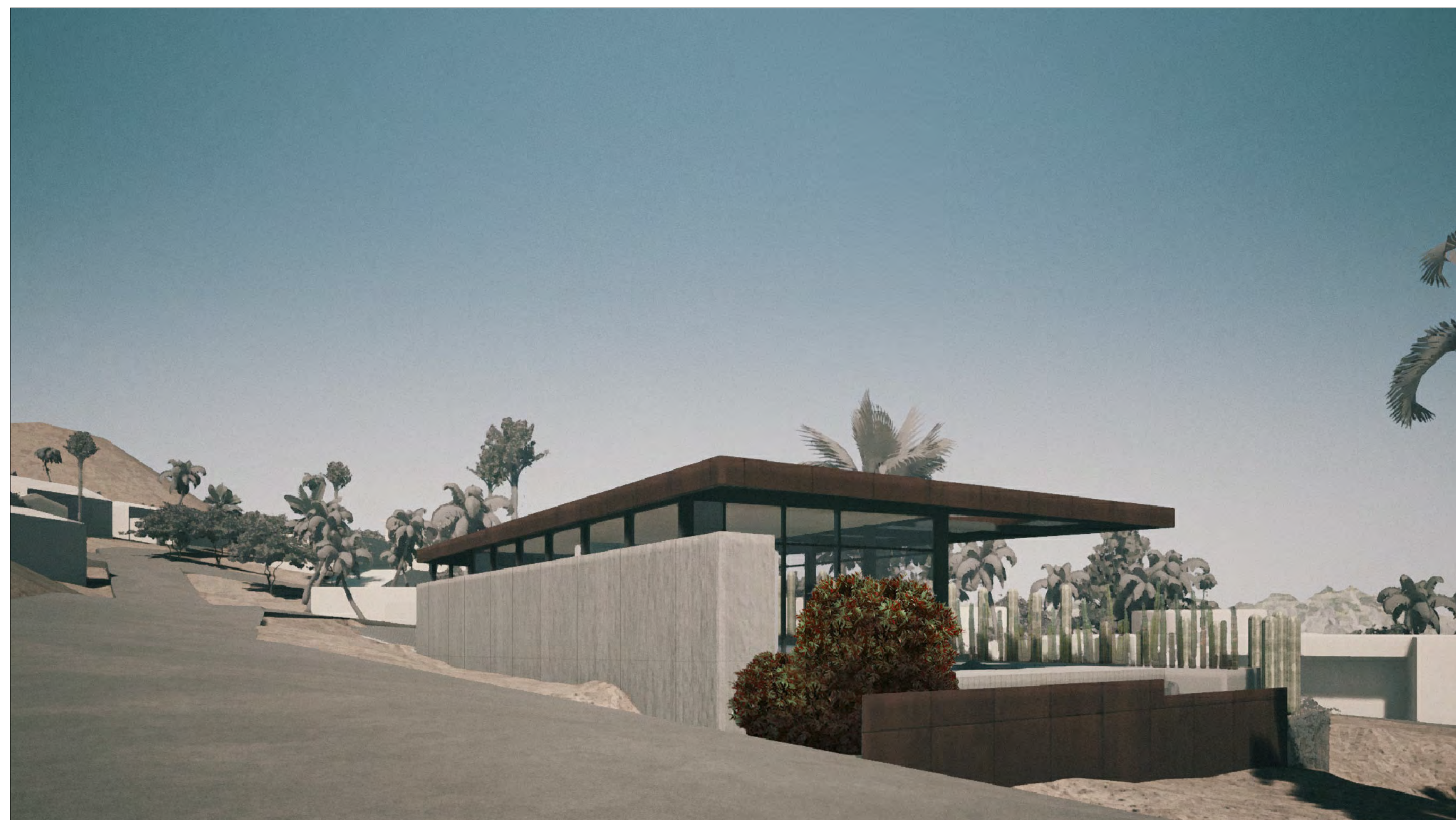
3 A801 LOOKING SOUTH-EAST
