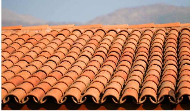
Roof – Spanish Tile
