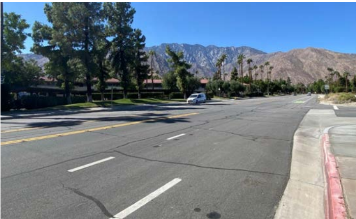
Construct a pedestrian crossing and median refuge at San Rafael Drive looking west at McCarthy Road
