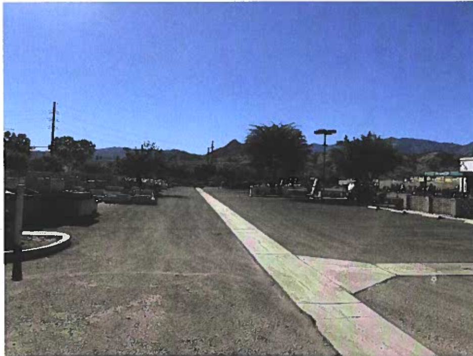
Photo #6 View of the concrete drainage channel along the eastern site boundary.
