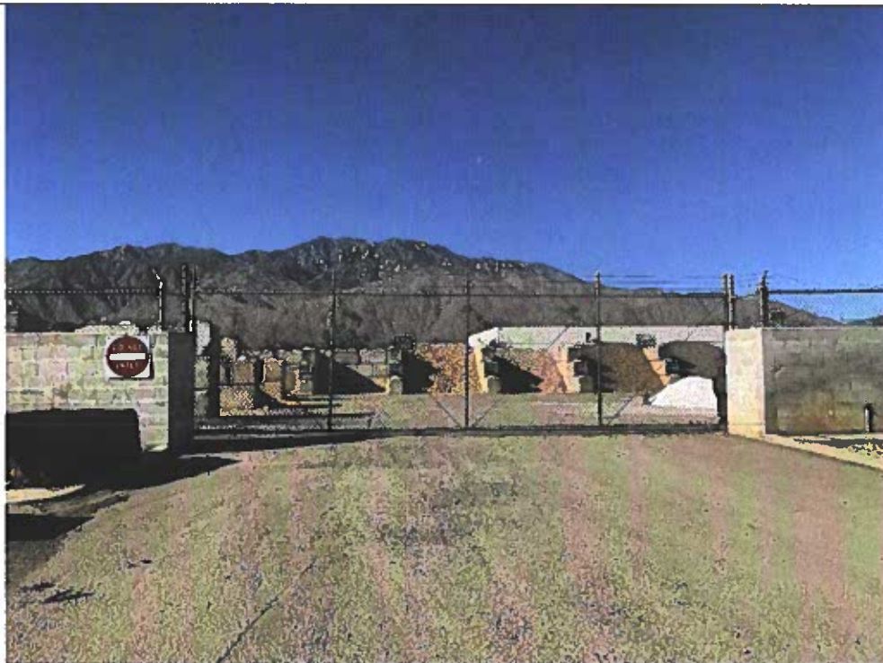
Photo #2 View of the locked portion of the Subject Property with segregated rock material for sale.
