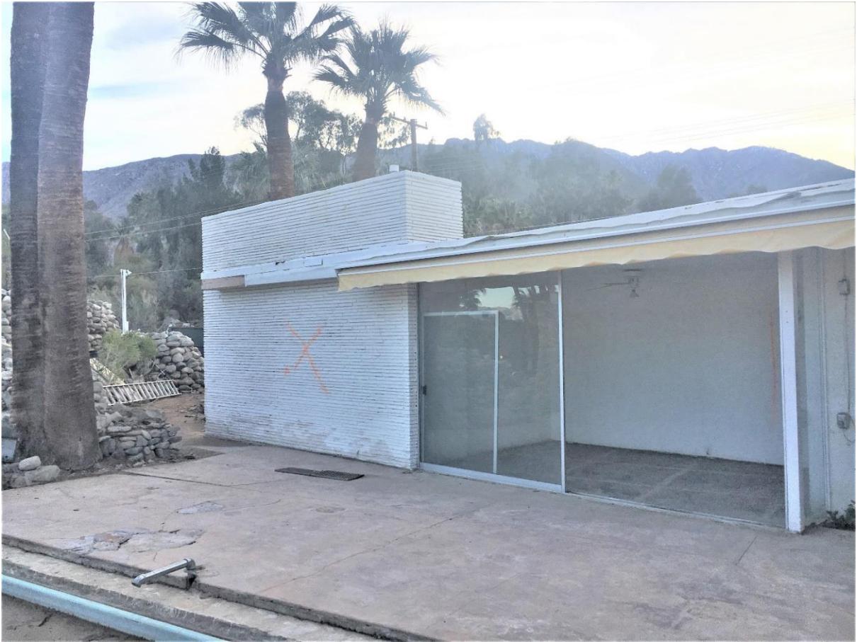
In this February 2019 photo, the original open dining patio had been enclosed with sliding glass doors. The louvered redwood ceiling had been covered with sheetrock, and a ceiling fan installed. Author's photo.
