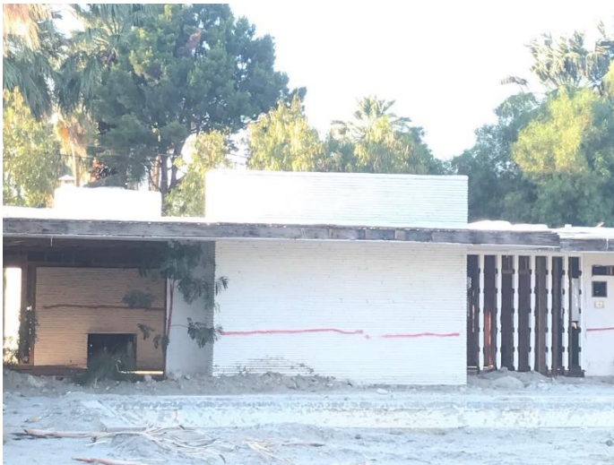
By the time Thomboy Properties bought the home, the horizontal muntins and obscure glass panes had been removed, leaving only the vertical supports. Photos taken July 9, 2019, as work was beginning on the restoration of the home. From left, Jackie Thomas, the author, and DeeAnn McCoy. Author's photos.
