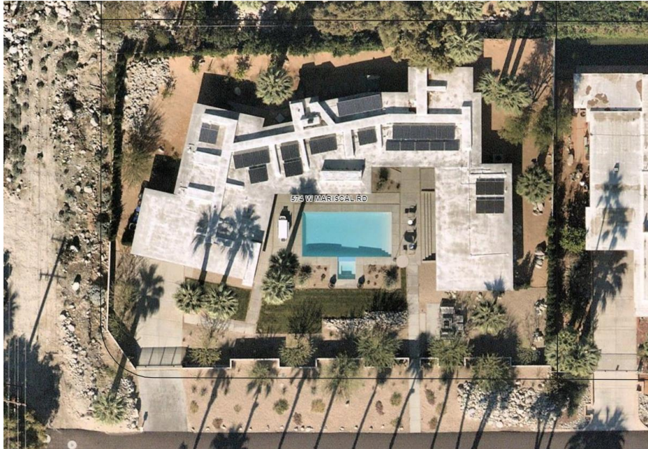
BELOW AN AERIAL VIEW OF THE RESIDENCE
