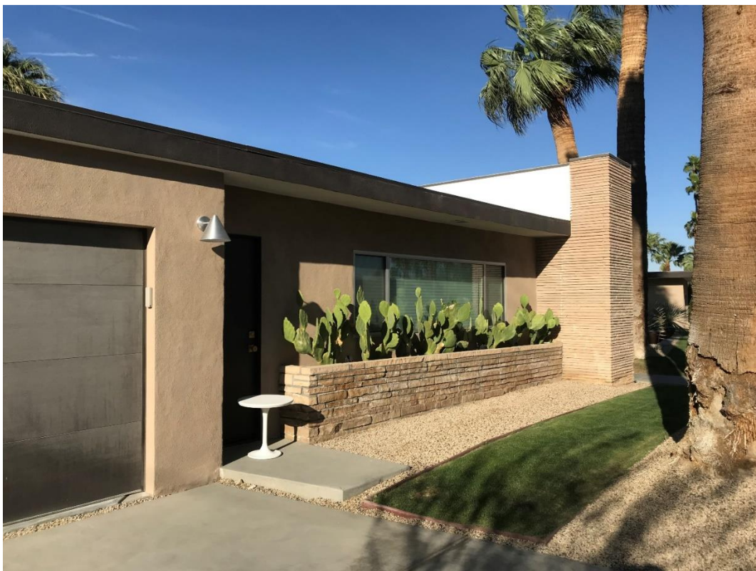
The restored sandstone planter. Author's photo.
