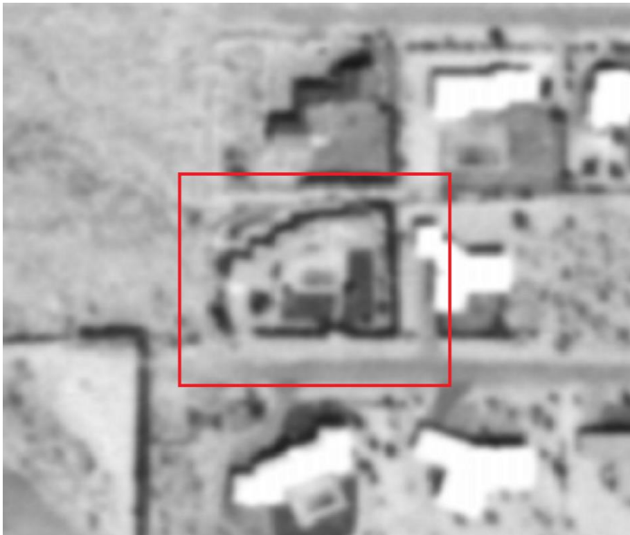
1953 aerial photograph, showing the 1952 bedroom addition to the left of the garage.
