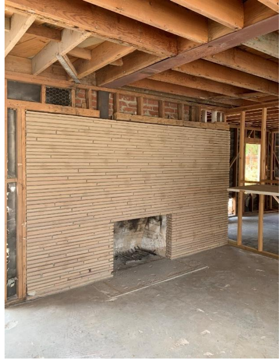
Left: In February 2019 photo, Herbert Burns' signature floating soffits had been removed from the interiors of the home. Author's photo.
