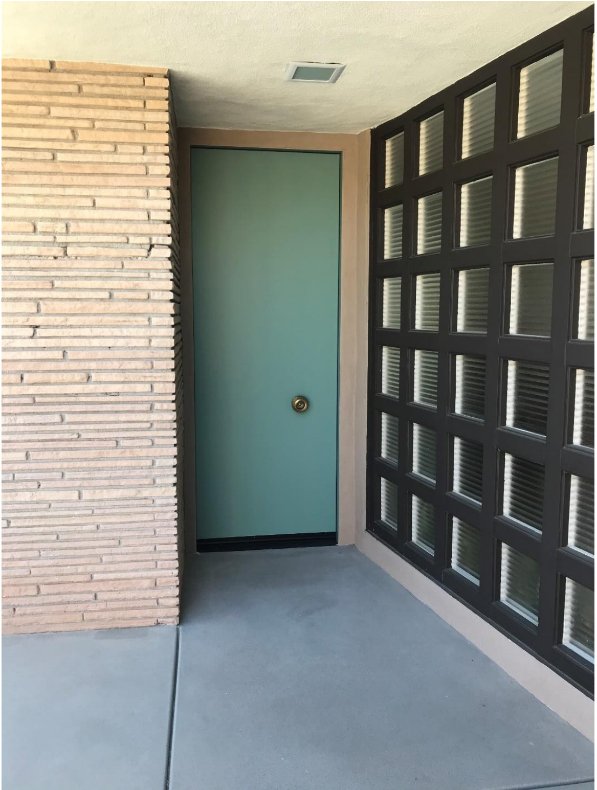
The historic turquoise paint color chosen by Burns for the front door was restored. Exterior paint colors are based on the two-toned tan and brown palette originally used. Photo courtesy Lance Gerber.
