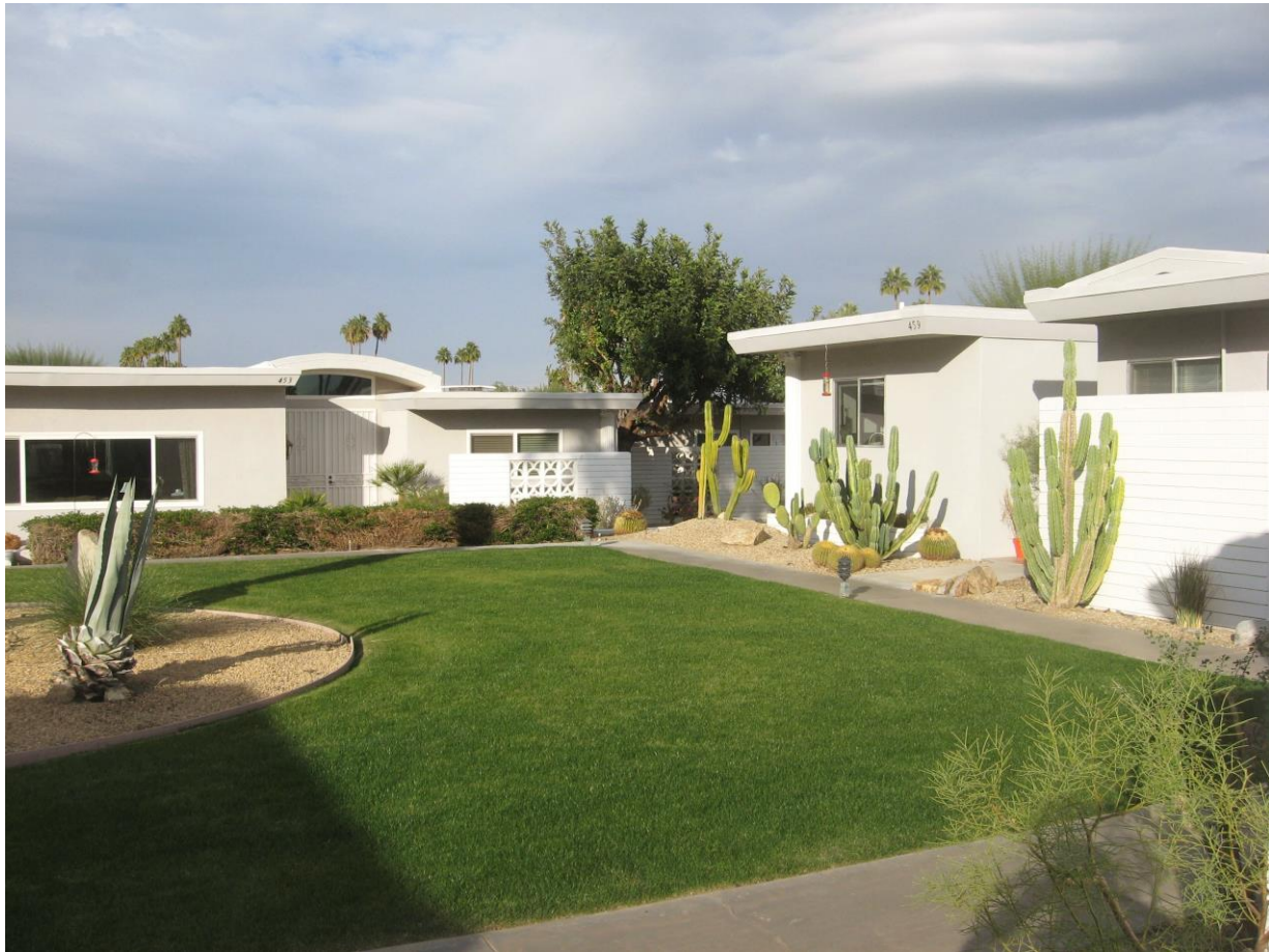
Typical Villa Roma court arrangement. Note rooflines and differences in entry roofs. (Author Photo. December 2020)
