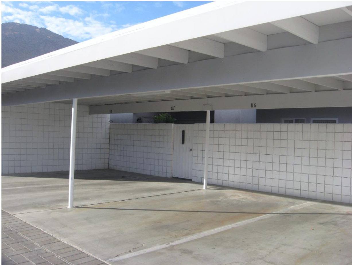
Example of a Villa Roma carport. Note treatment of patio walls and carport roof details. Pavers visible in lower-left were added in 2016, replacing original asphalt. (Author Photo. December 2020)
