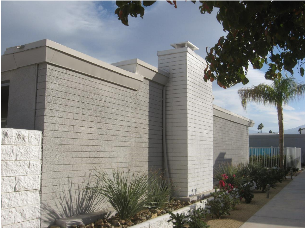
View demonstrating how Schuler used concrete block to achieve different visual effects. (Author Photo. December 2020)
