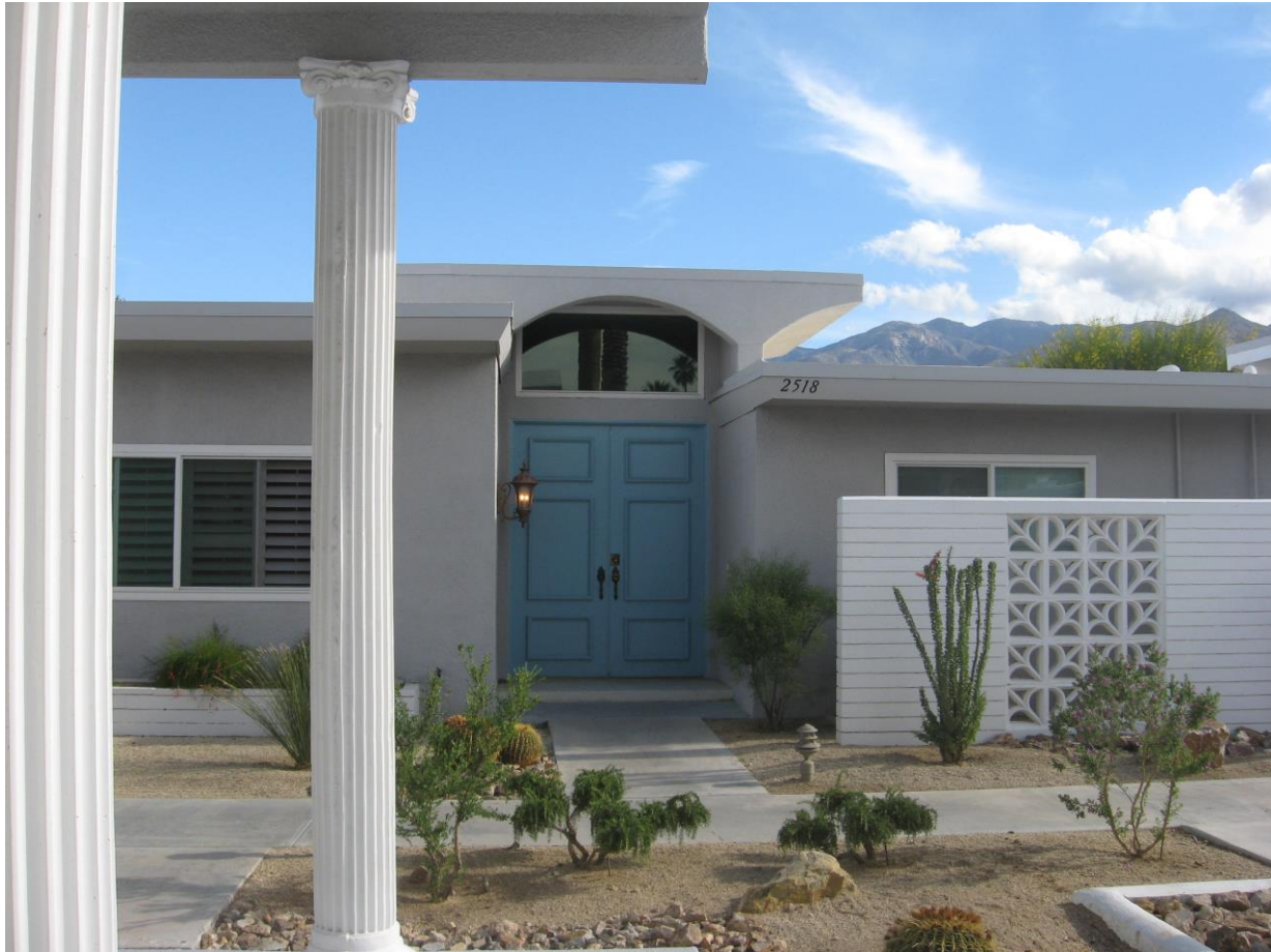
Villa Roma unit showing raised “platform” style of roof above entry. Note eaves, variegated roof heights, recessed entry, clerestory windows, carriage entry light and “Sprite” screen block wall, all typical original design features. Windows are vinyl-type replacements. (Author Photo. April 2021)
