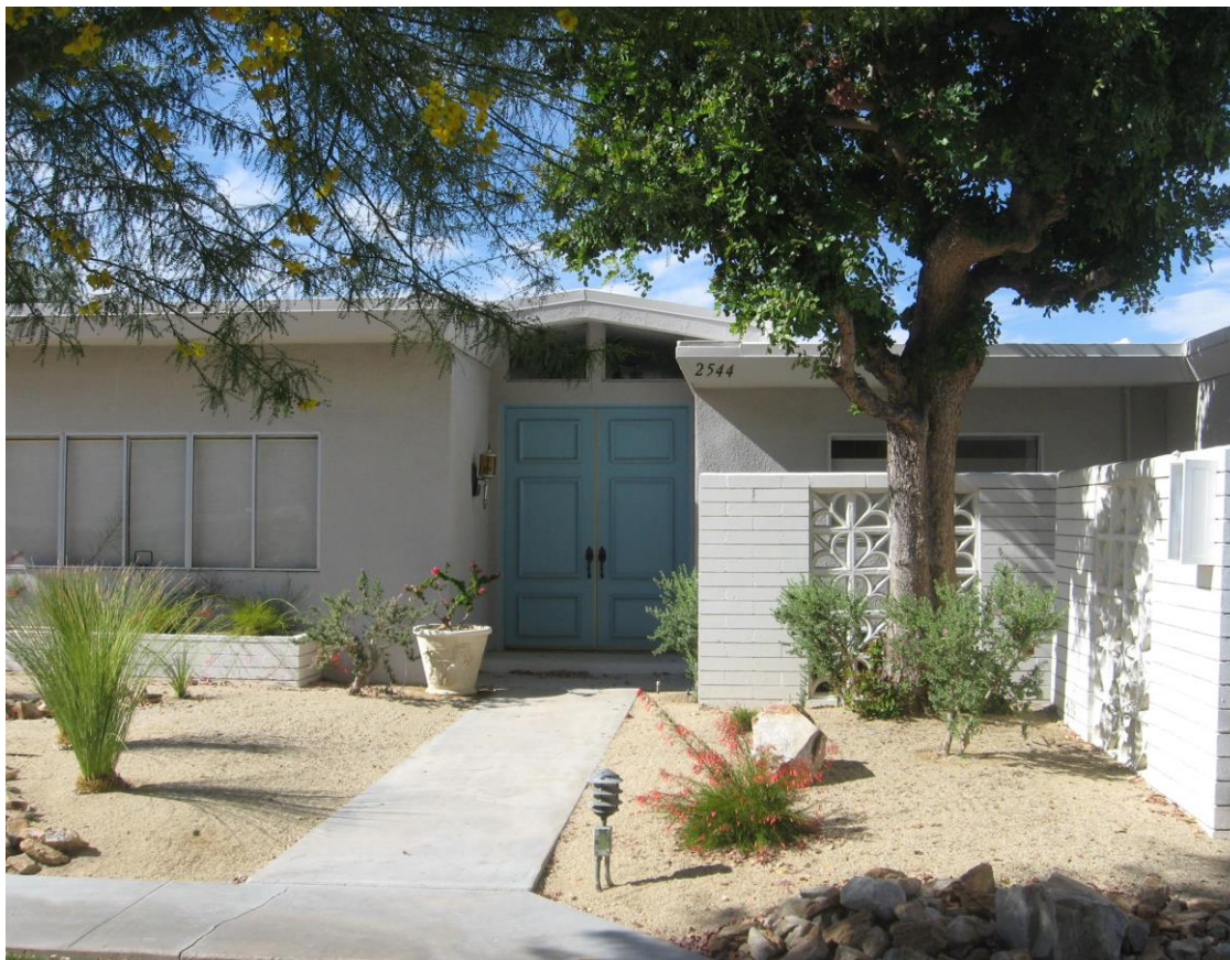
A typical Villa Roma unit showing original windows, double door, and light fixture. Note the variation in roof height, one of a number of ways Schuler minimized a box-like appearance. (Author photo. December 2020)
