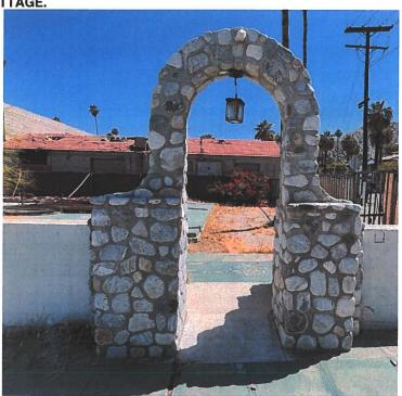
BELOW: OBSERVE THE STONEWORK OF THE ARCH IS BUILT OVER THE TOP OF AN ADJACENT STANDARD CONCRETE MASONRY BLOCK WALL WHICH DOES NOT APPEAR TO BE FROM THE 1915 PERIOD ASSOCIATED WITH THE COTTAGE'S CONSTRUCTION (REMNANT FLOORBOARDS SEEN BEYOND).
