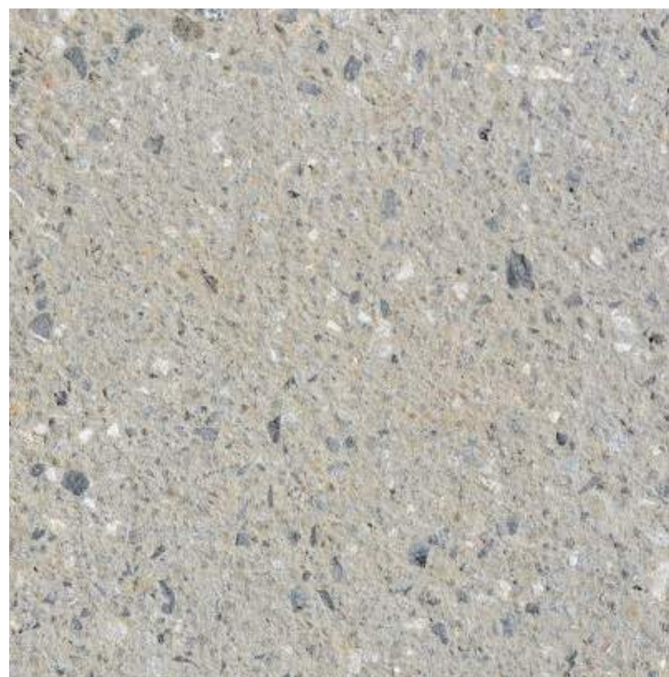
CAST-IN-PLACE CONCRETE WITH EXPOSED AGGREGATE DRIVEWAY
