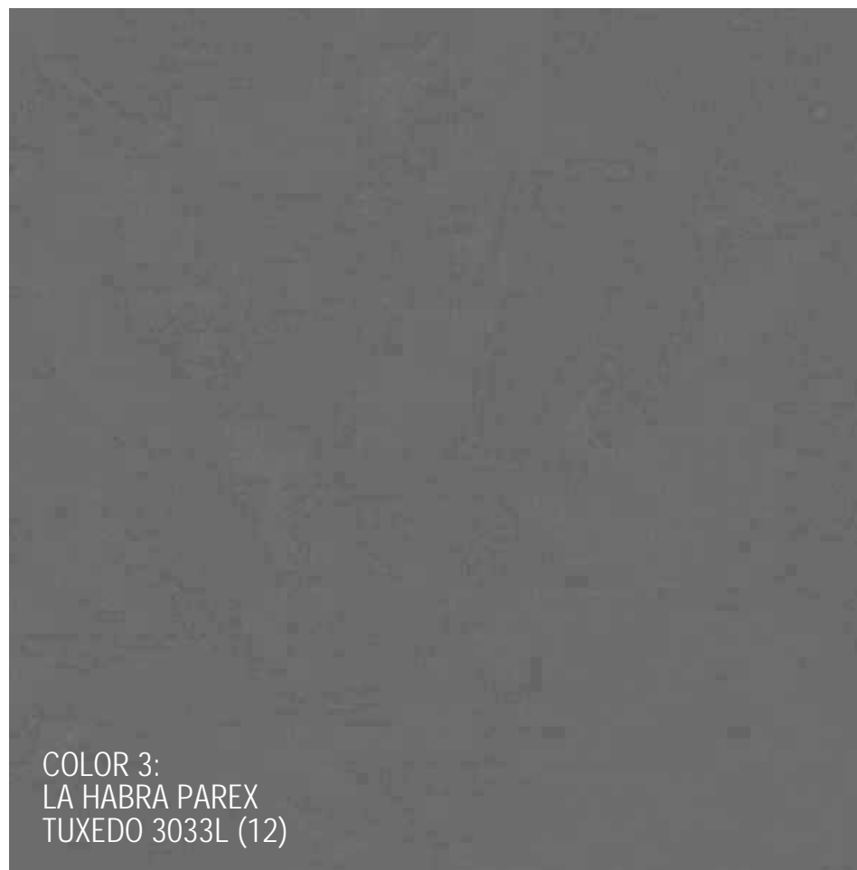
SMOOTH TROWELED PLASTER ENTRY ACCENT WALL
