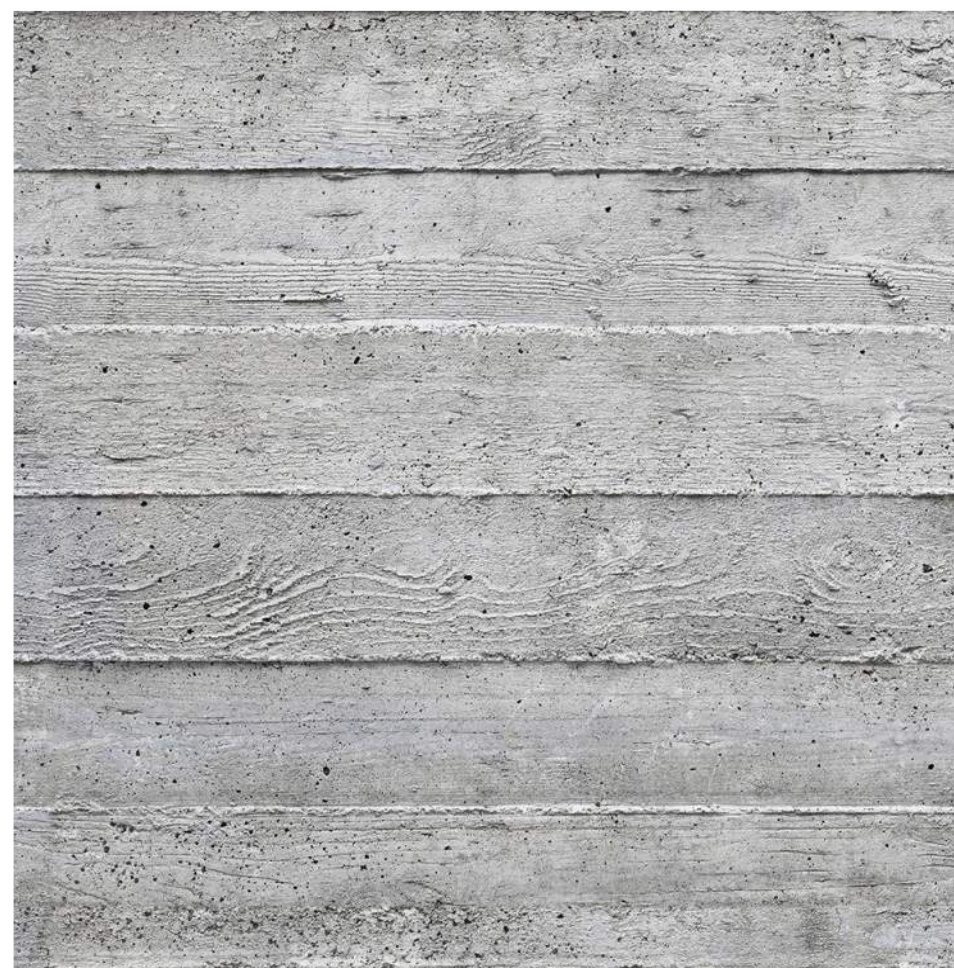
BOARD FORM CONCRETE POOL WALL
