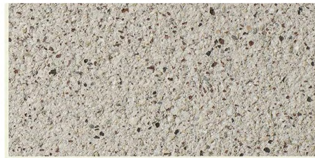
01. PERIMETER WALLS , ANGELUS BLOCK, COLOR NATURAL GRAY SHOTBLAST W/ 446 SPEC MIX MORTAR.
