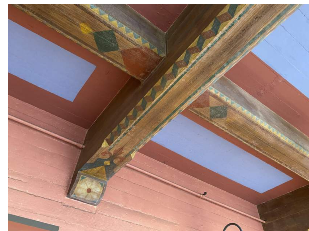
4 OUTER LOBBY CLG & BEAM
