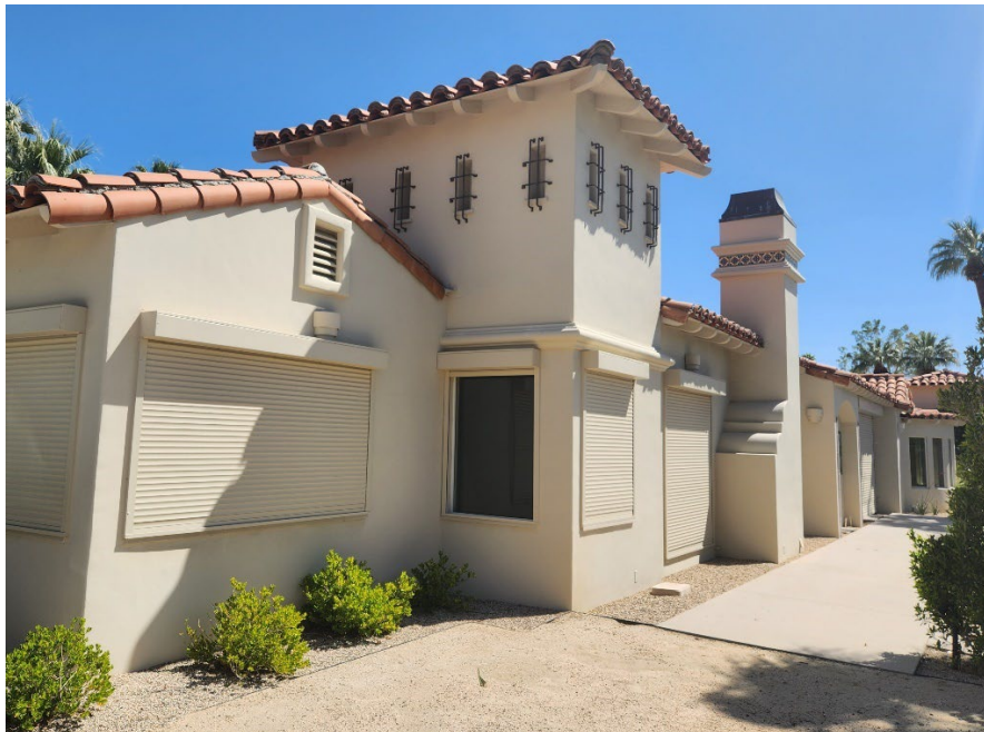
IMAGE OF THE SOUTH ELEVATION LOOKING EAST.
