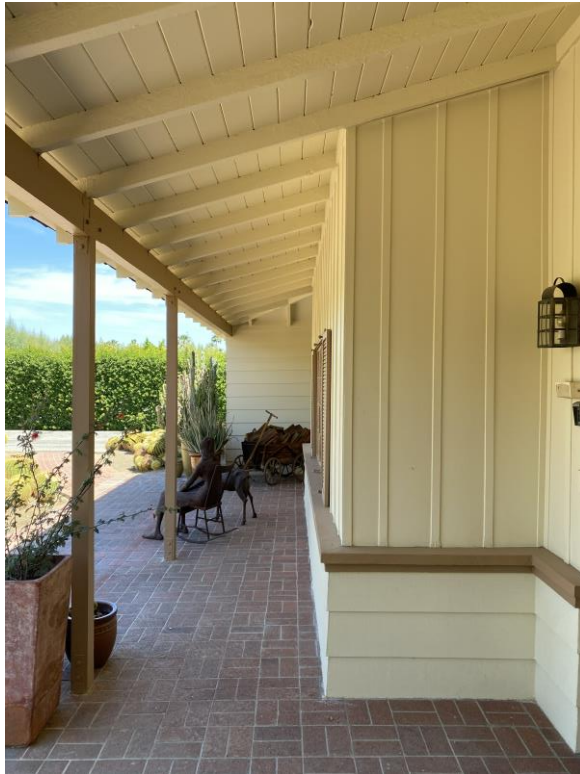
Photo 3. Looking north along porch. Note board-and-batten sheathing. (Thomas Morbitzer Photo. April 2021)
