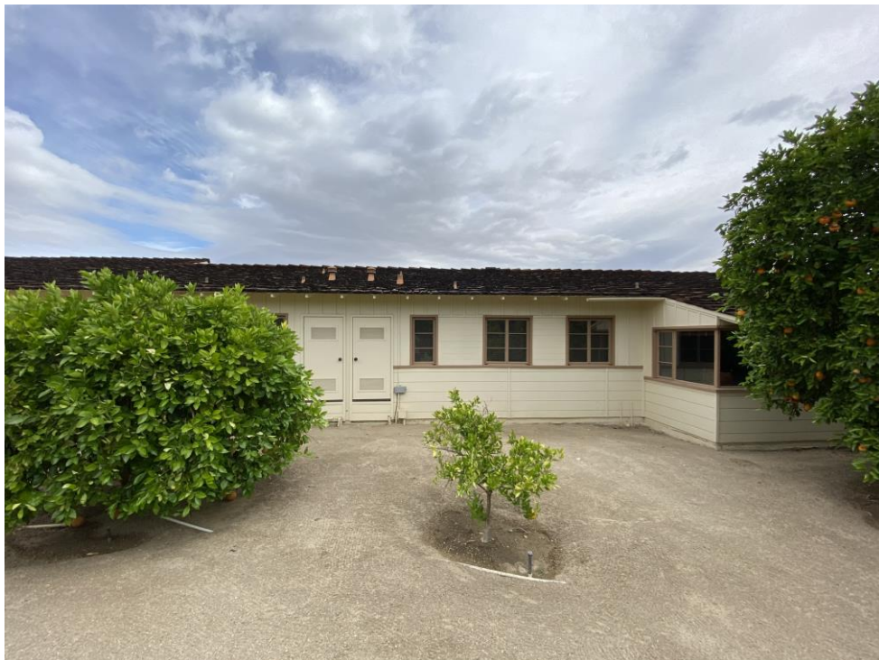
Photo 12. View of south wing facing north. (Thomas Morbitzer Photo. April 2021)
