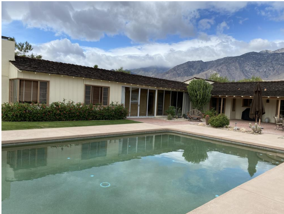
Photo 10. Looking across pool to southern wing. Note glass doors where outdoor patio was enclosed by Albert Frey (Thomas Morbitzer Photo. April 2021)
