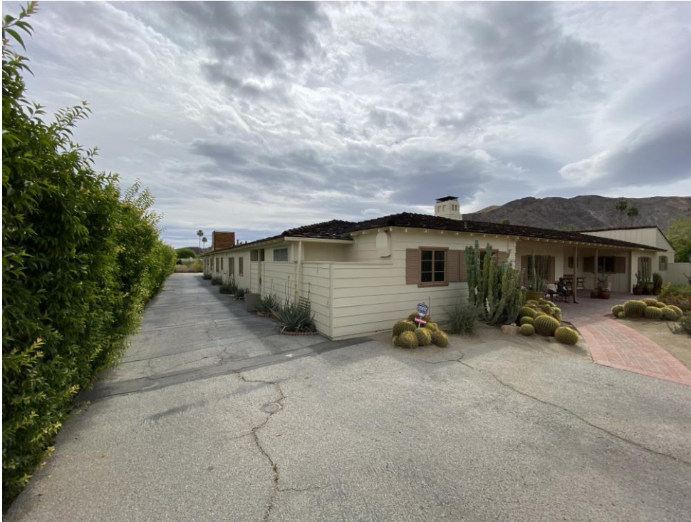
Photo 5. View on southeast looking up north wing towards garage. (Thomas Morbitzer Photo. April 2021)
