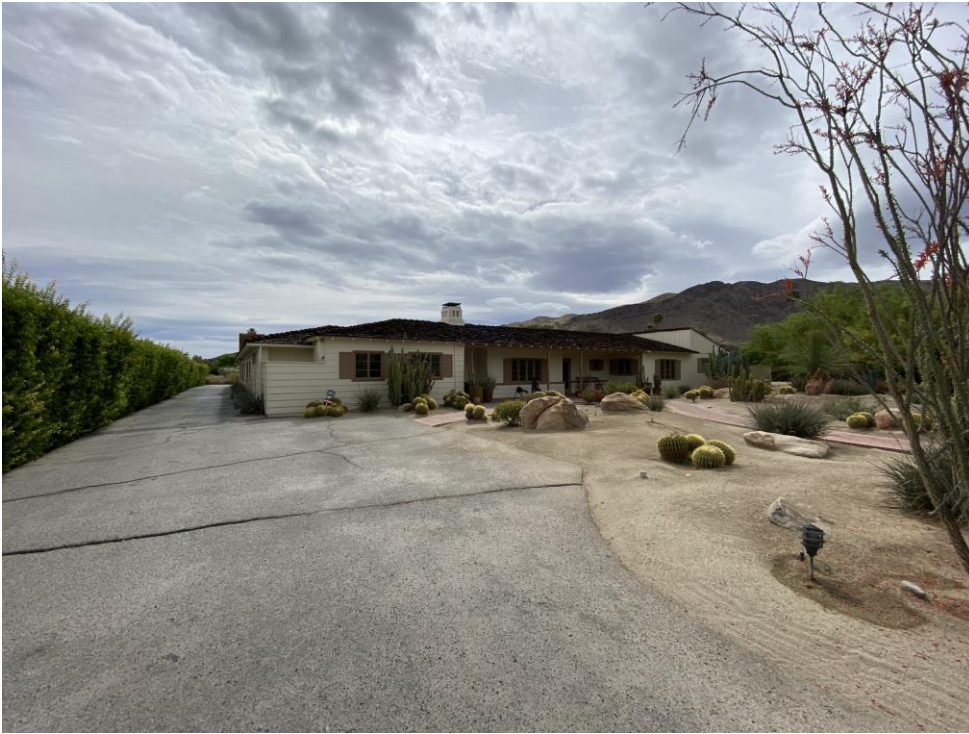
Photo 1. General view as seen from street looking east towards western façade. (Thomas Morbitzer Photo. April 2021)
