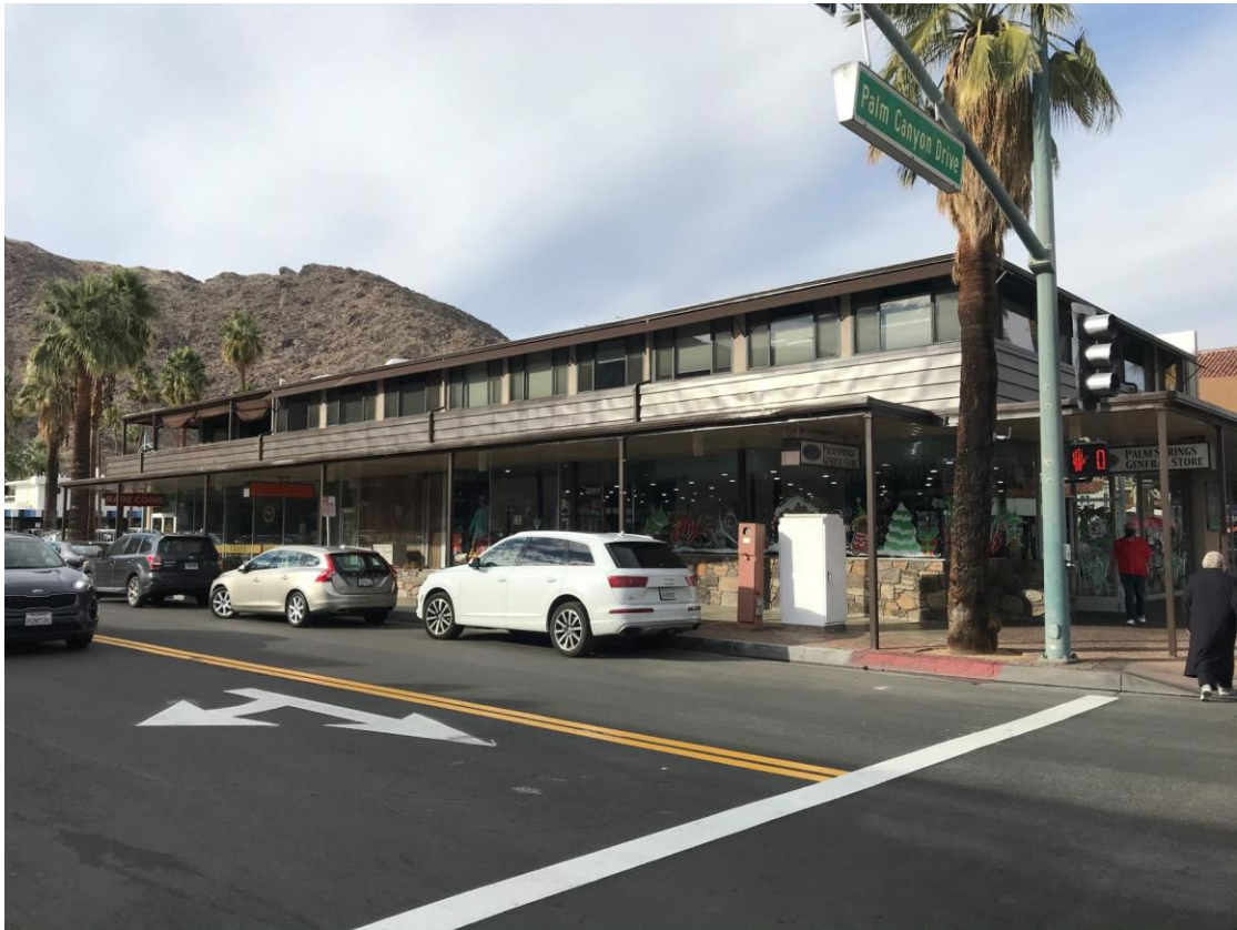
The southeast corner of the Atikian Building, showing the Arenas Road elevation.
