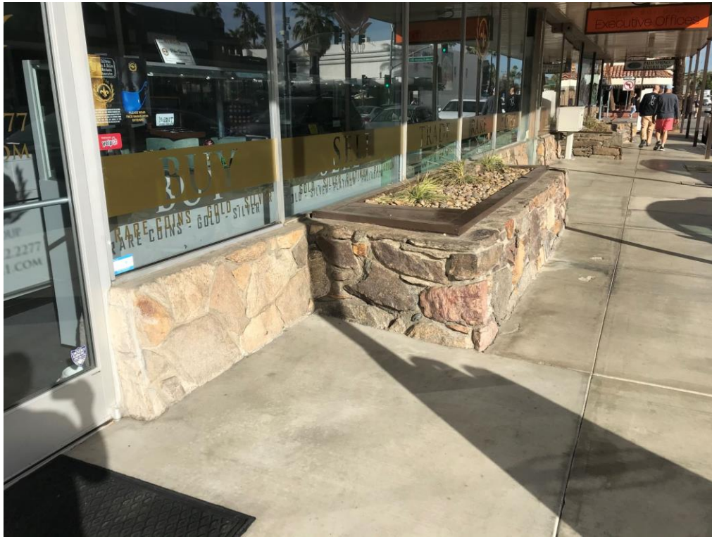
This smaller stone planter on Arenas Road was originally between two stores which had angled sawtooth configuration for interest. Those have been replaced by a straight line, with matching stone bases.
