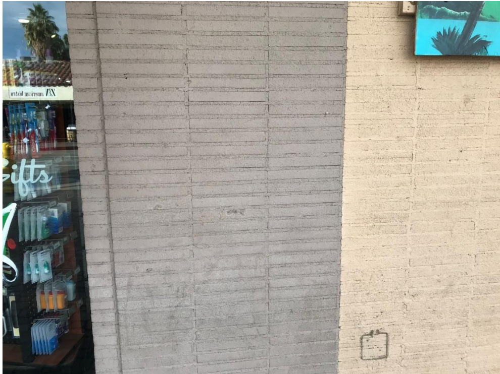
On the Palm Canyon Drive façade, Cody deliberately matched the existing Roman brick on the adjacent building, in size and application, creating a seamless transition.
