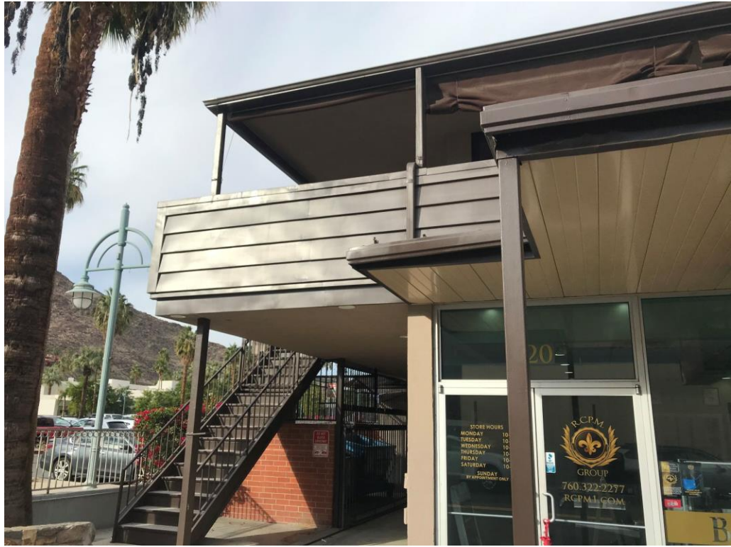
The new stair to the Atikian apartment's balcony.
