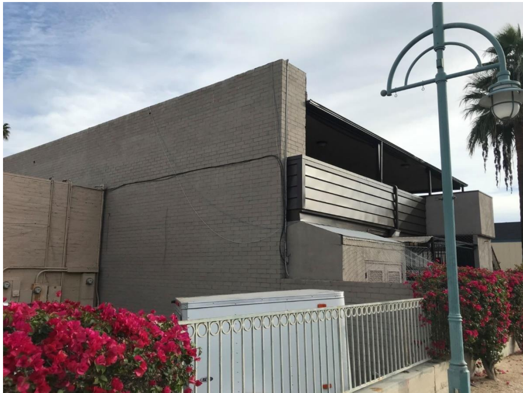
From the adjacent parking lot, a view of the back (north) side of the building shows the regular brick construction (vs. the Roman brick selected for the Palm Canyon façade).
