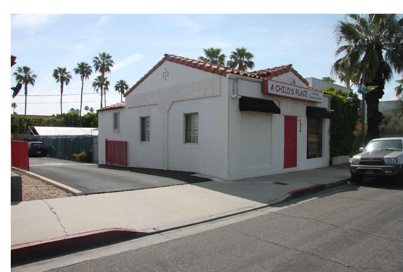
VIEW OF BLDG NORTHWEST CORNER
