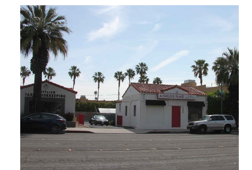
VIEW OF BUILDING WEST FACE
