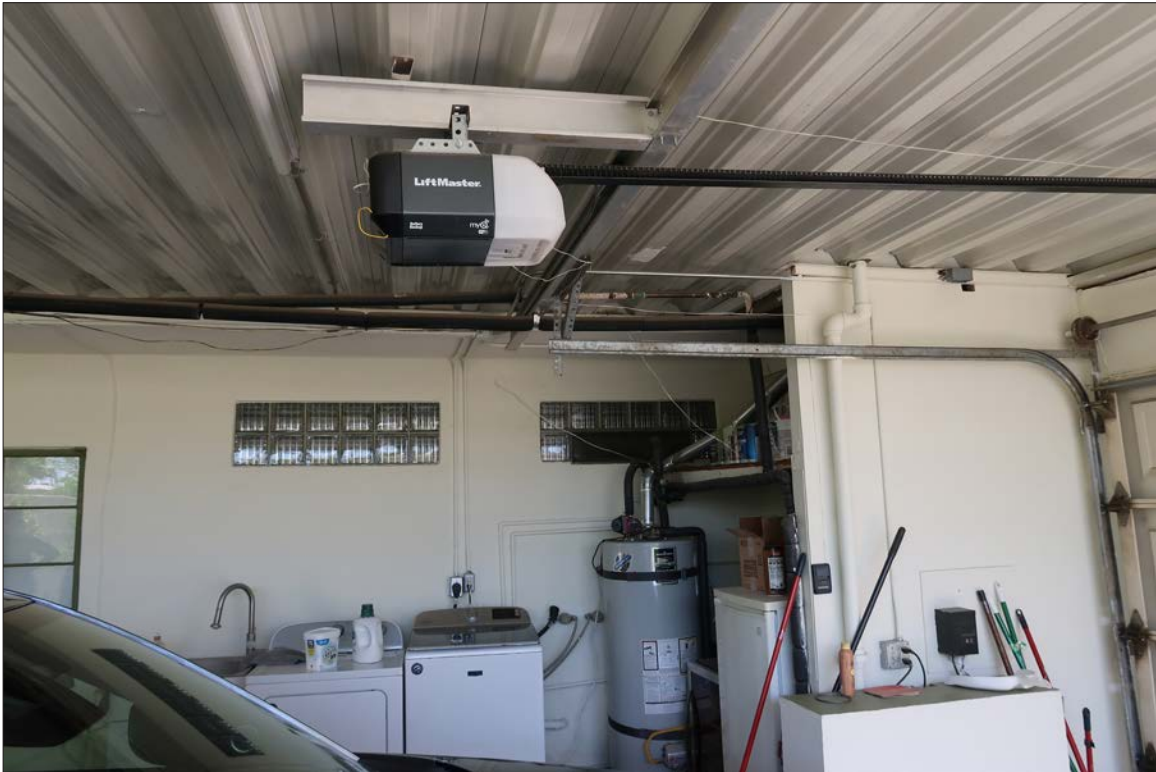
Image 55: Glass block windows at east elevation of residence, view west (Chattel, 2024)
