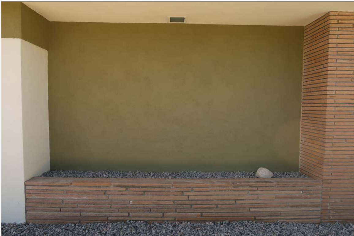
Image 18: North elevation with flat-stacked Arizona sandstone planter, view south (Chattel, 2024)
