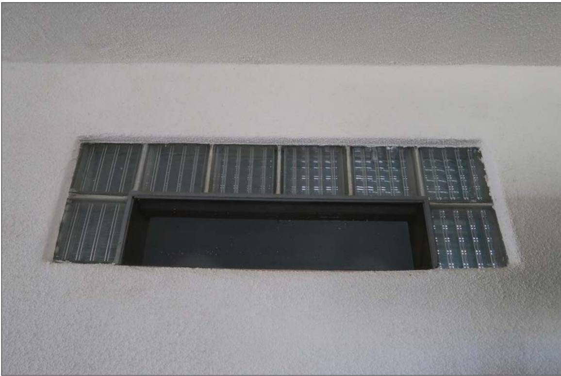
Image 56: Detail of glass block with vent installed, view west (Chattel, 2024)
