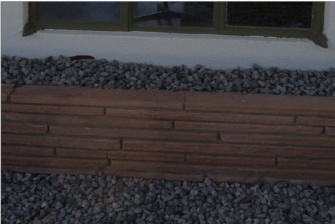
Image 14: Detail of flat-stacked Arizona sandstone planter at north elevation, view south (Chattel, 2024)
