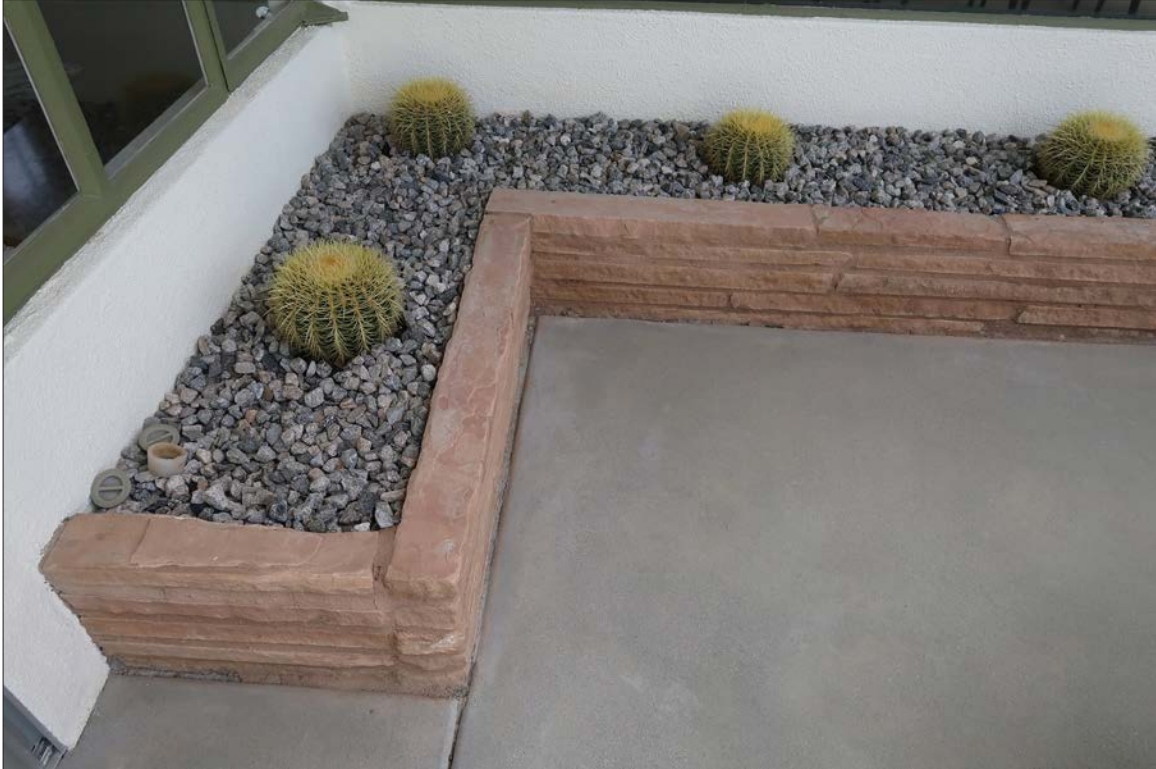
Image 43: Detail of planter at corner of south and west elevations, view east, note different application of mortar compared to north elevation planters (Chattel, 2024)
