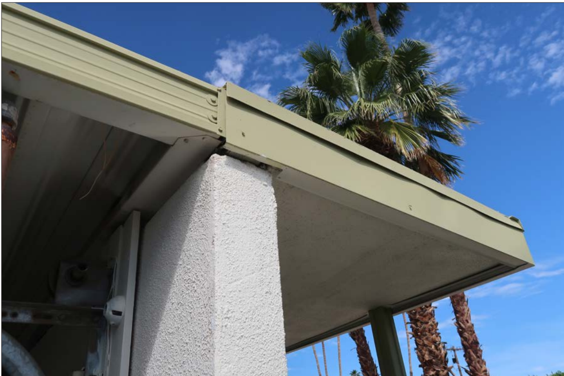
Image 60: Detail of added stucco-clad wall surround and stucco-clad eave at carport/garage (Chattel, 2024)
