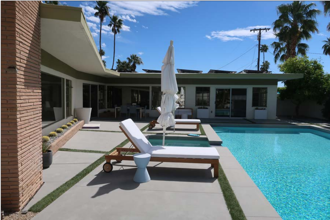
Image 35: West elevation facing pool, view east (Chattel, 2024)
