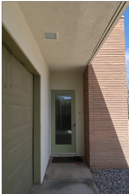
Image 22: Side door by carport/garage, view west (Chattel, 2024)
