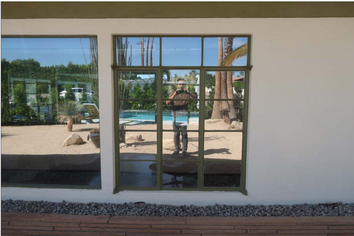
Image 12: Detail of casement windows with transom at north elevation, view south (Chattel, 2024)
