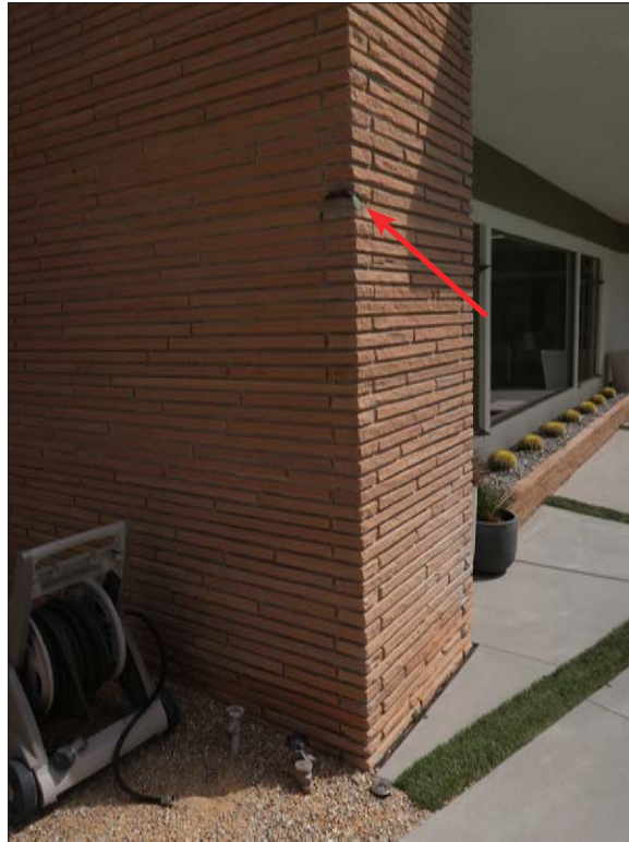
Image 29: Evidence of former gate attachment to flat-stacked Arizona sandstone chimney identified with red arrow, view northeast (Chattel, 2024)
