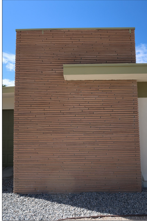
Image 19: Rectangular flat-stacked Arizona sandstone chimney at north elevation, view south (Chattel, 2024)
