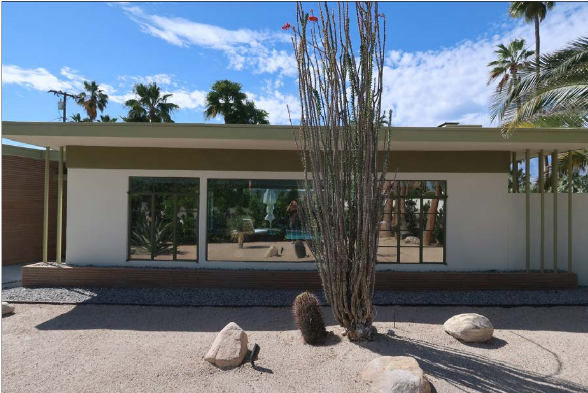
Image 9: North elevation of west volume, view south (Chattel, 2024)
