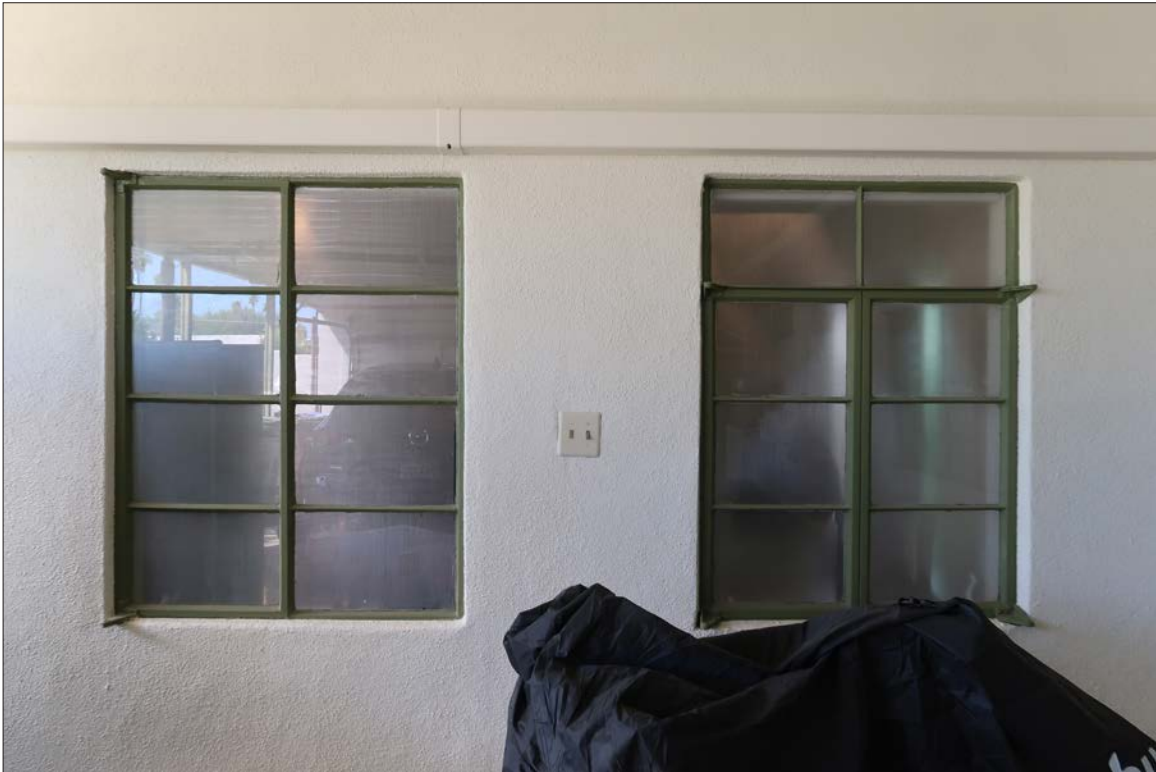
Image 53: Windows at north elevation of former maid's quarters, view north (Chattel, 2024)
