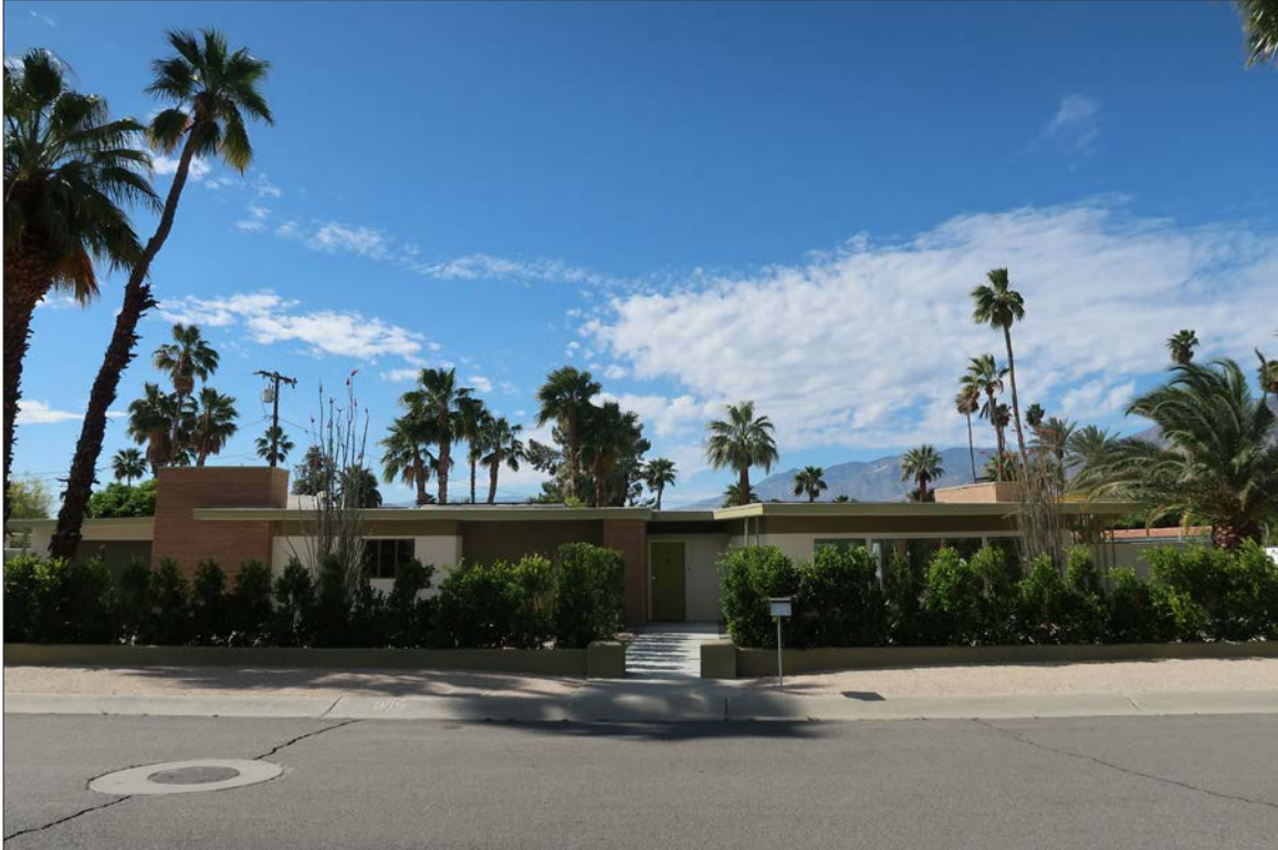
Image 3: Primary north elevation, view south (Chattel, 2024)
