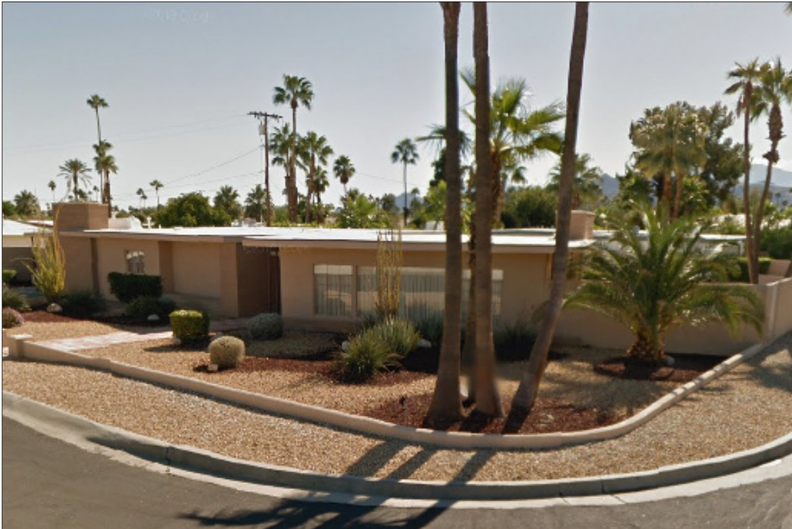
Image 5: North elevation of subject property prior to landscape alterations (Google Street View, 2011)
