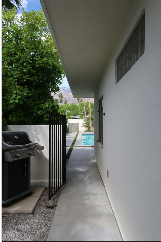
Image 45: South elevation path to carport/garage, view west (Chattel, 2024)
