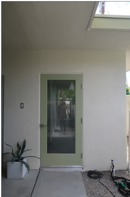
Image 46: Door to former maid's quarters behind carport/garage, view east (Chattel, 2024)
