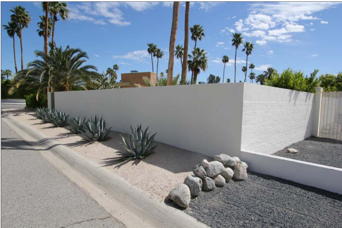
Image 26: Privacy wall at southwest corner of subject property, view northeast (Chattel, 2024)
