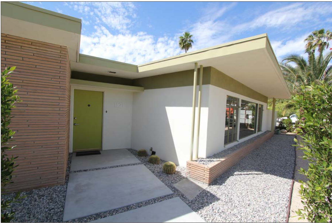
Image 8: Inset entryway and west volume at north elevation, view southwest (Chattel, 2024)
