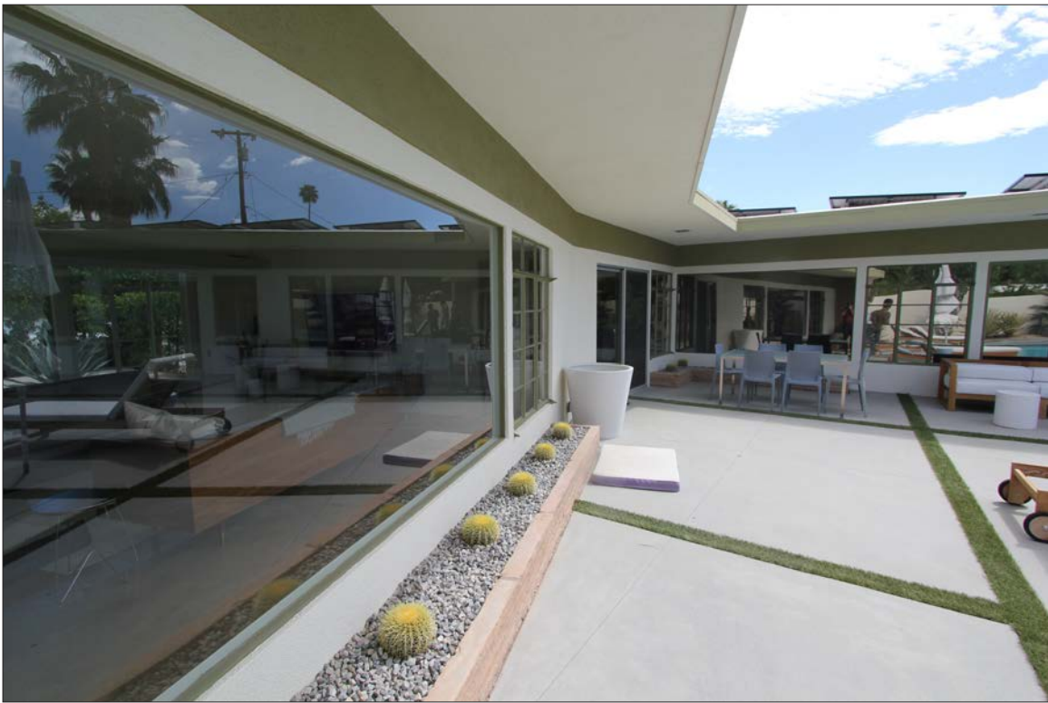
Image 38: South (left) and west (right) elevations, view east (Chattel, 2024)
