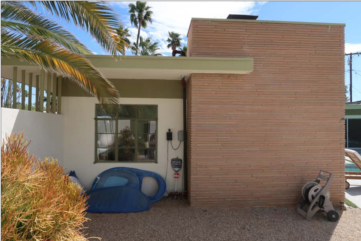
Image 27: West elevation, view east (Chattel, 2024)
