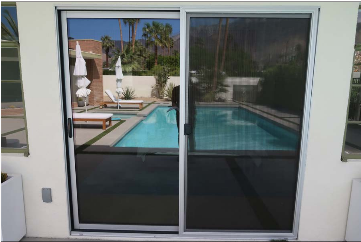
Image 42: Contemporary sliding door, view east (Chattel, 2024)
