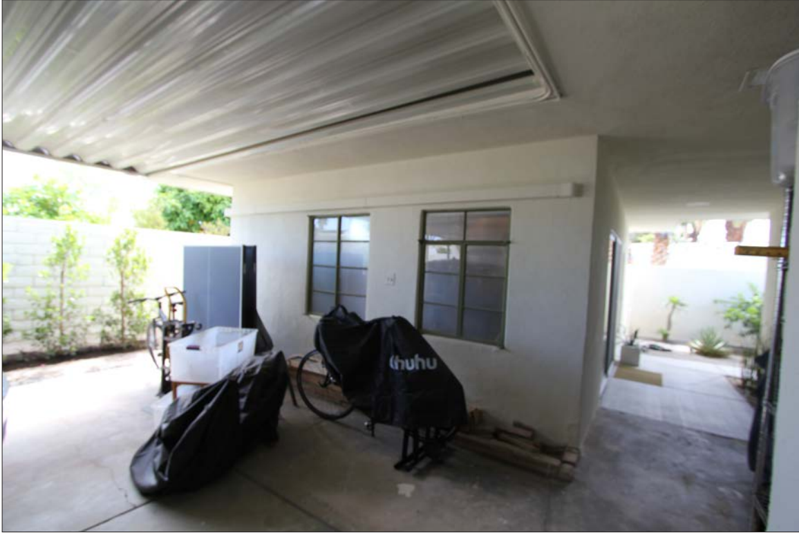
Image 49: North elevation of former maid's quarters, view southeast (Chattel, 2024)
