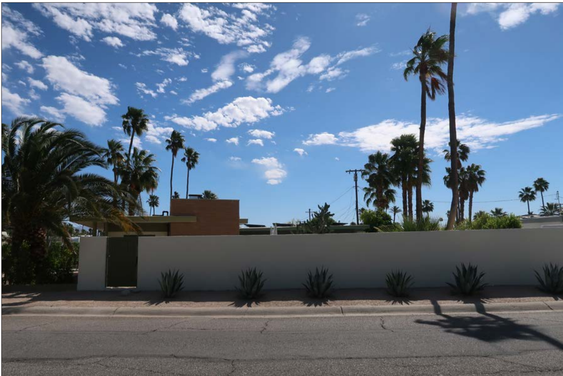
Image 4: West elevation, view east (Chattel, 2024)
