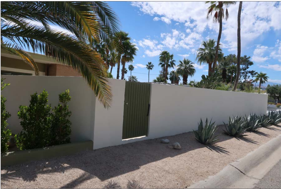
Image 24: Added privacy wall at west of subject property, view southeast (Chattel, 2024)
