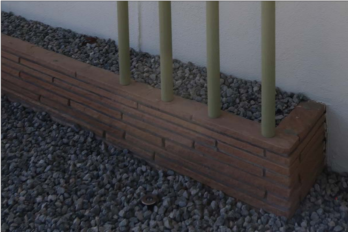
Image 13: Detail of flat-stacked Arizona sandstone planter at north elevation, view southeast (Chattel, 2024)
