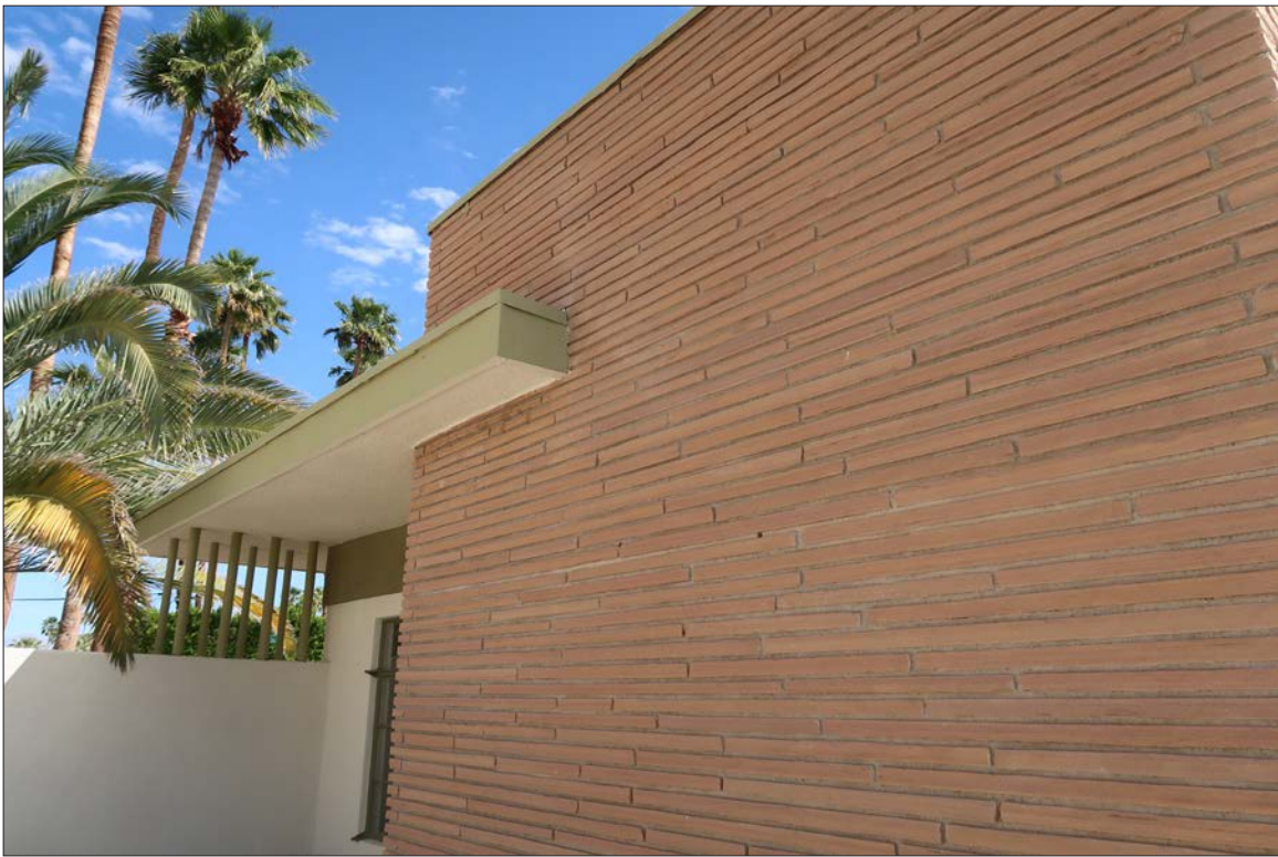
Image 28: Detail of eave continuing over flat-stacked Arizona sandstone chimney at west elevation, view northeast (Chattel, 2024)
