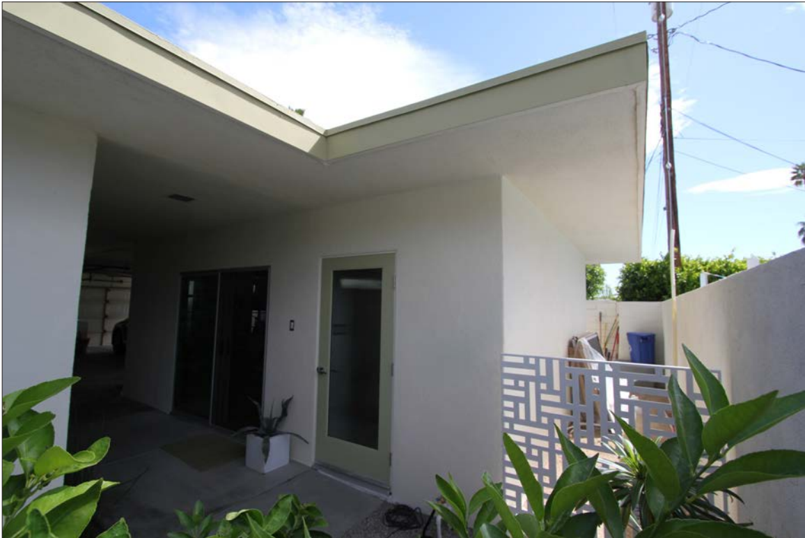
Image 47: West elevation of former maid's quarters, view northeast (Chattel, 2024)
