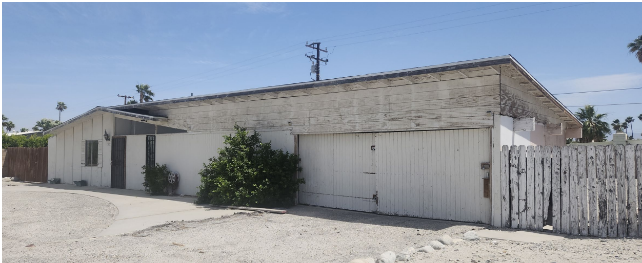
STREET VIEW OF THE EXISTING RESIDENCE, MAY 2024.
