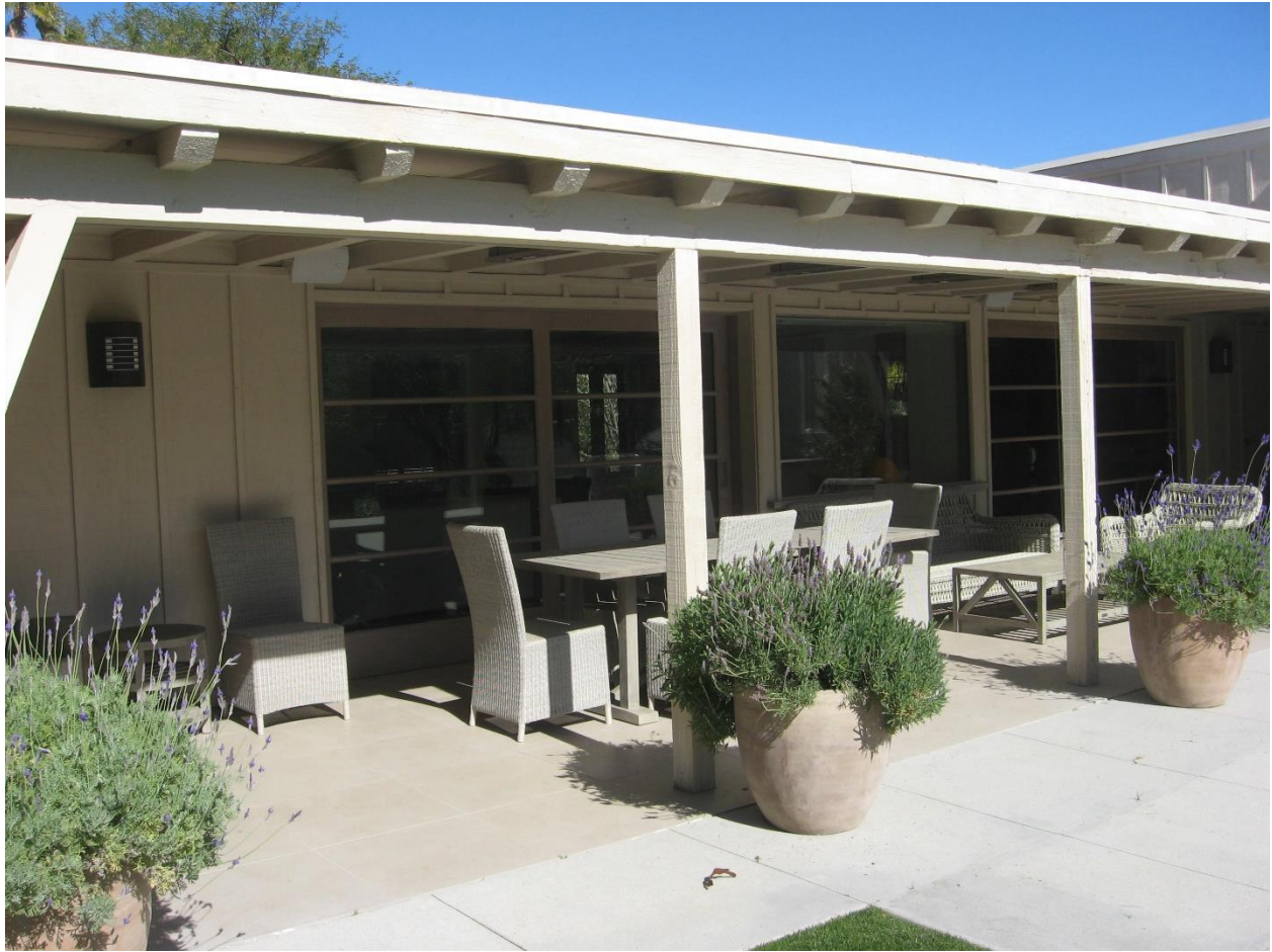
Rear porch showing oversized sliding door on left with new twin on right. Picture window in center is also a recent addition. (Author photo. February 2023)
