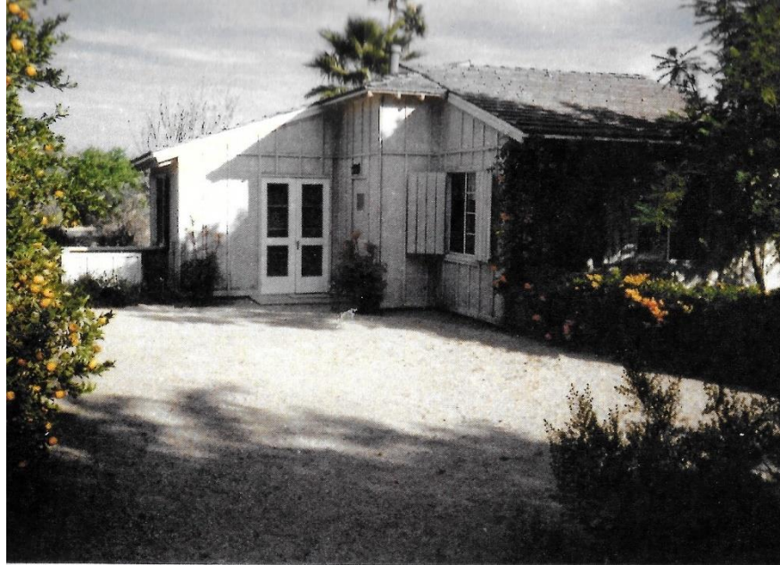
The future site of the 2016 master bedroom addition. (Courtesy Chuck Bentall)
