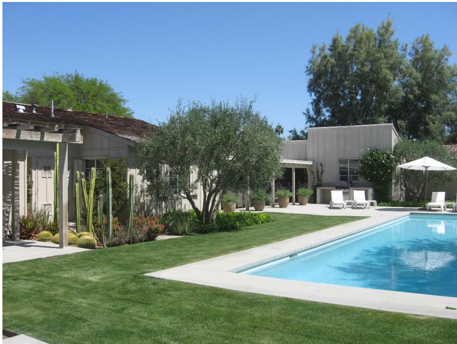
View of south façade with new master bedroom on left.
