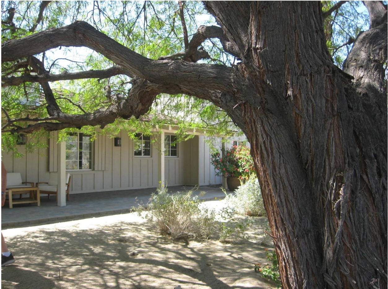
A portion of the north elevation of the Burnham-Wells Residence in 2023. Windows are recent replacements set within original openings. (Author photo. February 2023)
