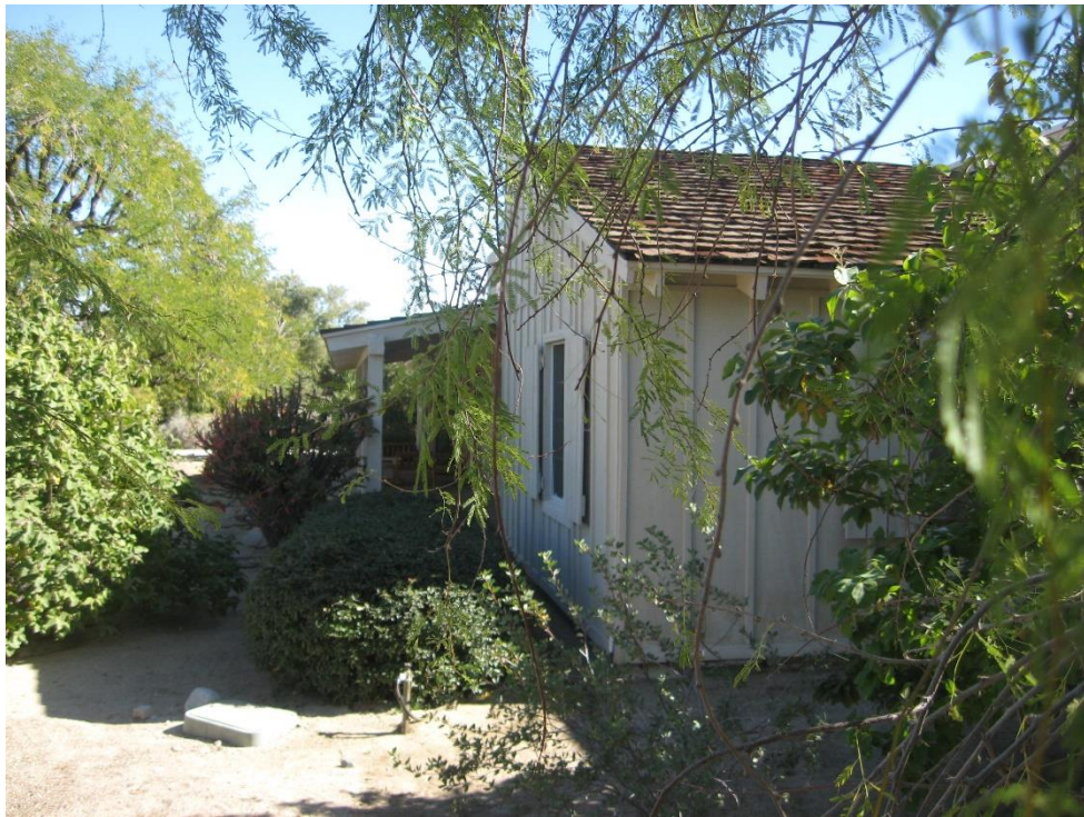
Looking eastwards towards front entrance. (Author Photo. February 2023)
