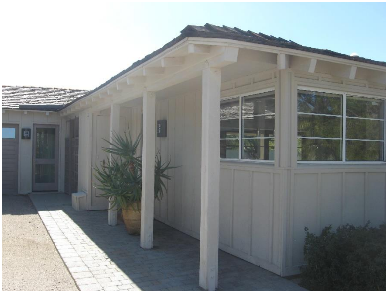
View of Albert Frey's kitchen porch addition (Author Photo. February 2023)
