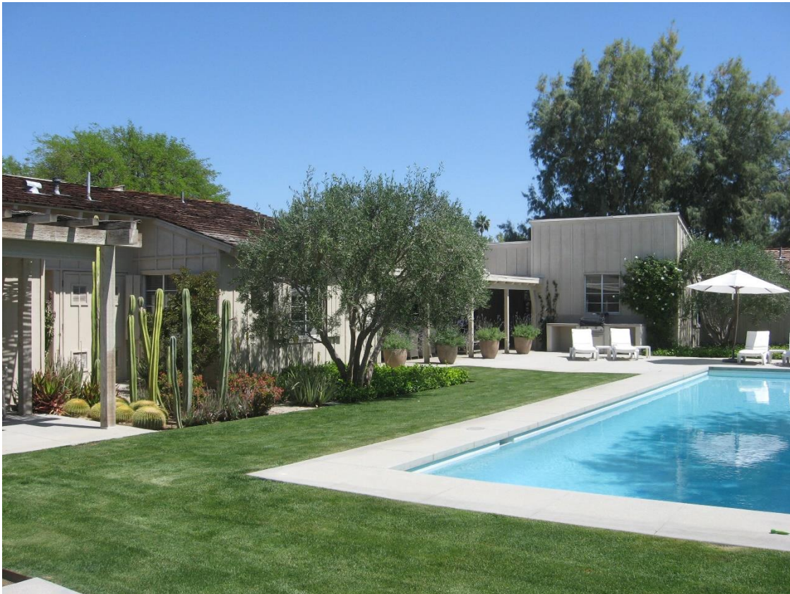
View looking east towards rear façade. Note the shed roof, deep porch. Pool is of recent (2016) vintage. (Author photo. February 2023)
