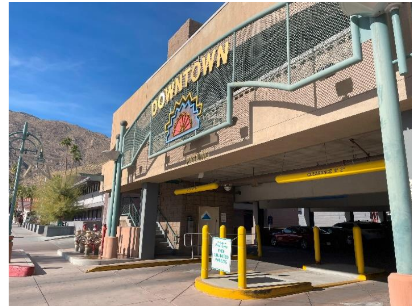
Downtown Parking Garage, South Palm Springs.
