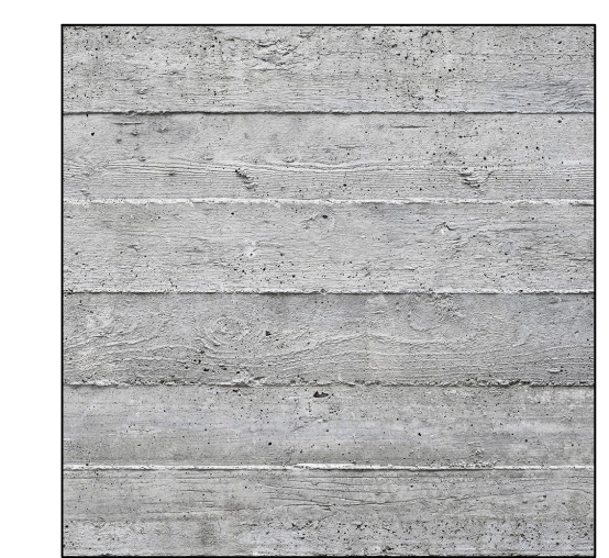
CW-1 Exposed Concrete Wall; Concrete Stone Veneer
